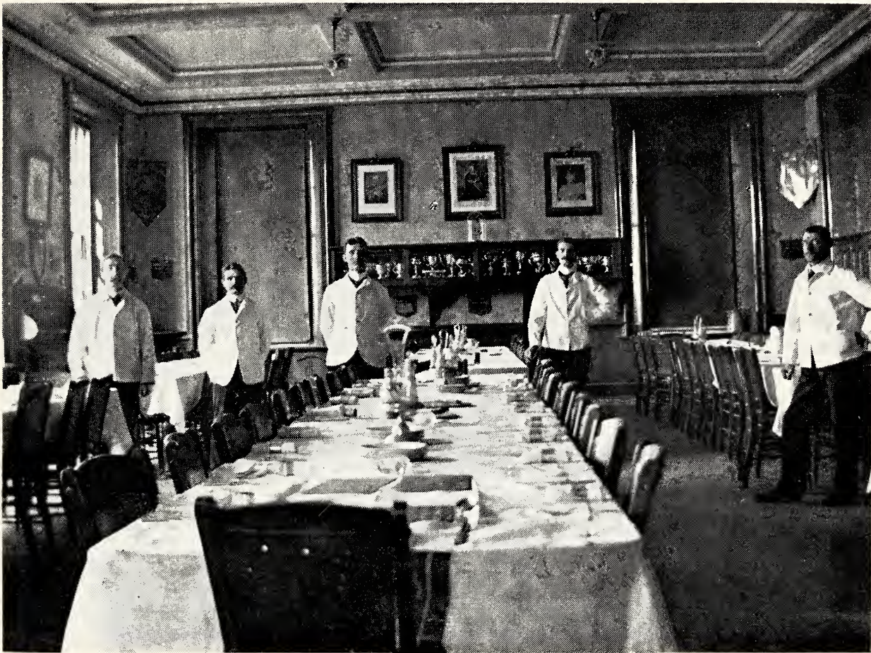
MESS HALL, "NORTH" (MacKENZIE) BUILDING (Courtesy of No. 761, James W. Ross)
