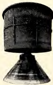
Blast Furnace Bell and Hopper for a Canadian Steel Mill
