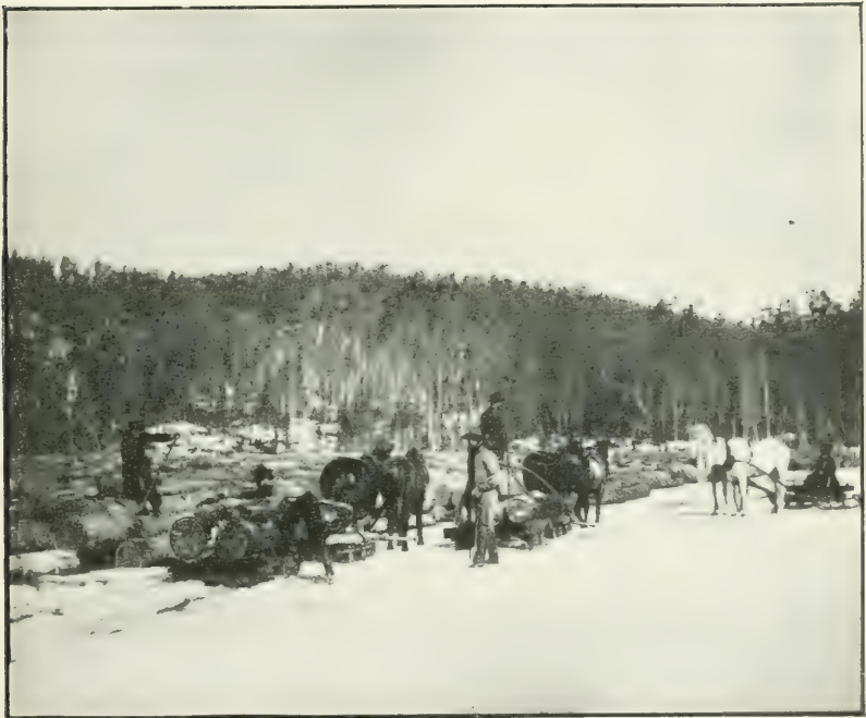
PILING LOGS ON THE FROZEN RIVER.
