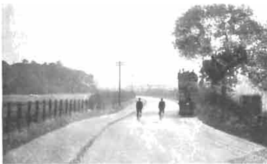
LIGHT RAILWAY CONSTRUCTION ON THE ROAD TO STOURPORT
