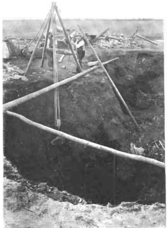
HOISTING A BLOCK OF DENNER HILL STONE
