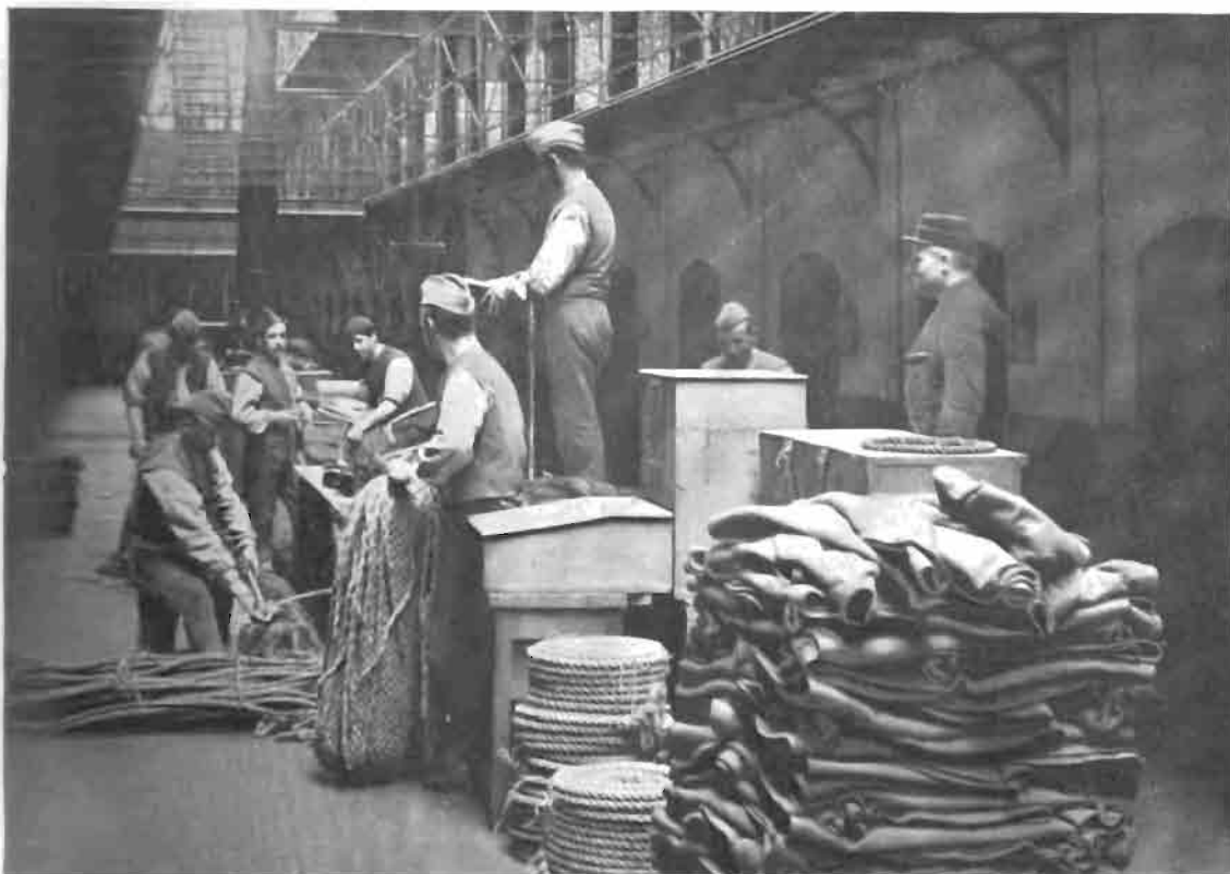
MAKING SHIPS' FENDERS FOR THE ADMIRALTY
