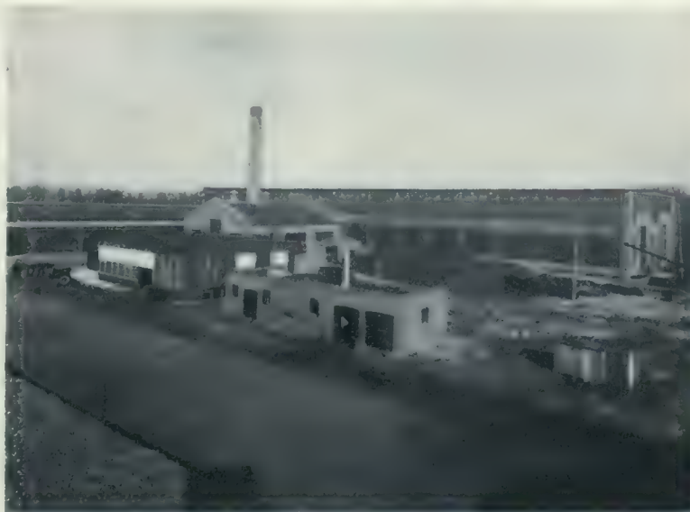
BOILER HOUSE, TRANSFORMER ROOM AND STORAGE.
