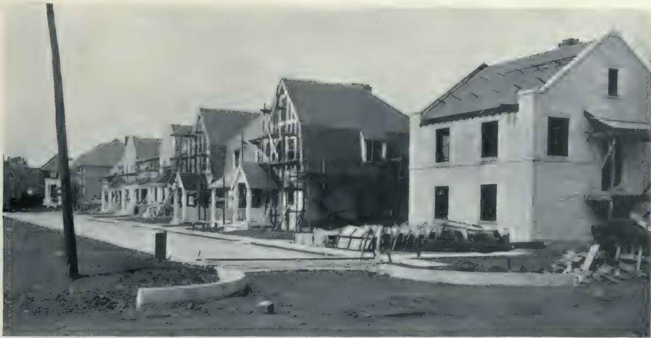
PROGRESS VIEW, RE-HOUSING DEVELOPMENT, HALIFAX, N. S.
