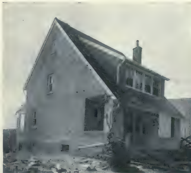
HYDRO-STONE CONSTRUCTION, RE-HOUSING DEVELOPMENT, HALIFAX, N. S.
