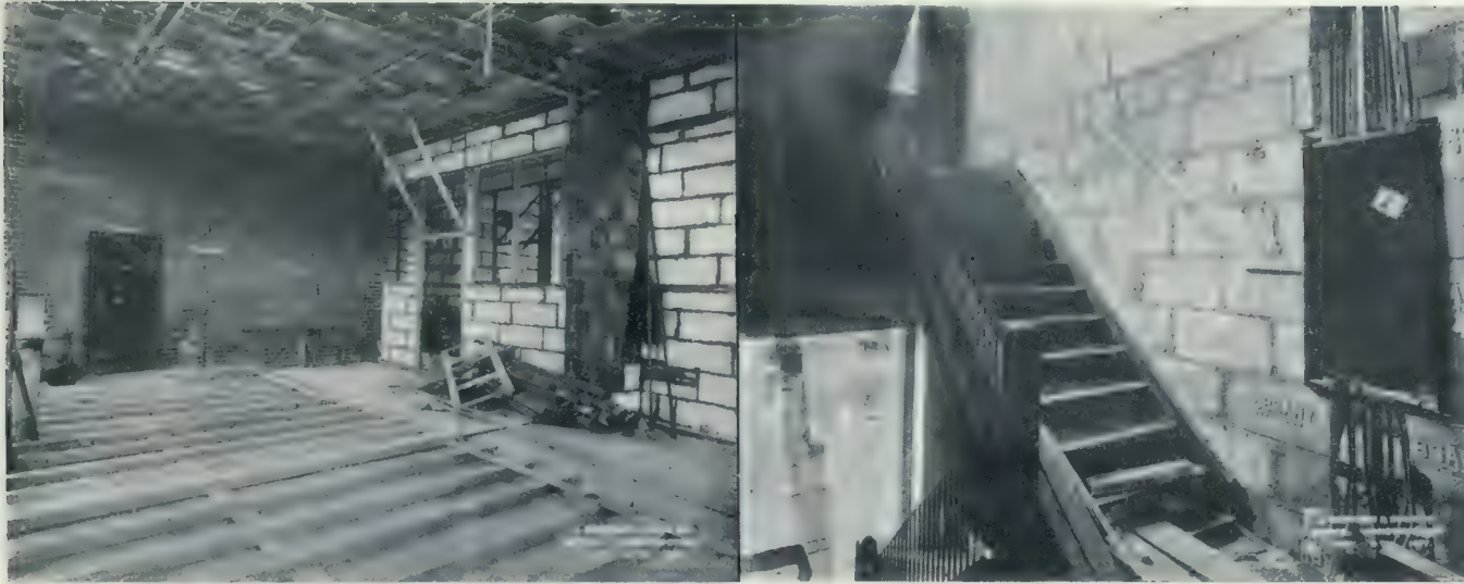
PROGRESS VIEW SHOWING GYPSUM BLOCK PARTITIONS AND HOLLOW TILE FLOORS WITH CINDER FILL AND NAILING STRIPS FOR HARDWOOD FINISH. OFFICE BUILDING OF JOHN BERTRAM & SONS COMPANY, DUNDAS, ONT.
