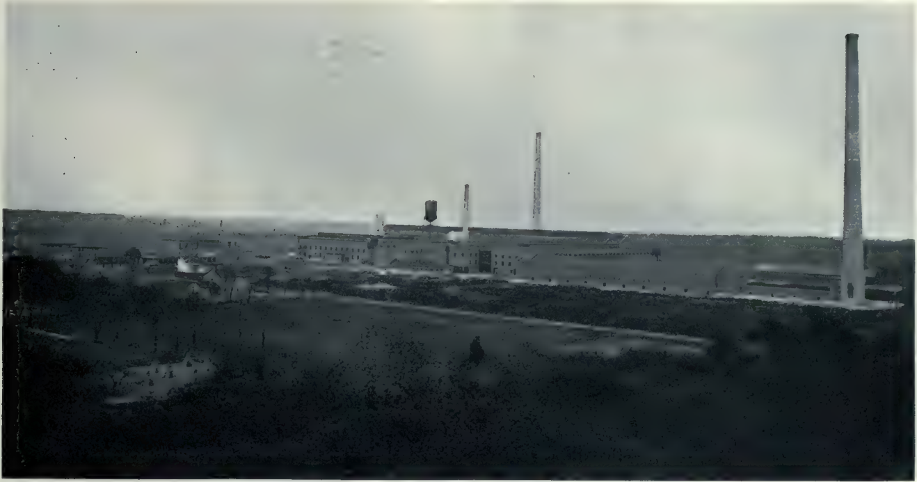
INTERNATIONAL NICKEL COMPANY'S PLANT FROM SOUTHWEST VIEWPOINT.
