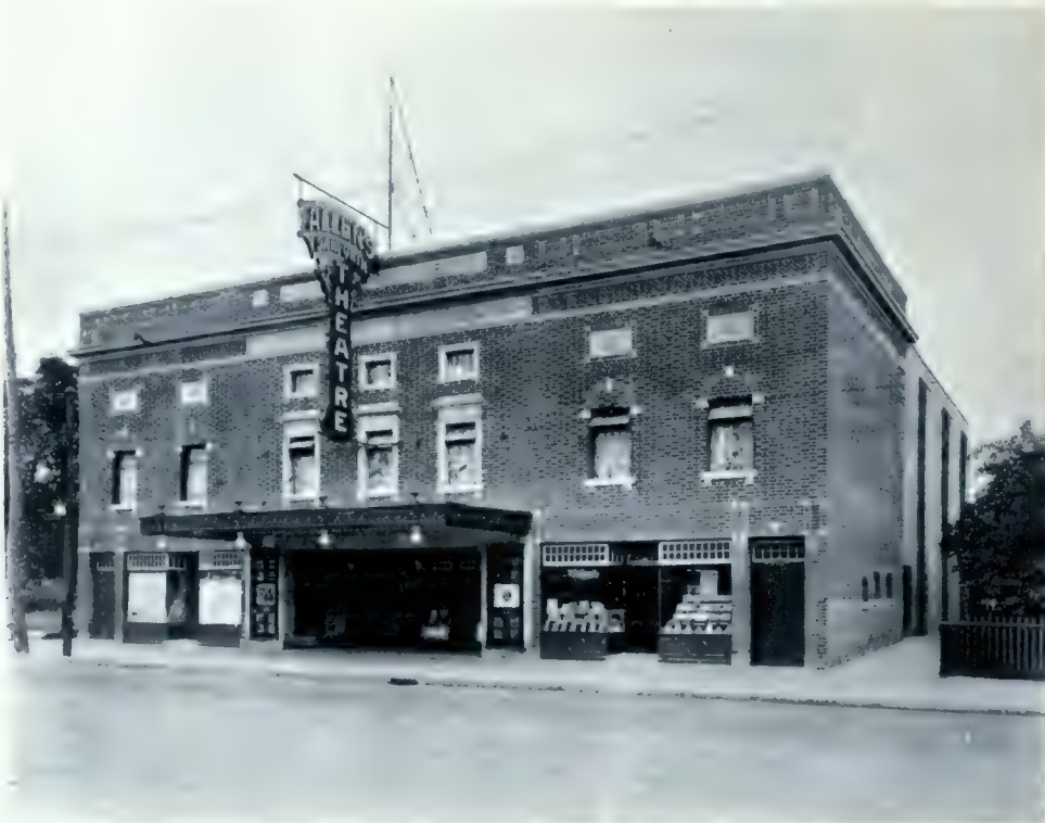
GENERAL VIEW, ALLEN'S DANFORTH THEATRE, TORONTO.
