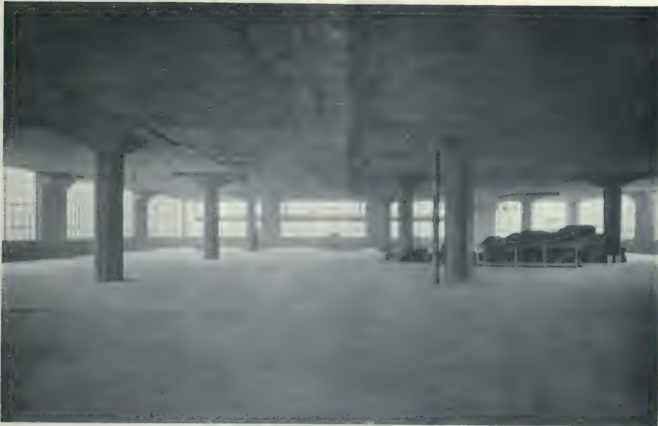
INTERIOR VIEW OF WAREHOUSE, SHOWING 30 FT. SPANS.
