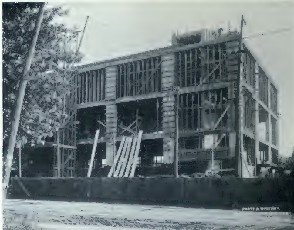
FORM WORK, PRATT & WHITNEY COMPANY'S BUILDING, DURING PROCESS OF CONSTRUCTION.
