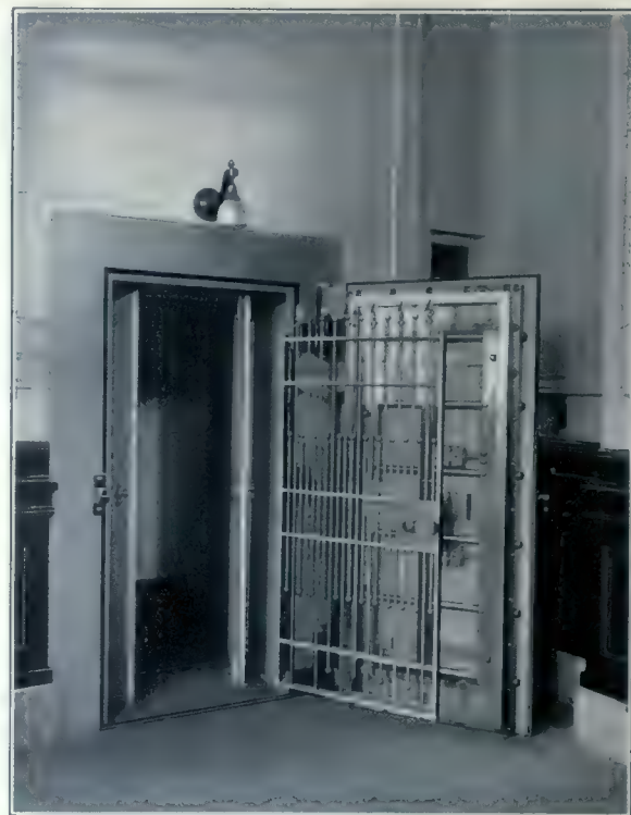
One of Two Similar Vaults Installed by the Goldie & McCulloch Co. in the Merchants Bank, Galt, Ont.
