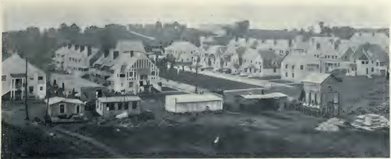
COMPLETED COURT DEVELOPMENT, RE-HOUSING SCHEME, HALIFAX, N.S.
