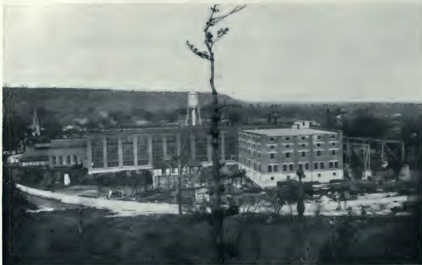
GENERAL VIEW FROM THE SOUTH-WEST.
