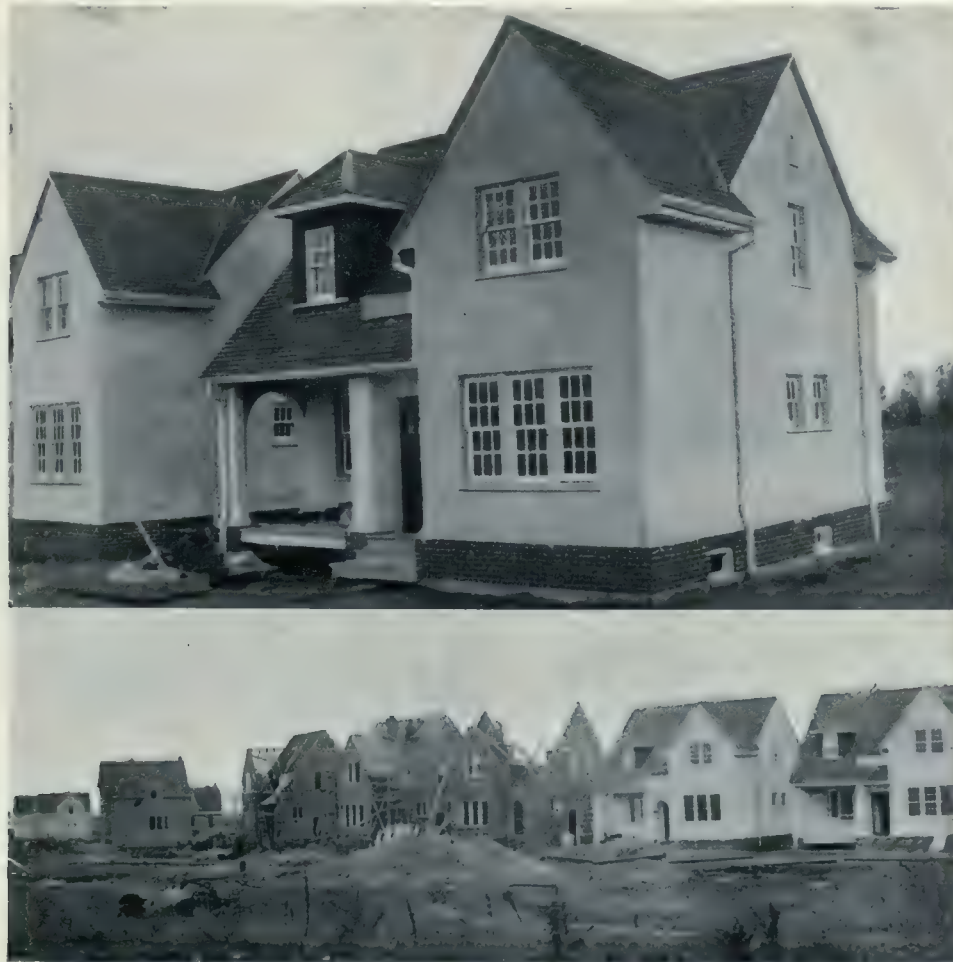
LANDSDOWNE PARK ESTATE, BRANTFORD, ONT., SHOWING TYPE OF HOUSES BEING ERECTED FOR THE DOMINION STEEL PRODUCTS COMPANY. SCOTT & WARDELL, ARCHITECTS.
