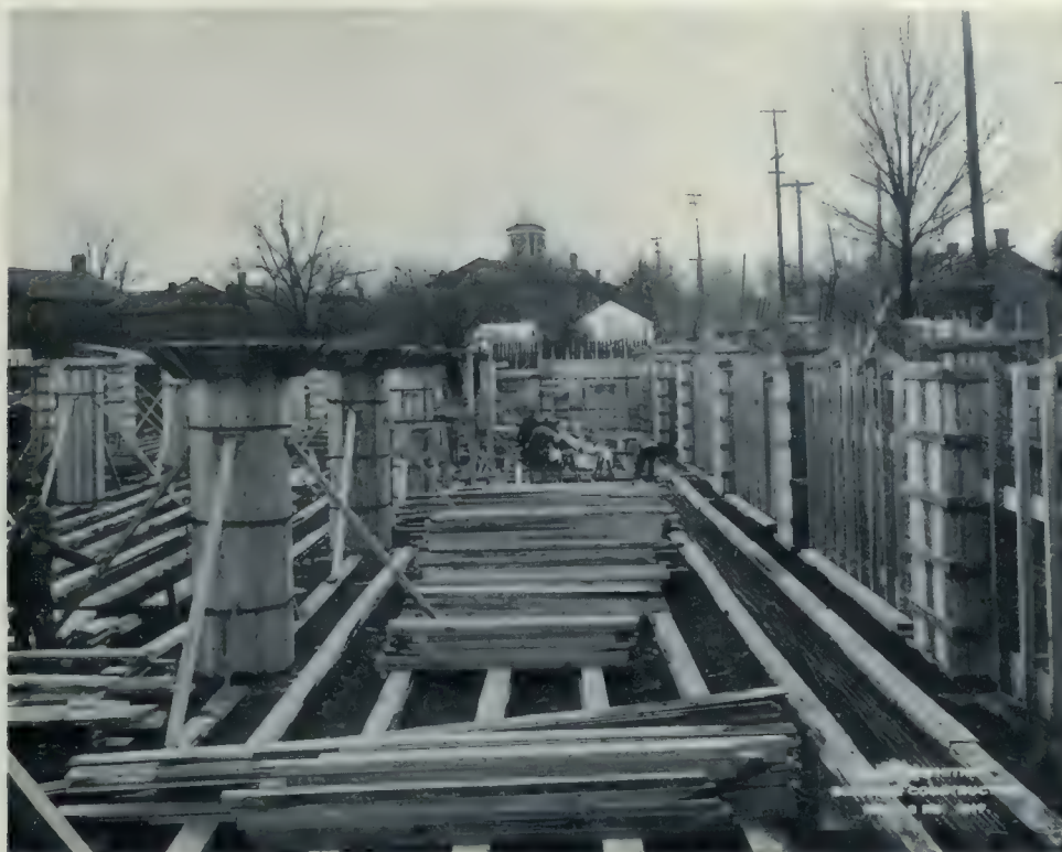
VIEW SHOWING FORM WORK OF BASEMENT, PRATT &amp; WHITNEY BUILDING, DUNDAS, ONT.
