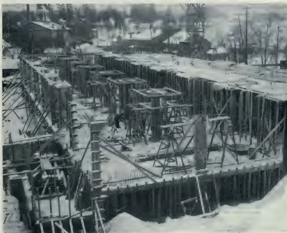
LOWER FLOOR COLUMNS, PRATT &amp; WHITNEY COMPANY'S BUILDING, SHOWING FORMS FOR CAPS.
