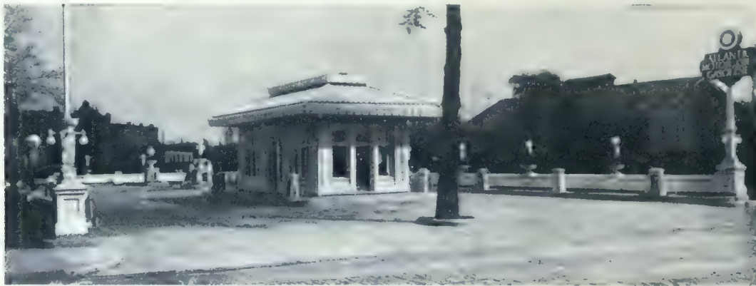
SERVICE STATION AT EAST LIBERTY, PITTSBURG, PA.
