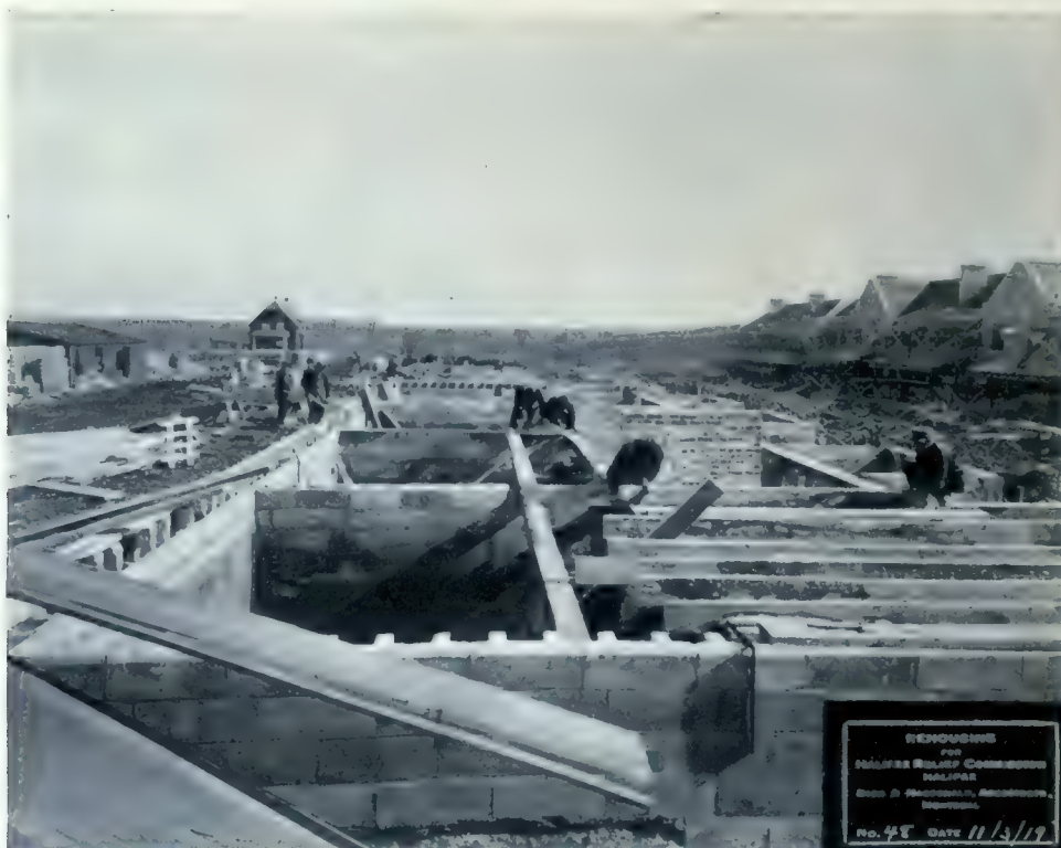
VIEW SHOWING WALL CONSTRUCTION OF HYDRO-STONE HOUSES.
