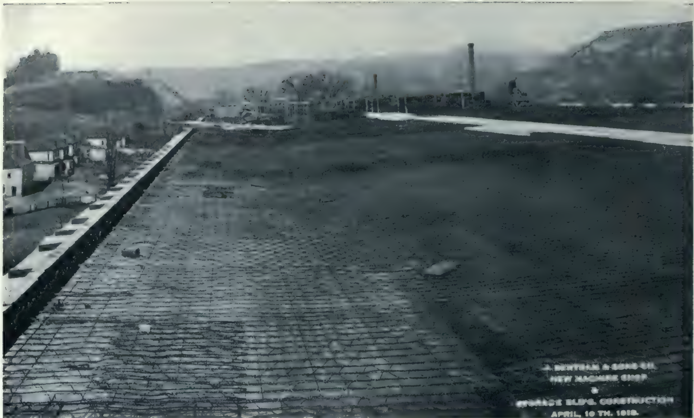
ROOF OF PERMANENT STORAGE BUILDING.
