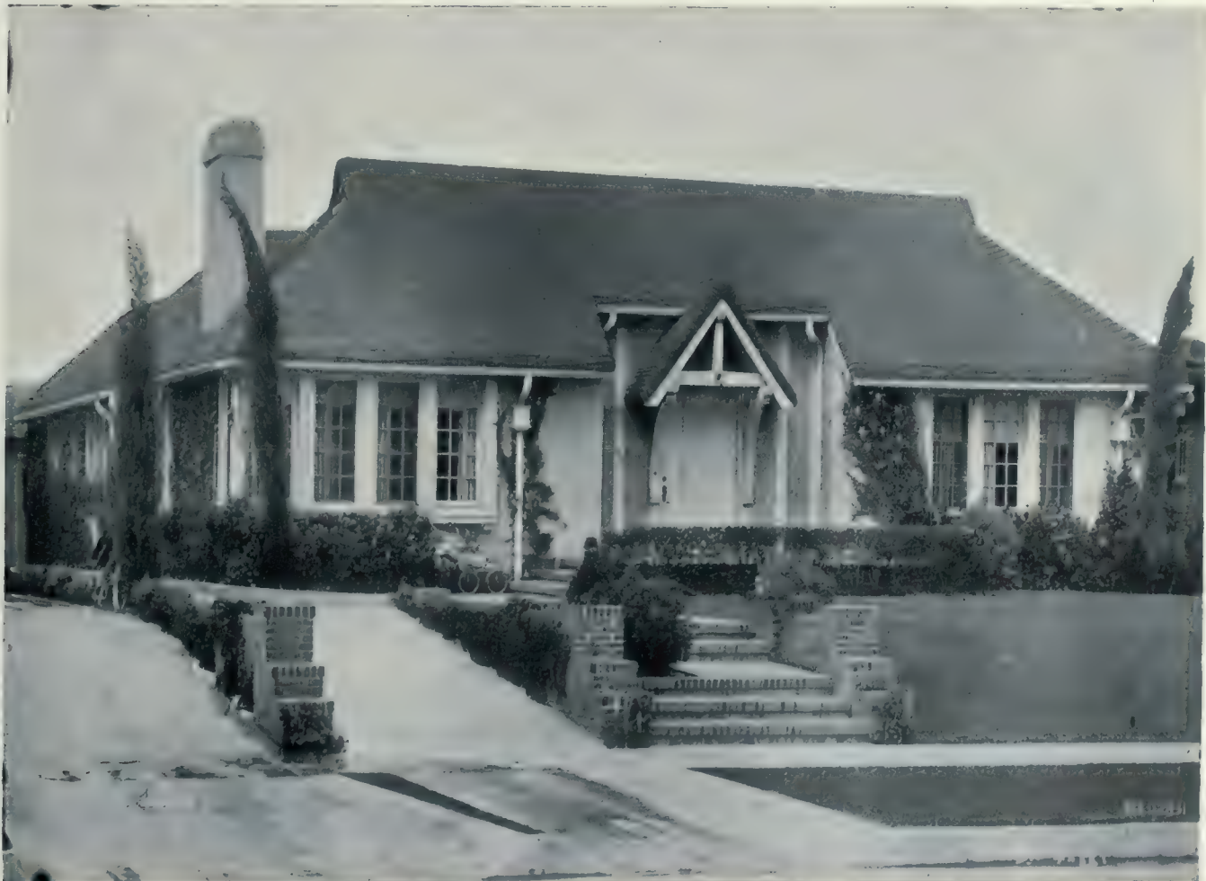
THE THATCHED SHINGLE ROOF, A SOMEWHAT RECENT INNOVATION, AS SEEN IN A SMALL CALIFORNIA HOME.
