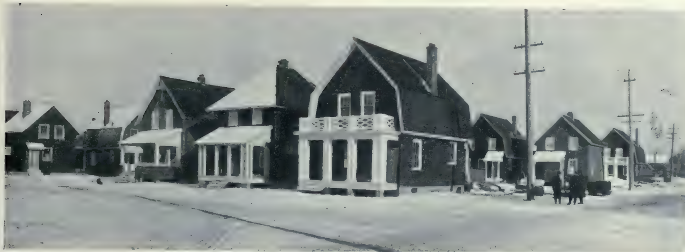
FRAME DWELLINGS, RE-HOUSING DEVELOPMENT, HALIFAX, N. S.
