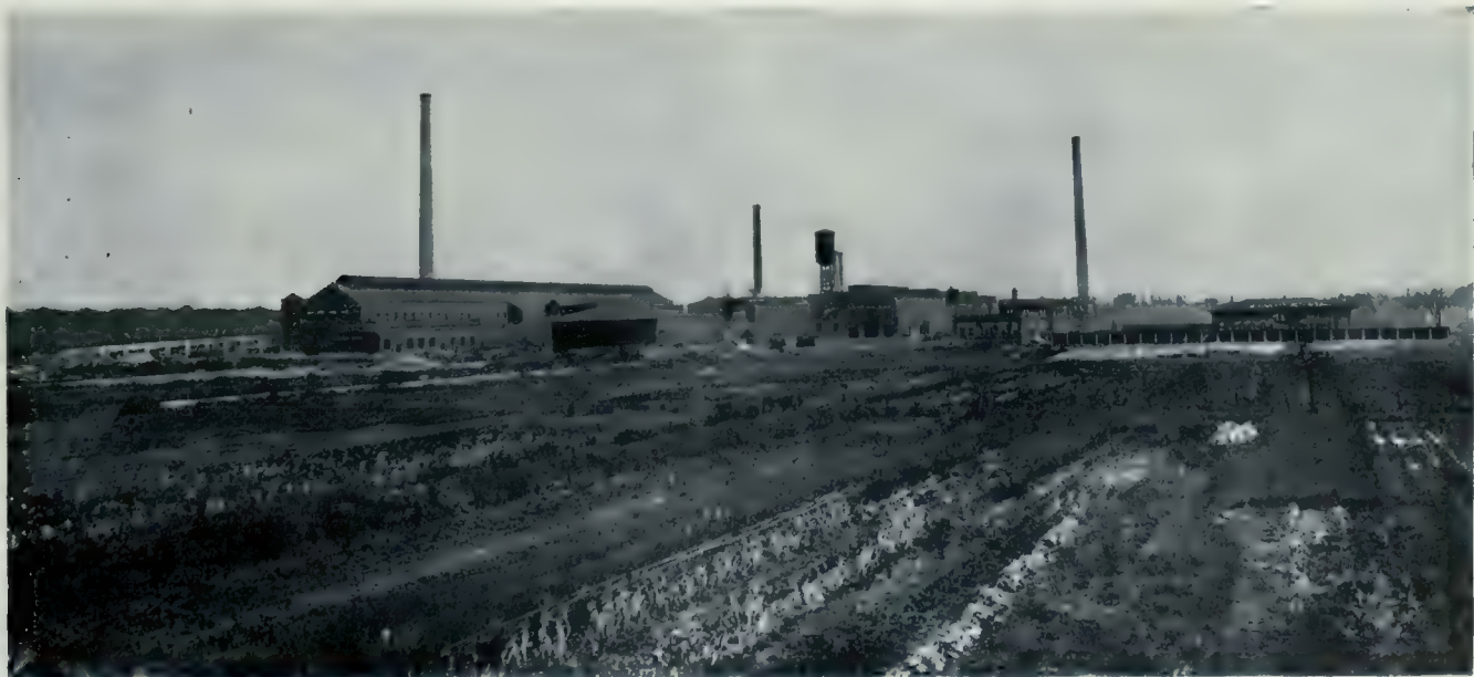
VIEW OF PLANT FROM NORTHEAST POSITION.
