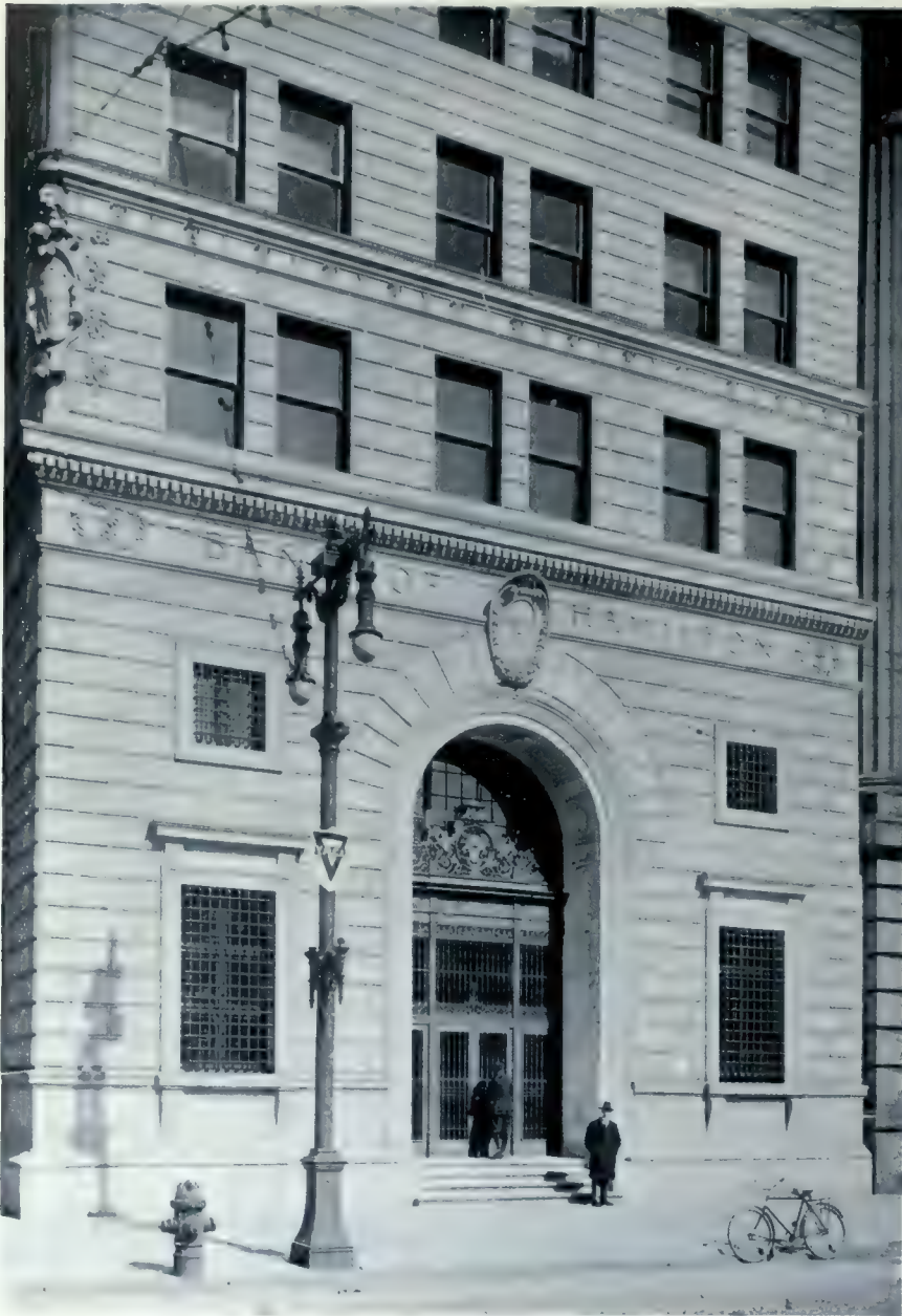
DETAIL OF LOWER FACADE: BANK OF HAMILTON BUILDING, WINNIPEG.
