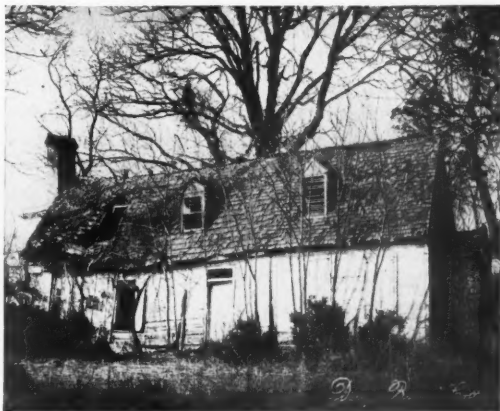
THE OLD DAVID BURNS COTTAGE. One of the original houses on the site of Washington.
