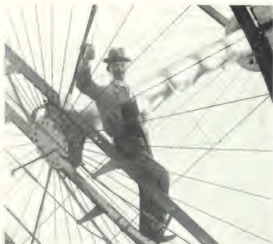
THE SOLAR BOILER
