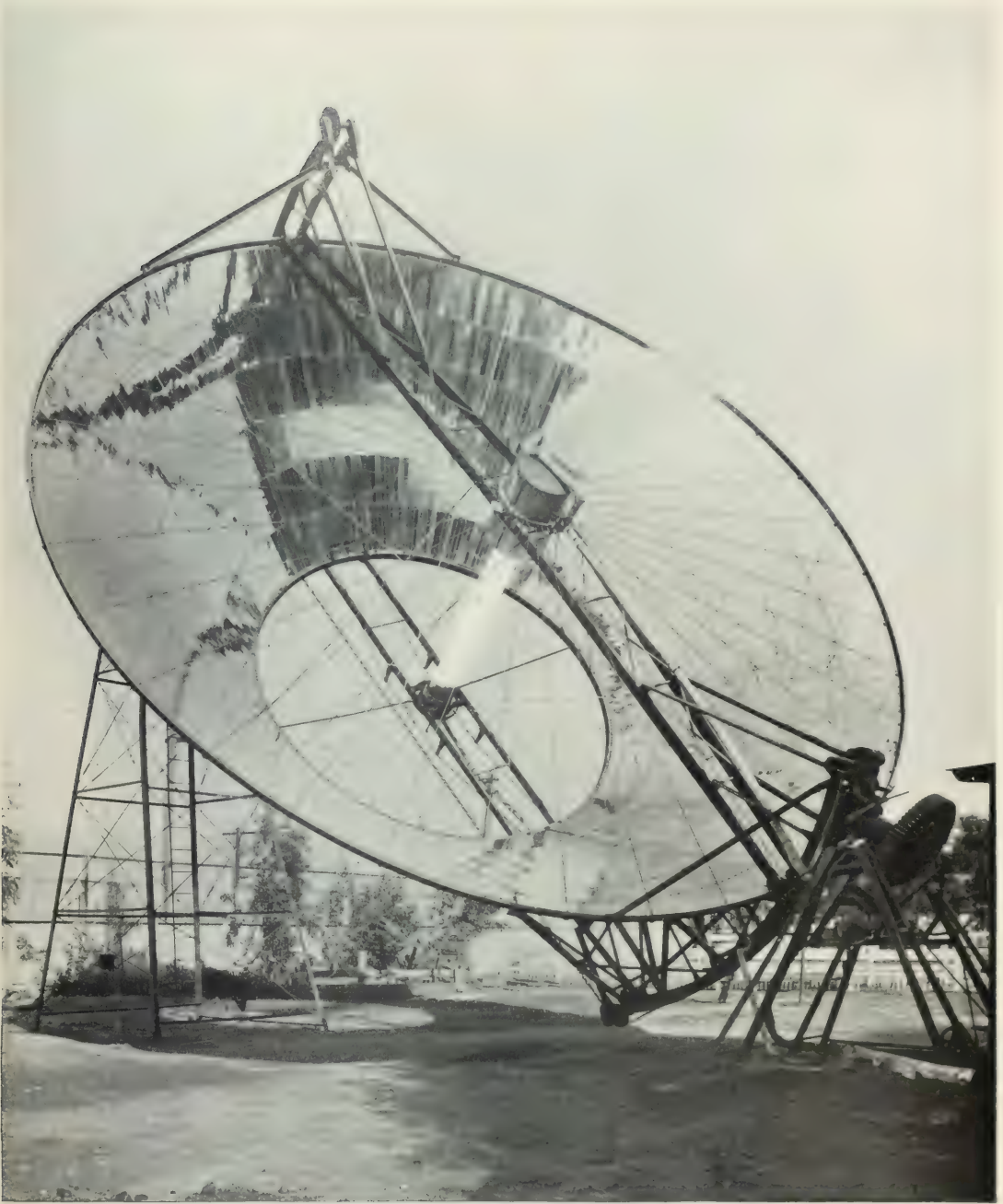
BLOWING OFF STEAM WITH A PRESSURE OF 210 LBS.
