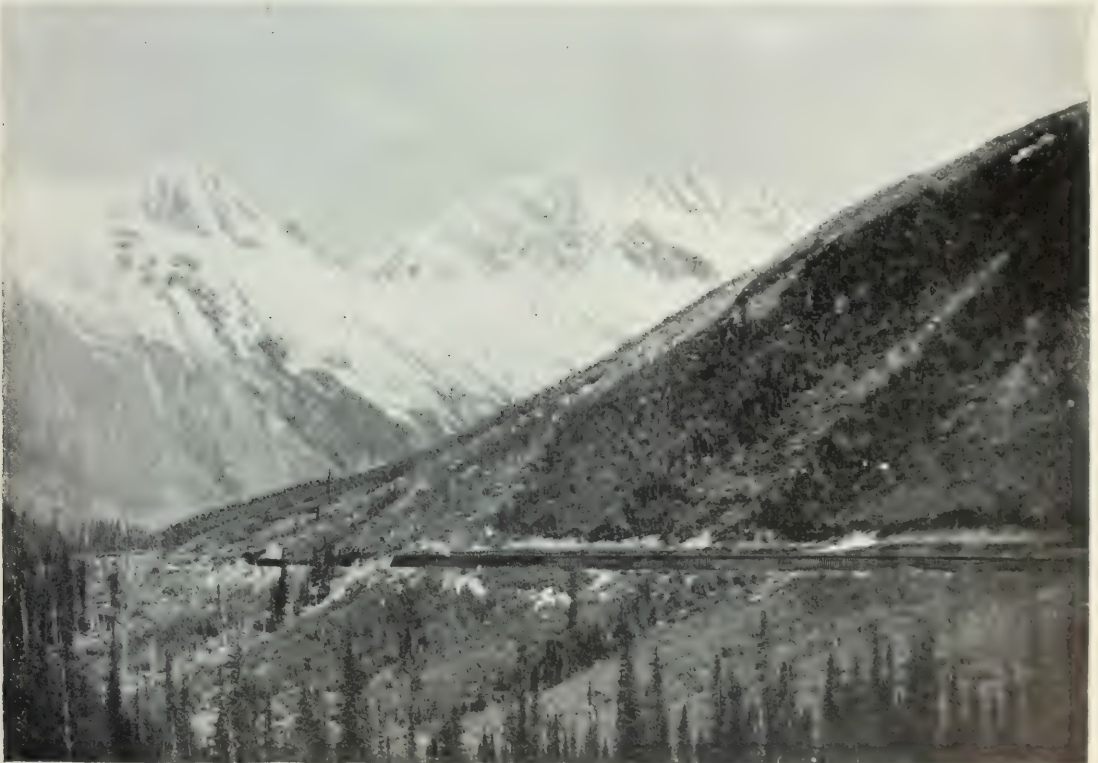
THE SNOW SHEDS FROM THE OUTSIDE.
