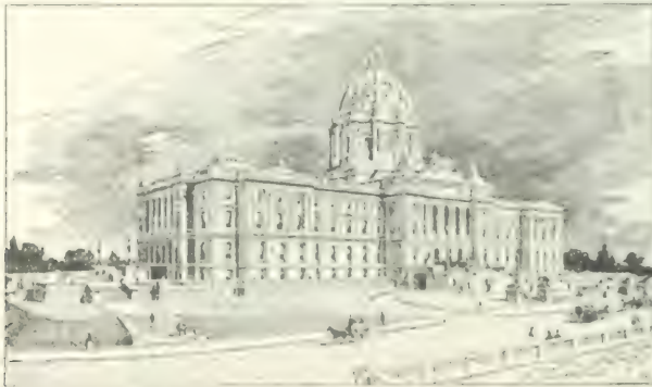
THE NEW CAPITOL OF MINNESOTA AT ST. PAUL.
