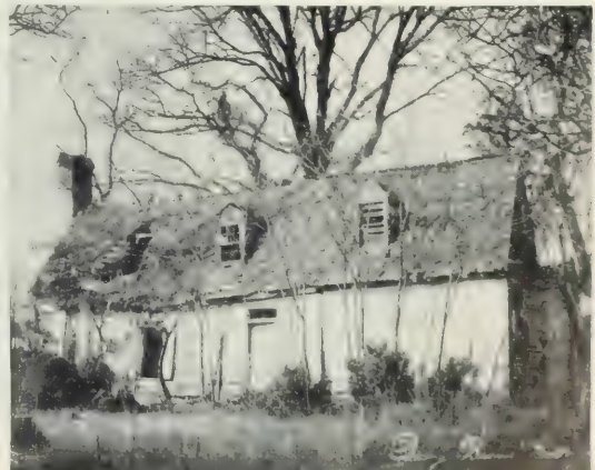
THE OLD DAVID BURNS COTTAGE One of the original houses on the site of Washington.
