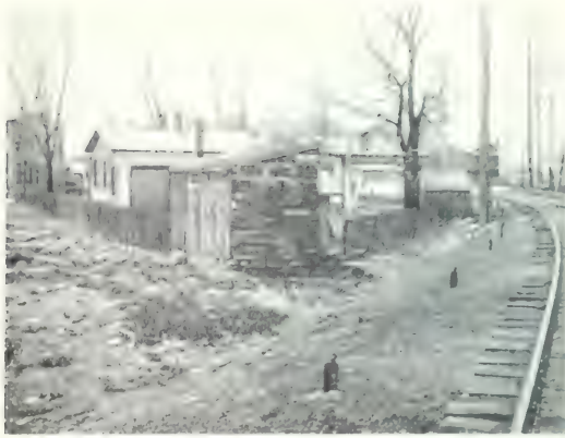
A FORMER VIEW ALONG A RAILROAD LEADING INTO DAYTON, OHIO
