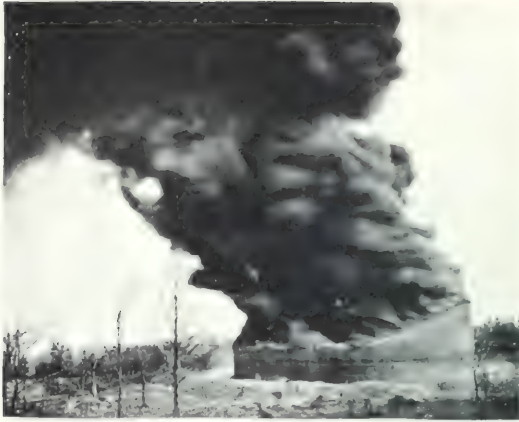
A BURNING OIL TANK.
