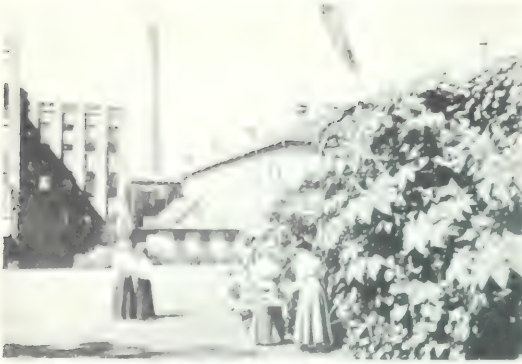
A GARDEN WITH TERRACE FOR EMPLOYEES AT "WESTINGHOUSE" CO. (CITY OF PITTSBURGH)
