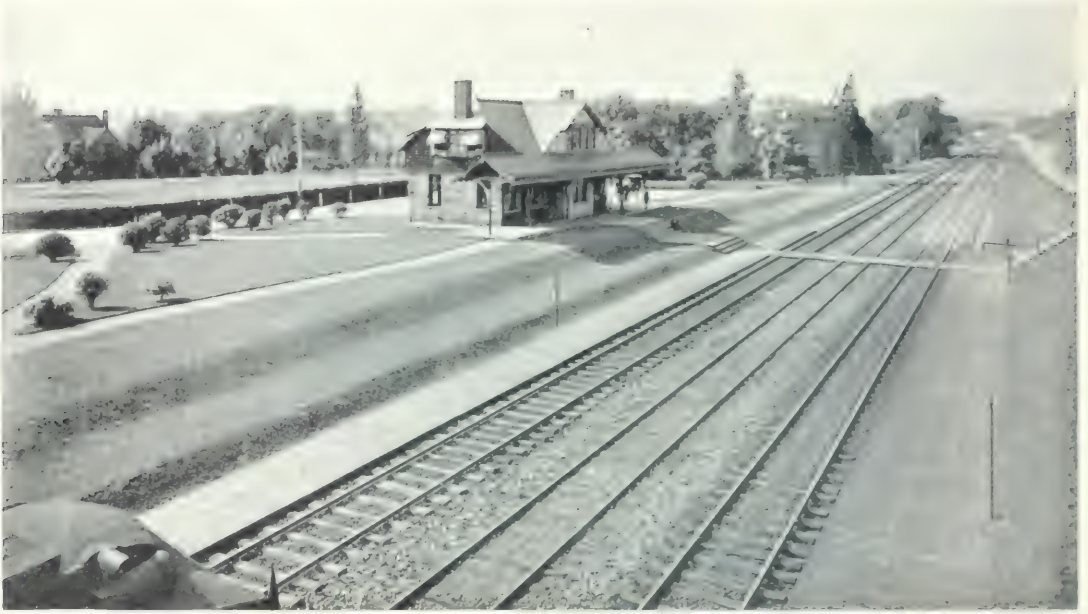
RUXTON STATION, NEAR BALTIMORE.
