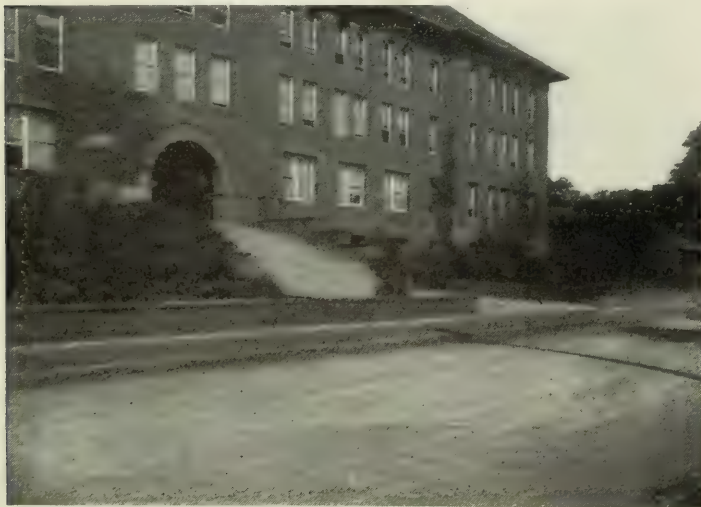
A MAIN ENTRANCE TO THE BROOKLINE, MASSACHUSETTS, HIGH SCHOOL
