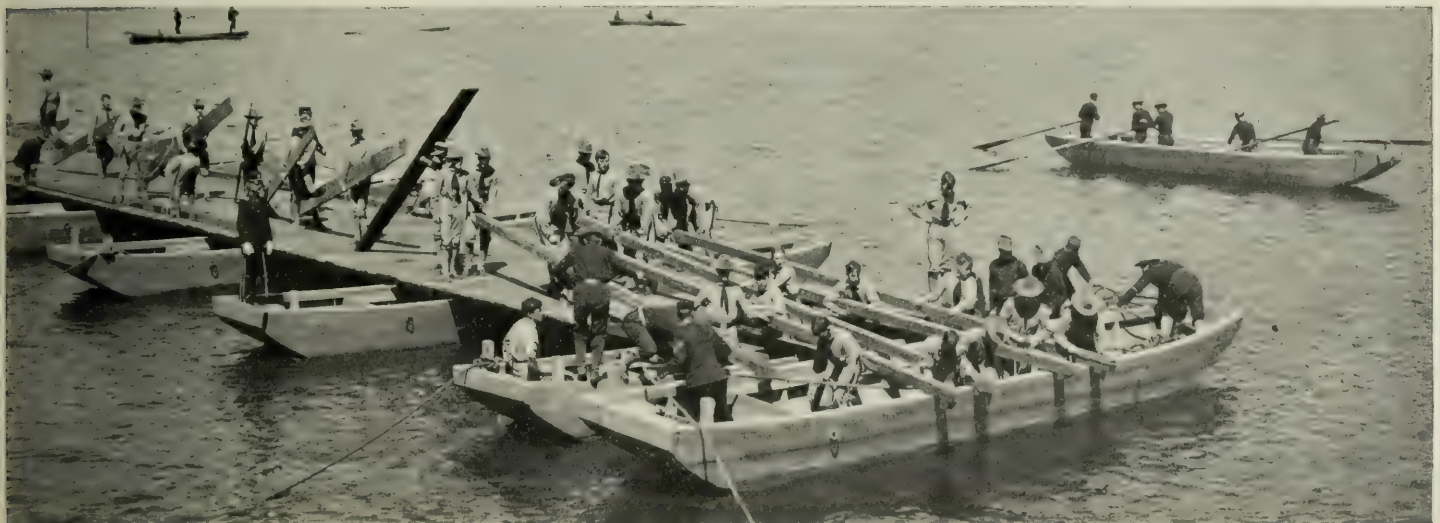
PONTOON BRIDGE BUILDING Laying lengthwise timbers
