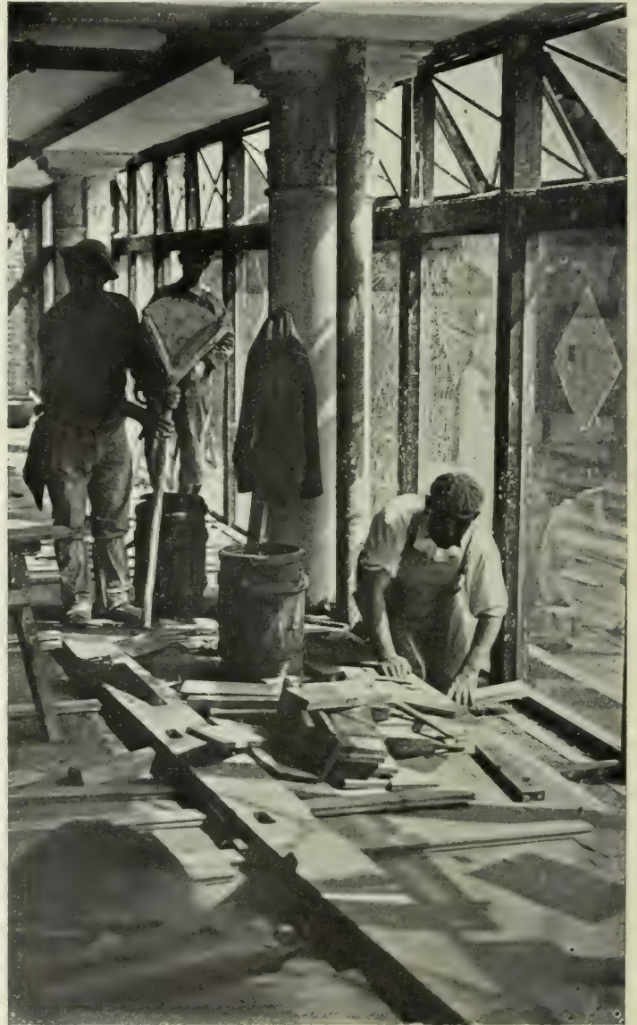
A CARPENTER LAYING A FLOOR
