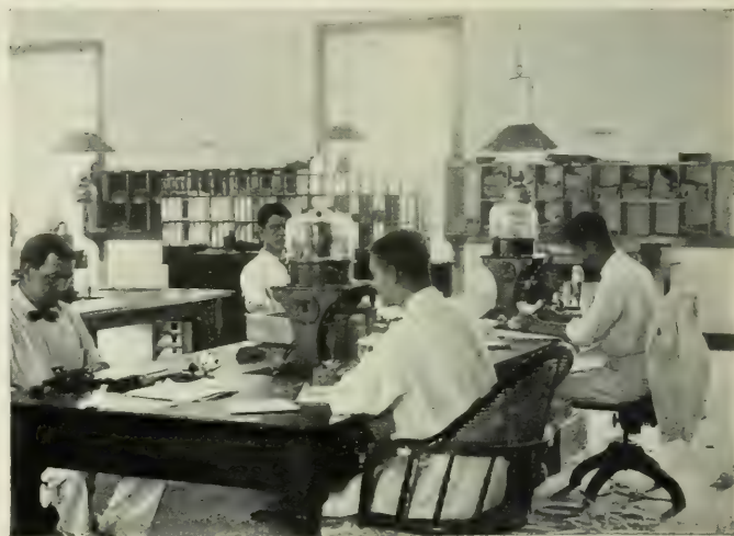
A CABLE STATION AT ST. VINCENT
