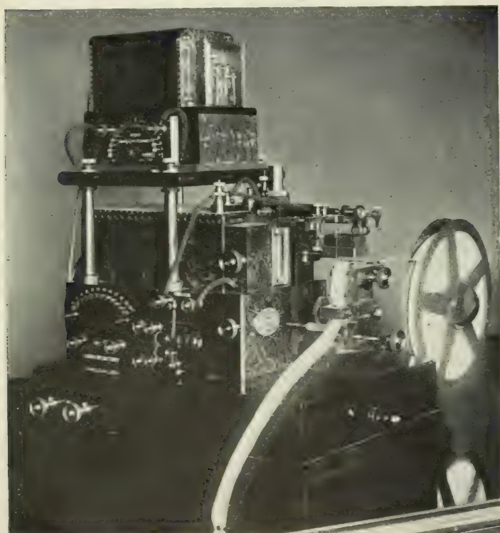
A MODERN LONG DISTANCE SIPHON RECORDER
