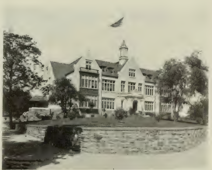
A MODEL CITY SCHOOL Showing shrubbery presented by residents of the neighborhood
