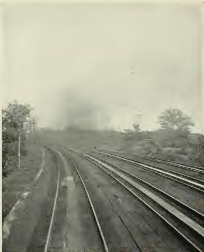
TRACK TANKS WHICH SUPPLY WATER TO LOCOMOTIVES WHILE TRAVELING AT FULL SPEED
