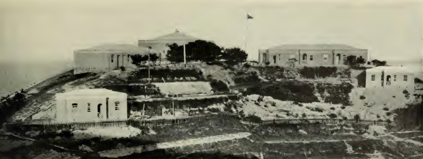
THE EASTERN EXTENSION CABLE STATION AT SHARP PEAK
