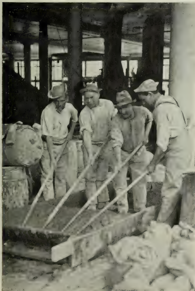
MIXING MORTAR: ONE OF THE LEAST SKILLED TRADES
