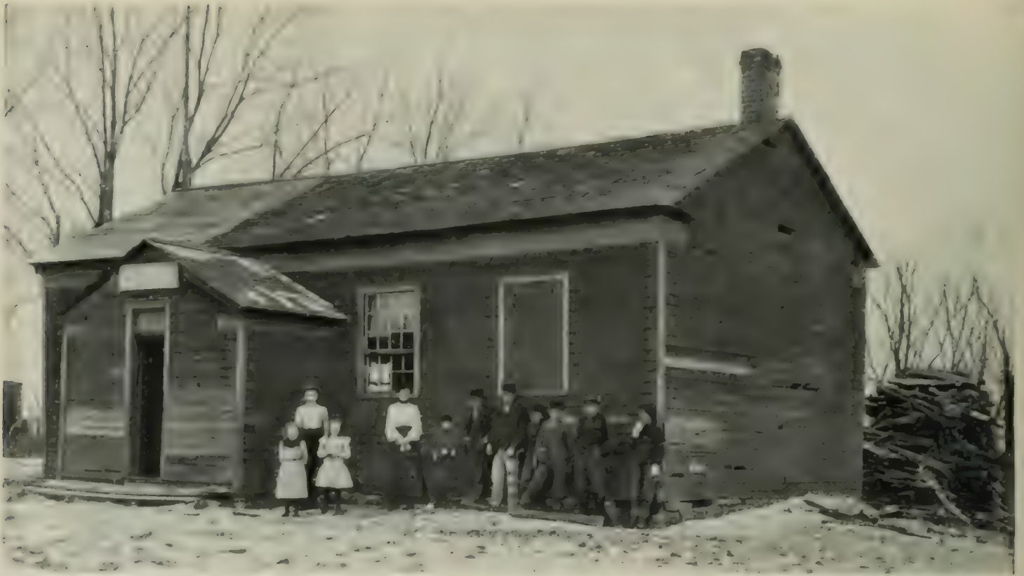
THE WORST SCHOOL BUILDING IN WINNEBAGO COUNTY—THE RESULTS OF NEGLECT
