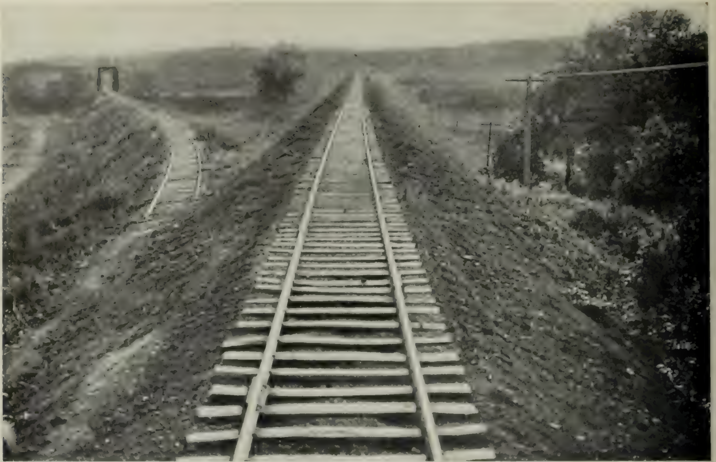
STRAIGHTENING THE TRACK AND IMPROVING THE GRADE
