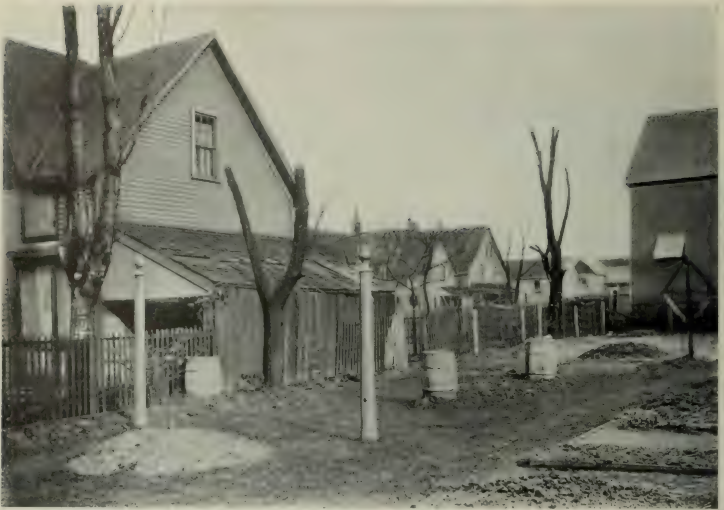
A NEGLECTED BACK YARD
