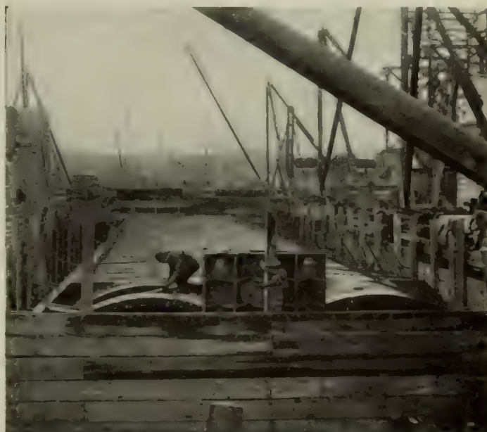
BOLTING THE HARLEM RIVER TUNNEL SECTIONS AND COVERING THEM WITH CONCRETE
