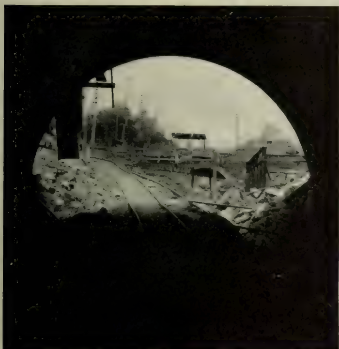
WHERE TUNNEL CHANGES TO TRENCH
