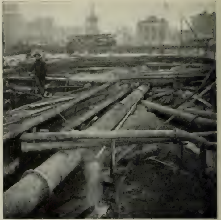
THE TANGLE OF PIPES THAT THE DIGGERS HAD TO DISPOSE OF
