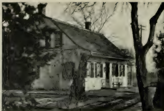
AN IDEAL VILLAGE HOUSE JUST OFF THE MAIN STREET AND AT RIGHT ANGLES TO IT
