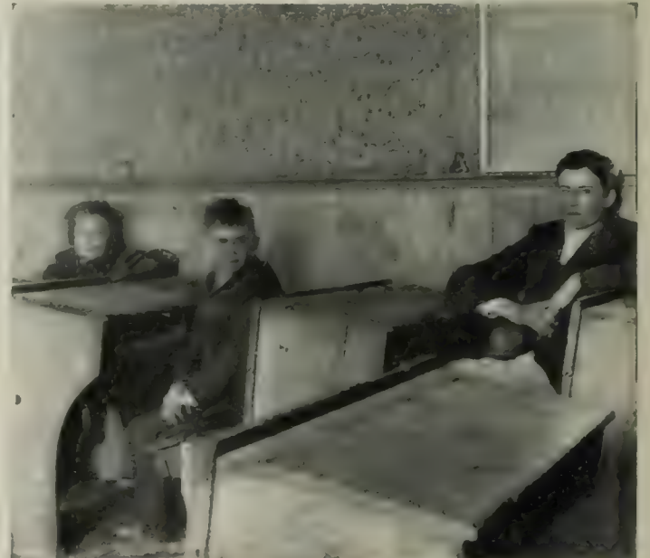
THE INTERIOR OF THE WORST SCHOOL-HOUSE
