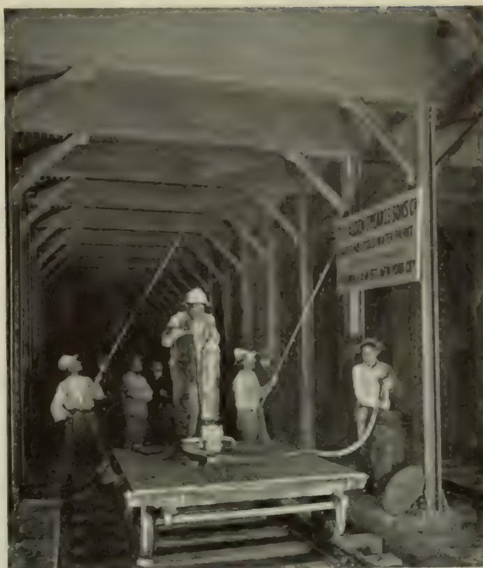
PAINTING THE INTERIOR WITH PNEUMATIC SPRAYS
