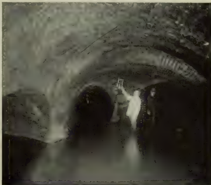
ONE OF THE SEWERS THAT HAD TO BE DIVERTED
