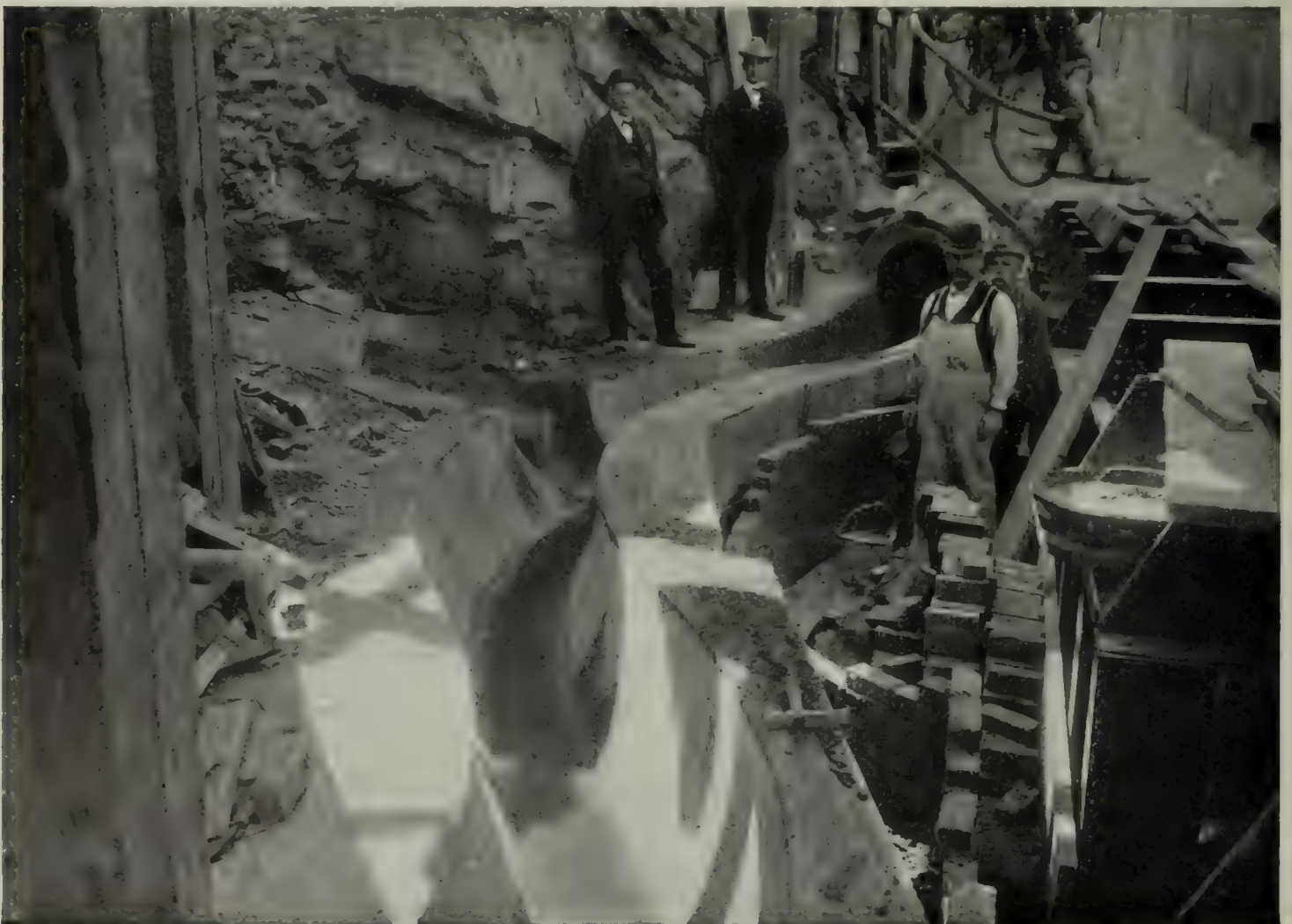
AFTER THE BRICKLAYERS STRUCK, SEWERS WERE MADE OF CONCRETE
