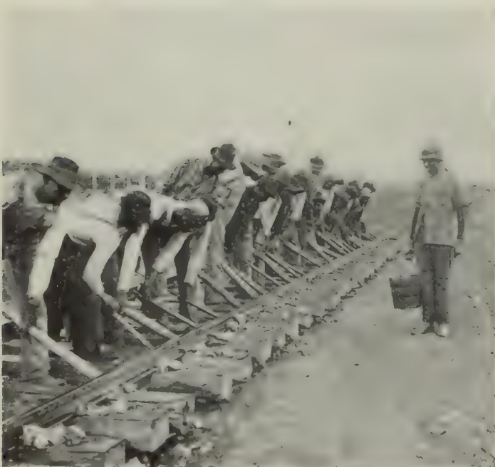
THROWING THE TRACK BODILY FROM A TEMPORARY TO A PERMANENT BED
