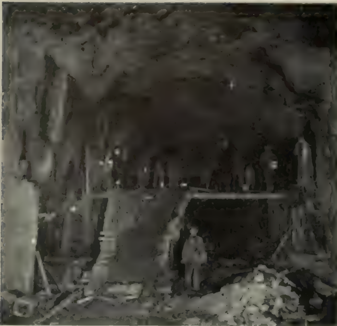
WHERE MINING WAS CARRIED ON AT 167th STREET 150 FEET UNDERGROUND
