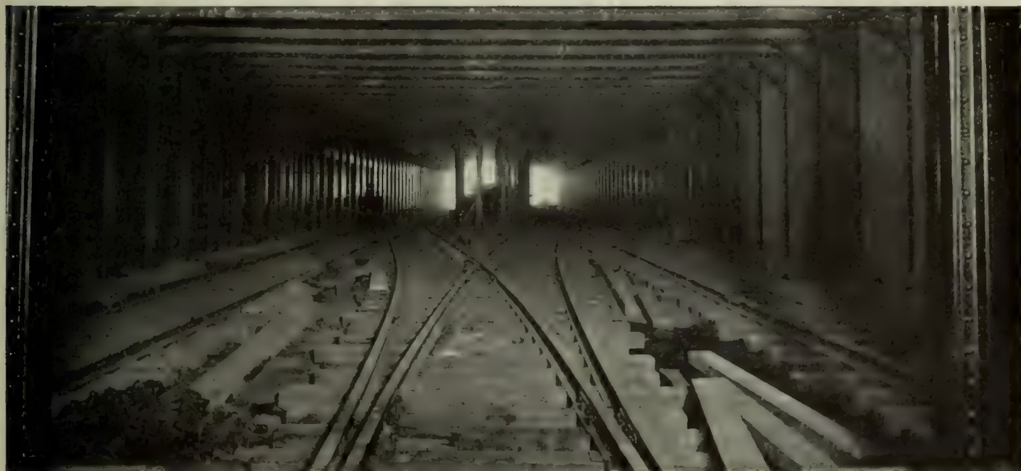
THE CONSTRUCTION OF THE SUBWAY IS OF THIS GENERAL CHARACTER
