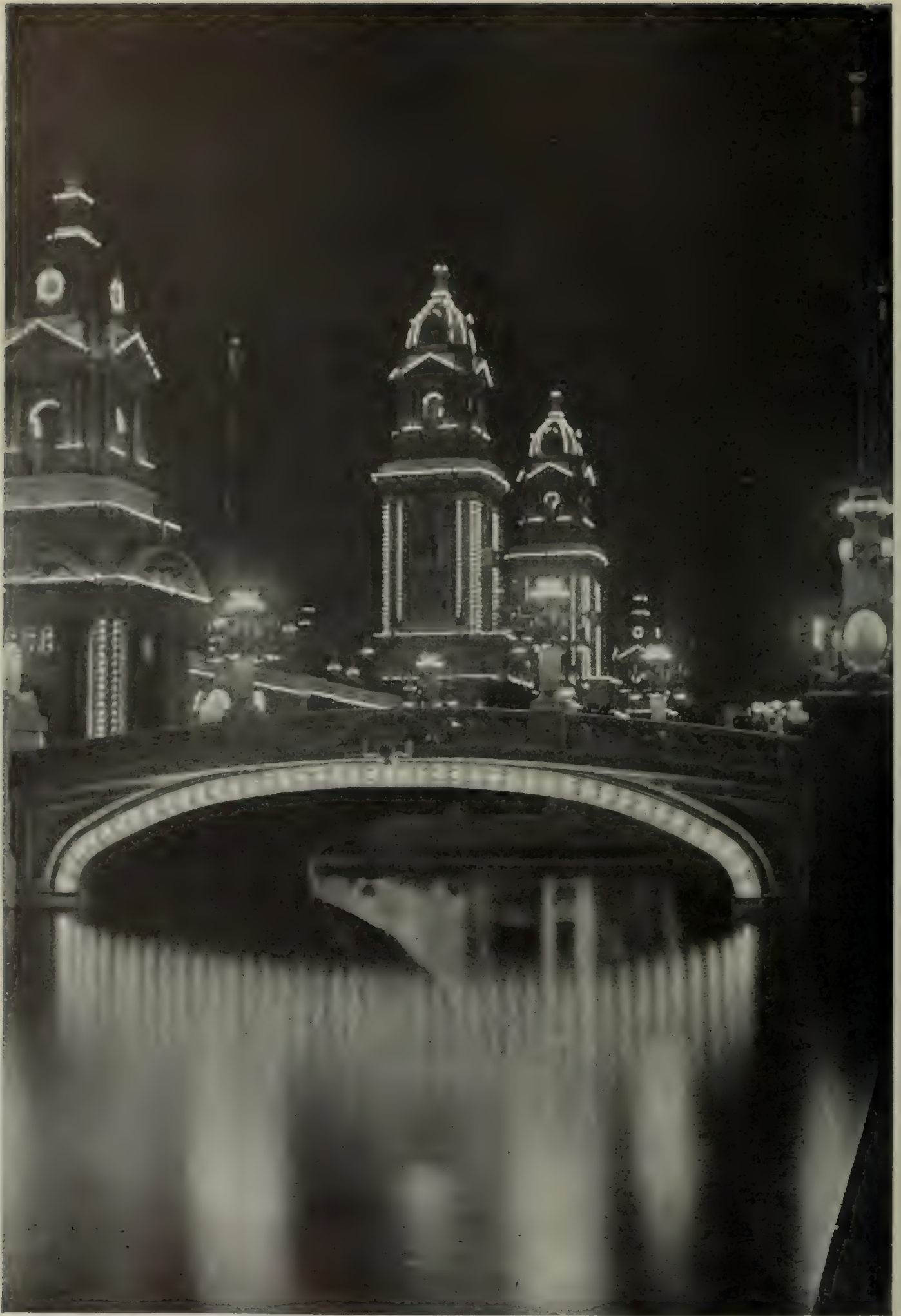
THE PALACE OF MACHINERY
