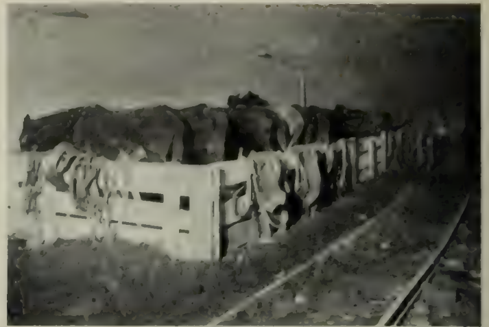
THE MULES STABLED IN THE MINE AT 167th STREET
