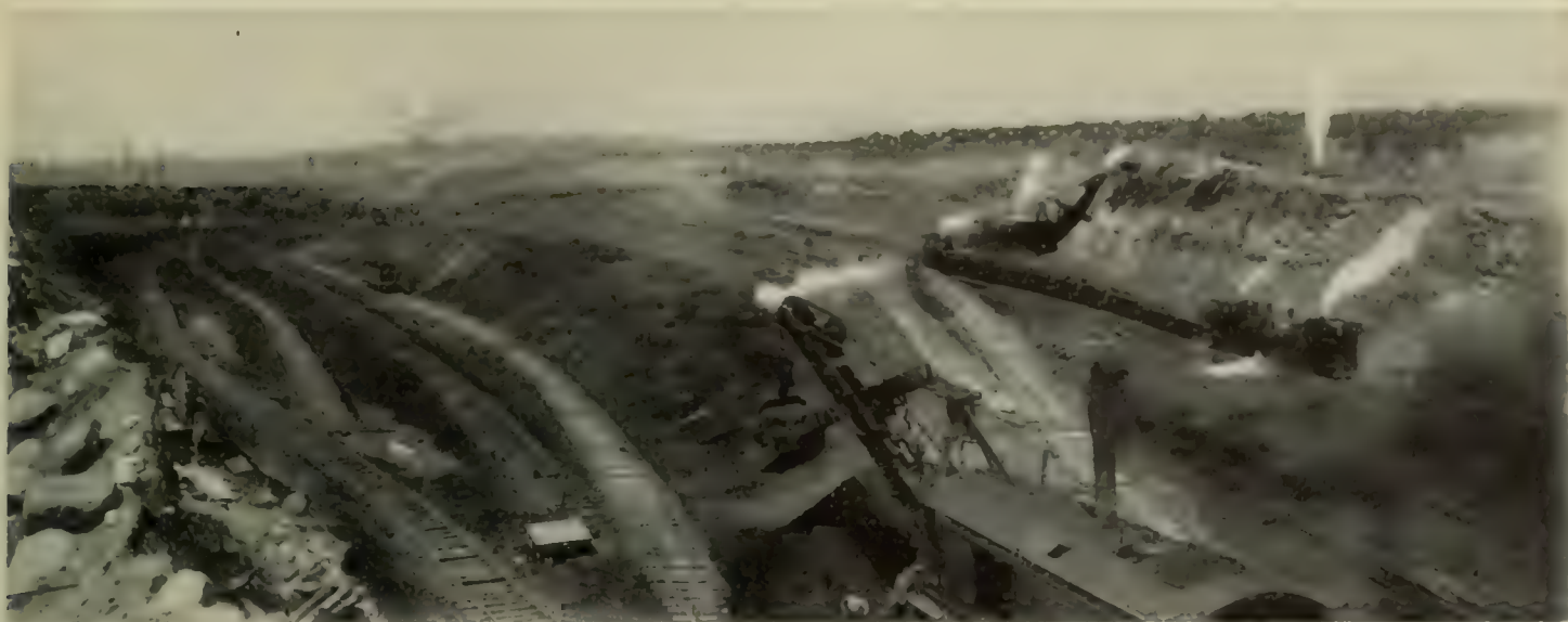
THE PHOTOGRAPH SHOWS THREE SHOVELS "STRIPPING" SURFACE SOIL, AND ONE, IN THE FOREGROUND, "BUCKING" THE ORE-BANK
