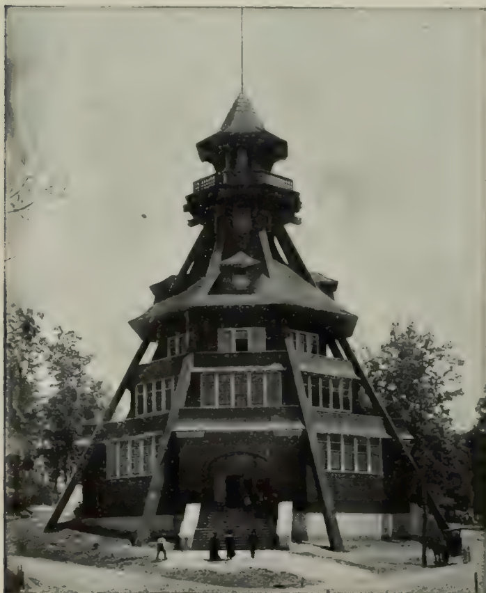
WASHINGTON'S STATE BUILDING IS SUPPORTED BY SINGLE TIMBERS 110 FEET LONG
