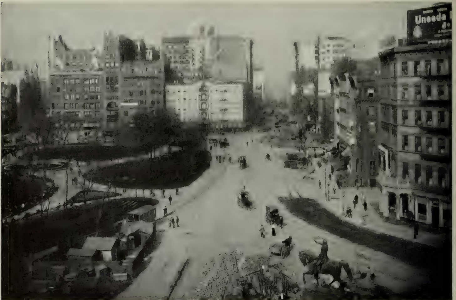
UNION SQUARE WITH THE SUBWAY COMPLETED—CARTS REMOVING THE DEBRIS
