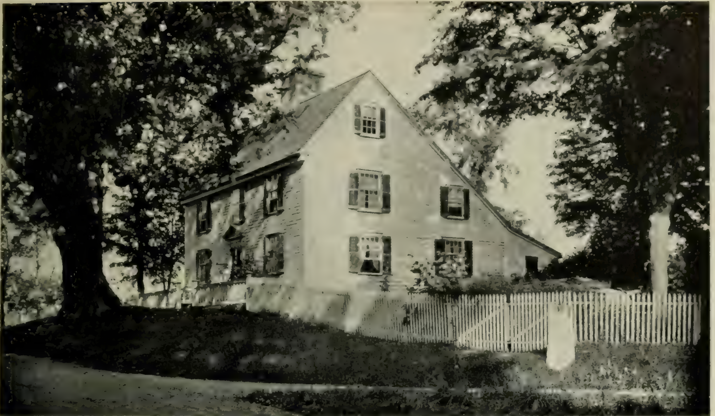
AN IDEAL LANDMARK AT THE FORK IN THE ROAD—THE APPROACH TO THE IDEAL VILLAGE
