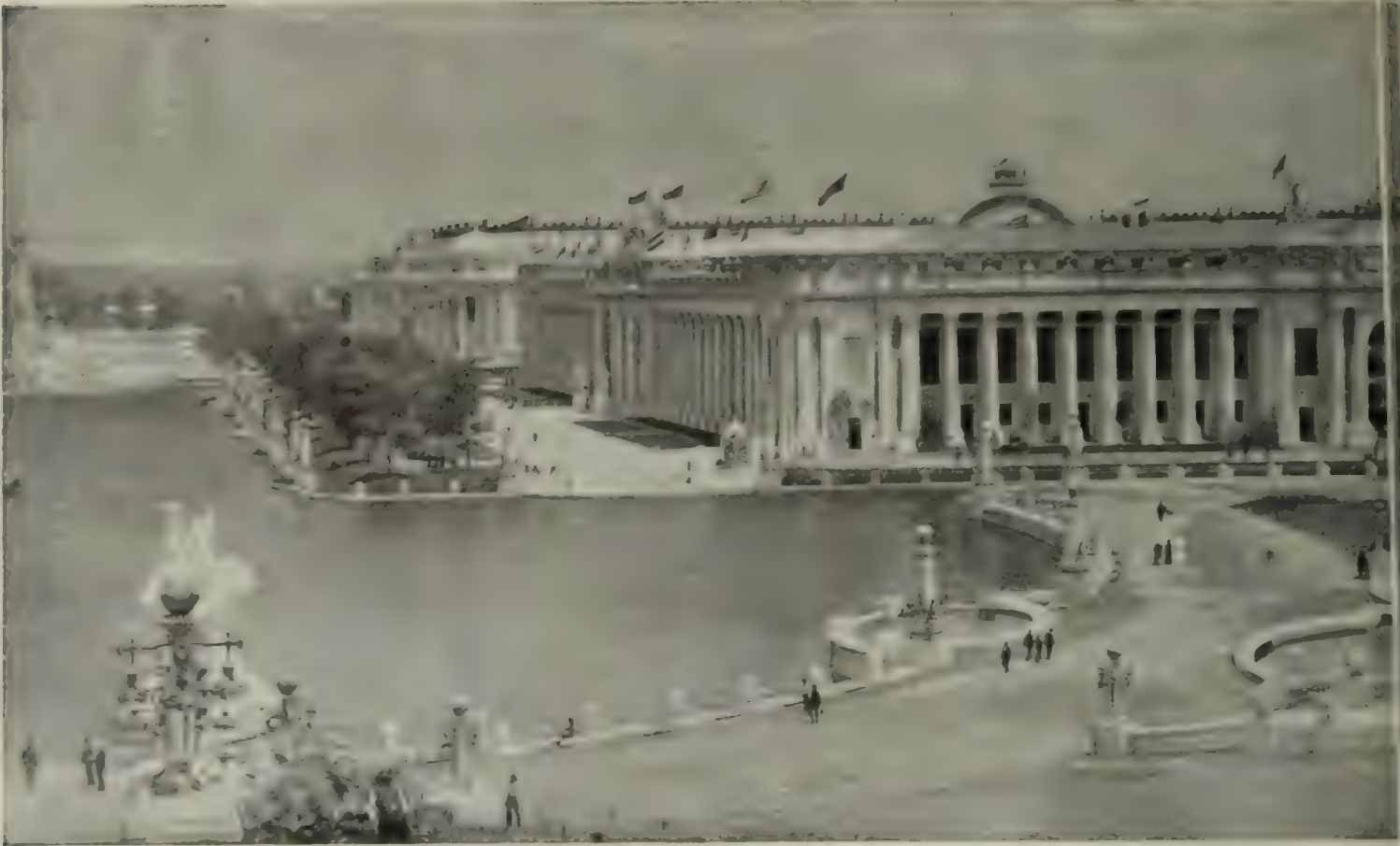
VIEW FROM HALF-WAY UP THE CASCADE
