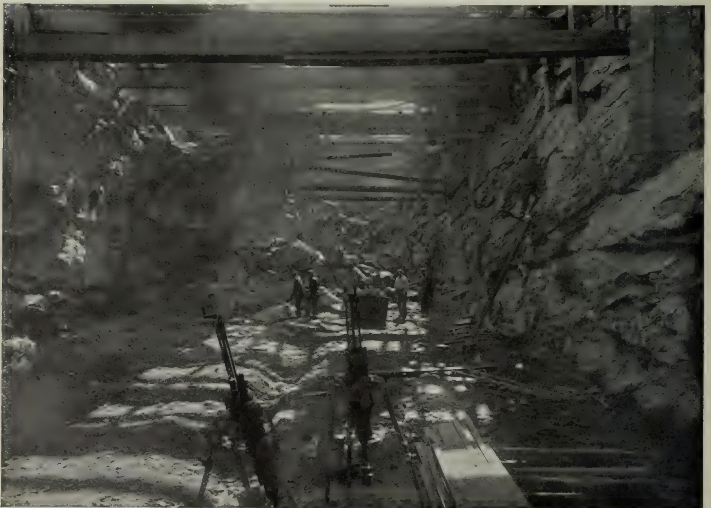
BEFORE THE CONCRETE FLOOR WAS LAID
