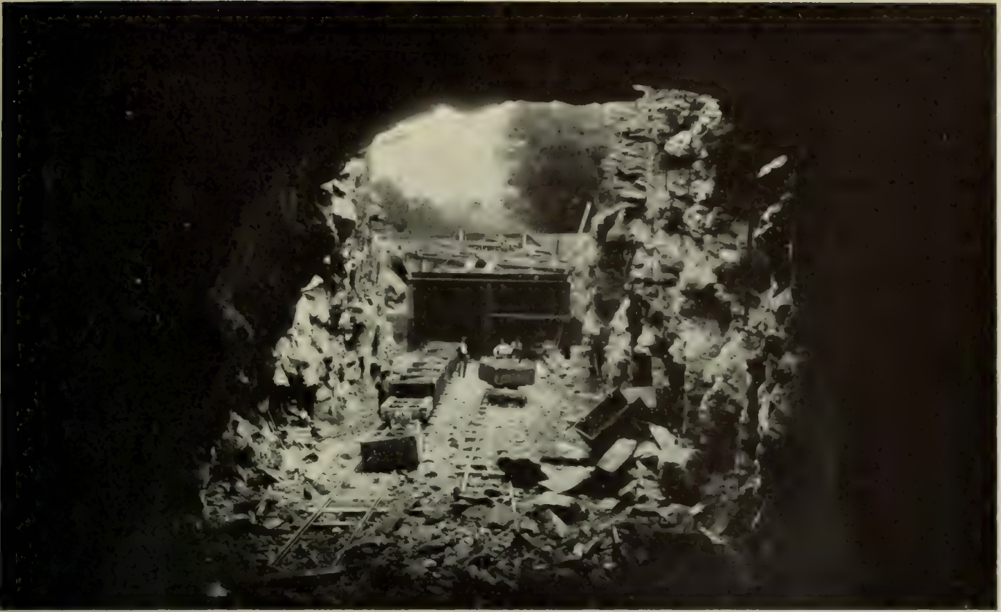
THE SUBWAY ADVANCING THROUGH THE SOLID ROCK OF UPTOWN NEW YORK
