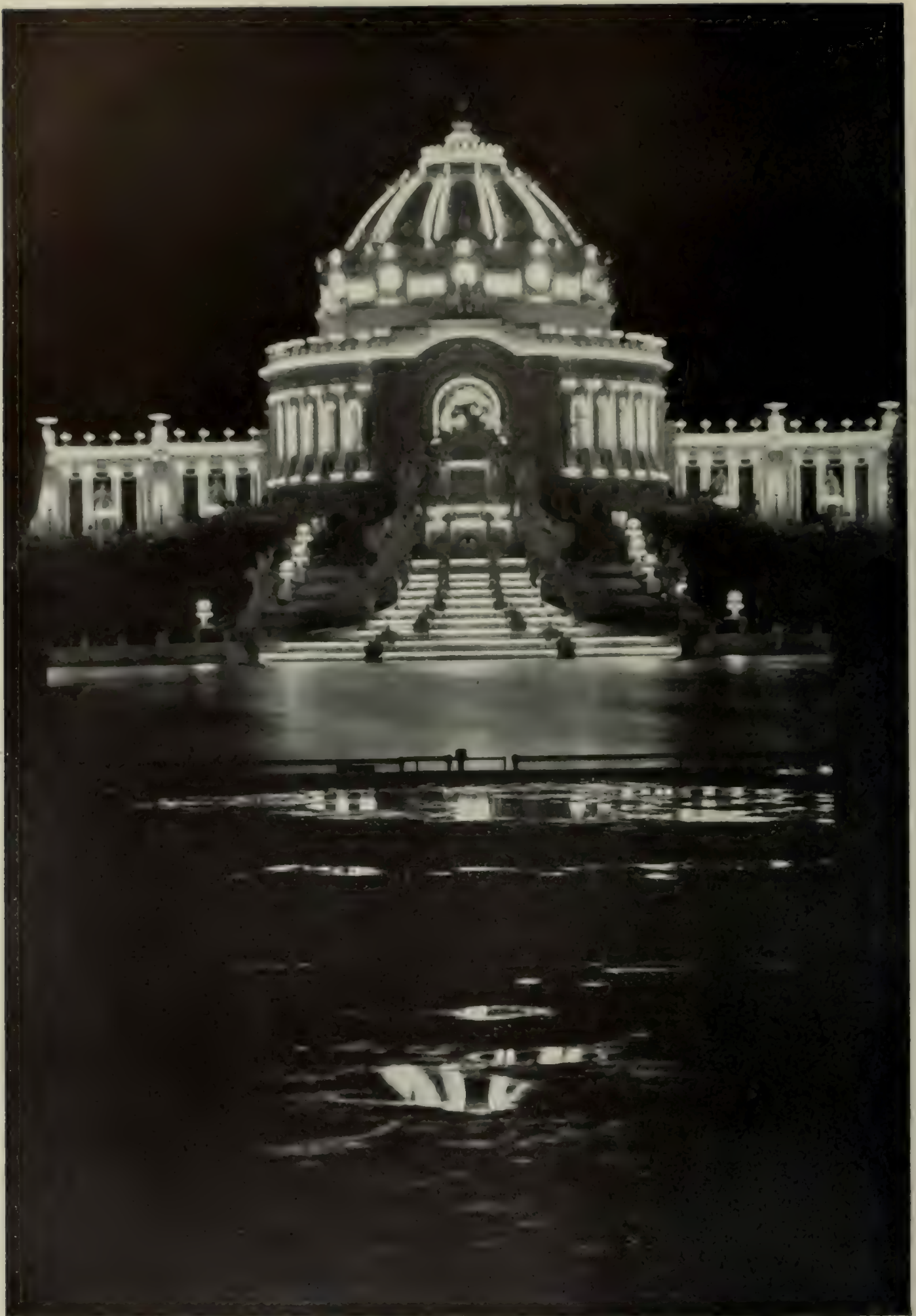
A VIEW OF FESTIVAL HALL AND THE COLONNADE OF STATES AT NIGHT This is the central spectacle of the Fair, and from this radiate the successions of palaces that contain the principal exhibits
