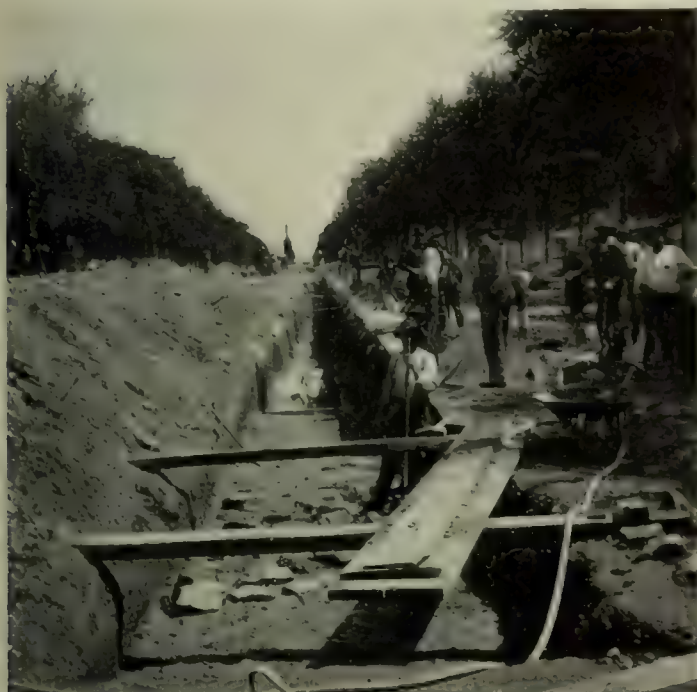
THE FIRST STEPS IN OPENING A TRENCH FOR THE SUBWAY
