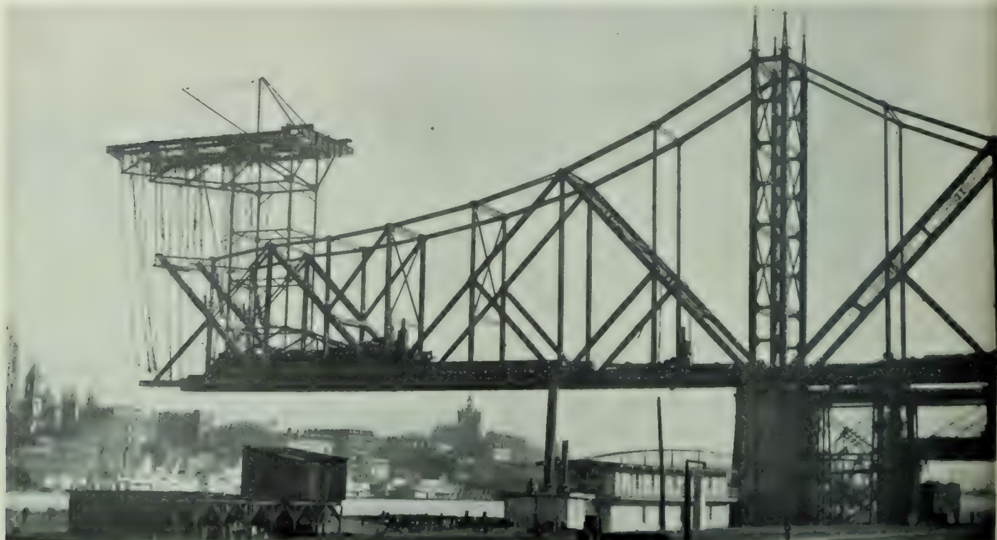
THE METHOD OF CONSTRUCTION
