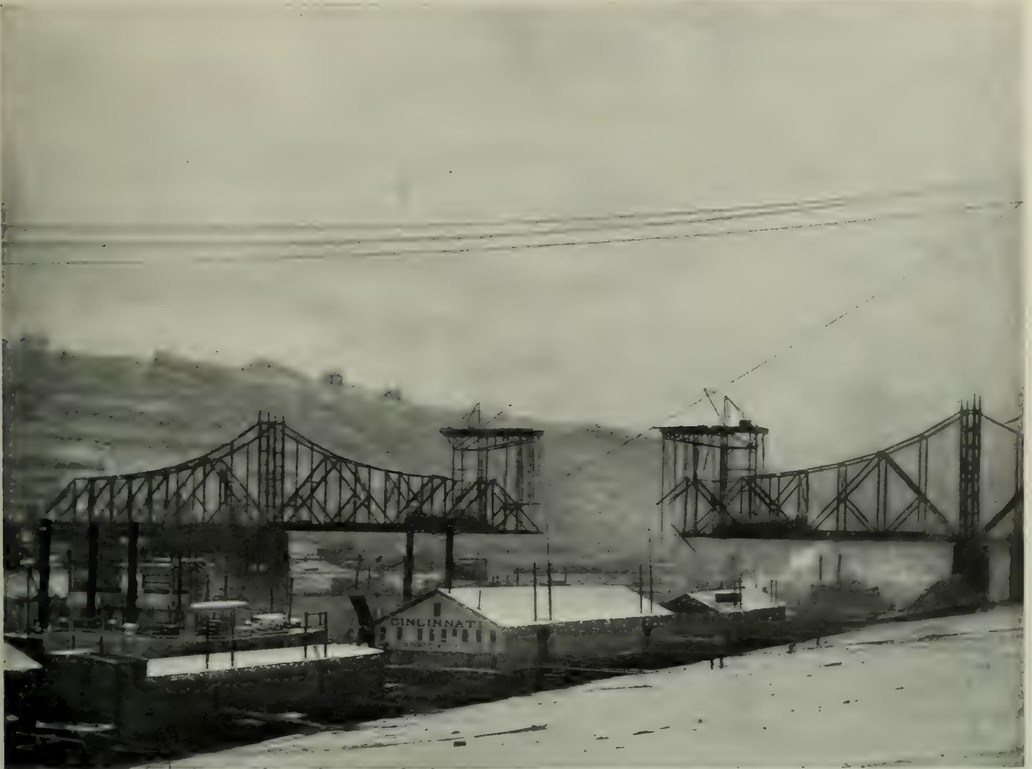
THE BRIDGE APPROACHING THE CENTRE
