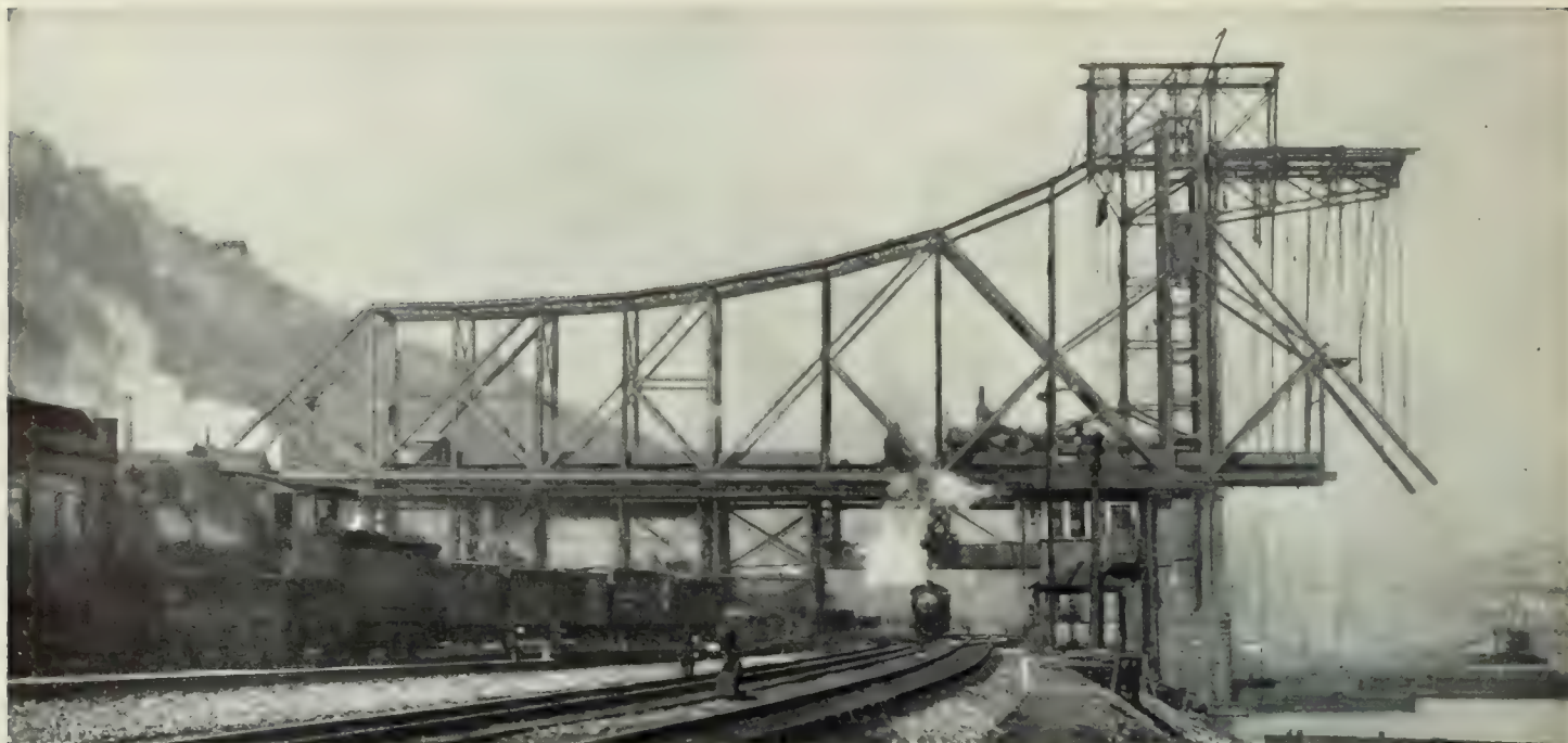
STARTING THE WABASH CANTILEVER BRIDGE OVER THE MONONGAHELA
