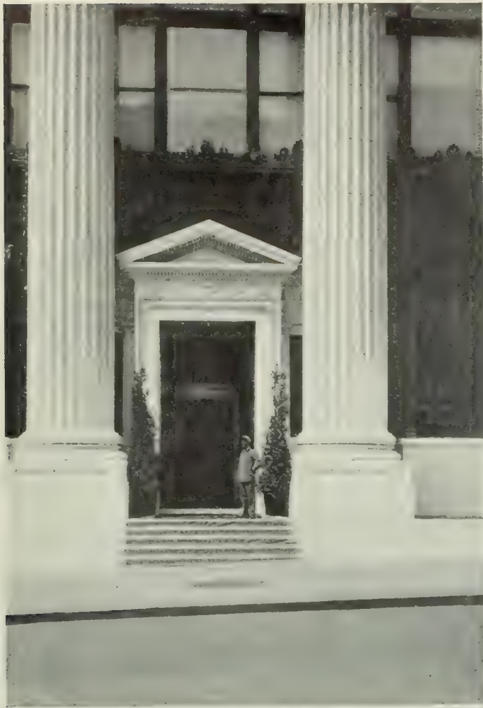
Photographed by A. Radclyffe Dugmore THE BRONZE AND MARBLE ENTRANCE to the building of the Knickerbocker Trust Company, New York
