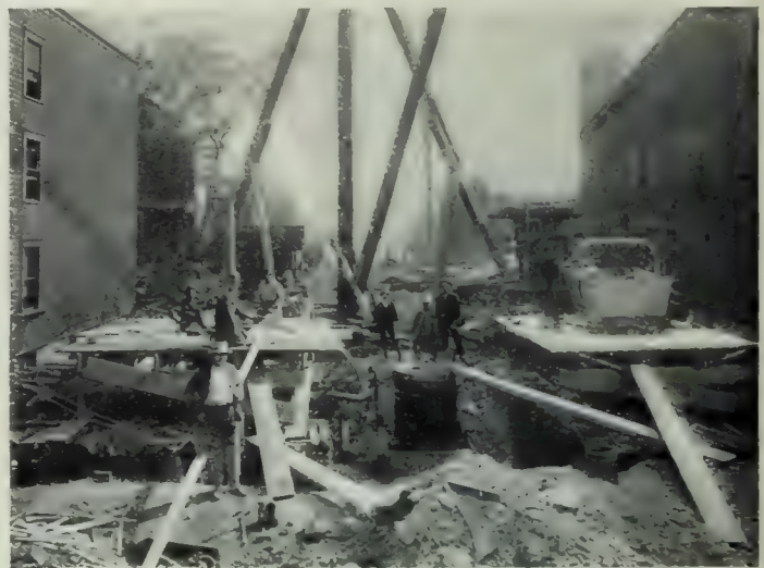
FILLING THE CAISSONS WITH CONCRETE
