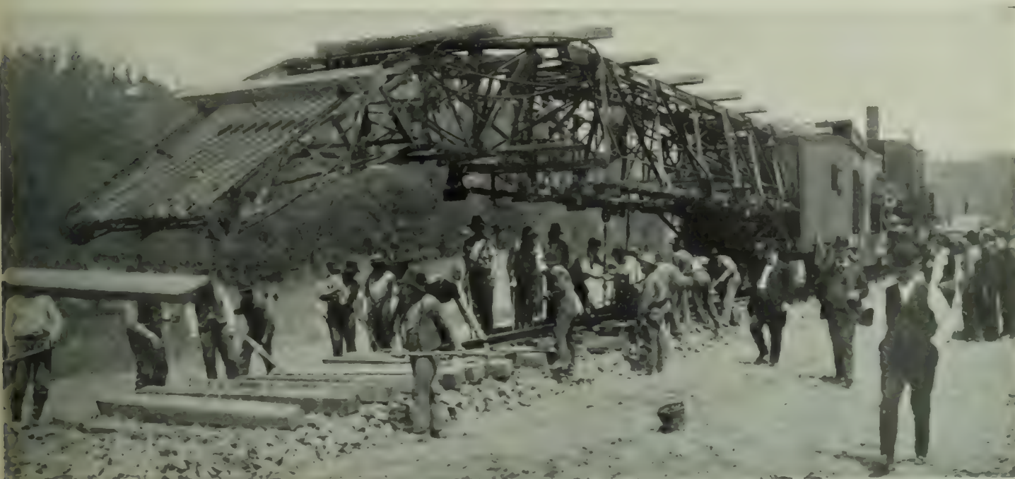
LAYING TRACK BY MACHINERY
