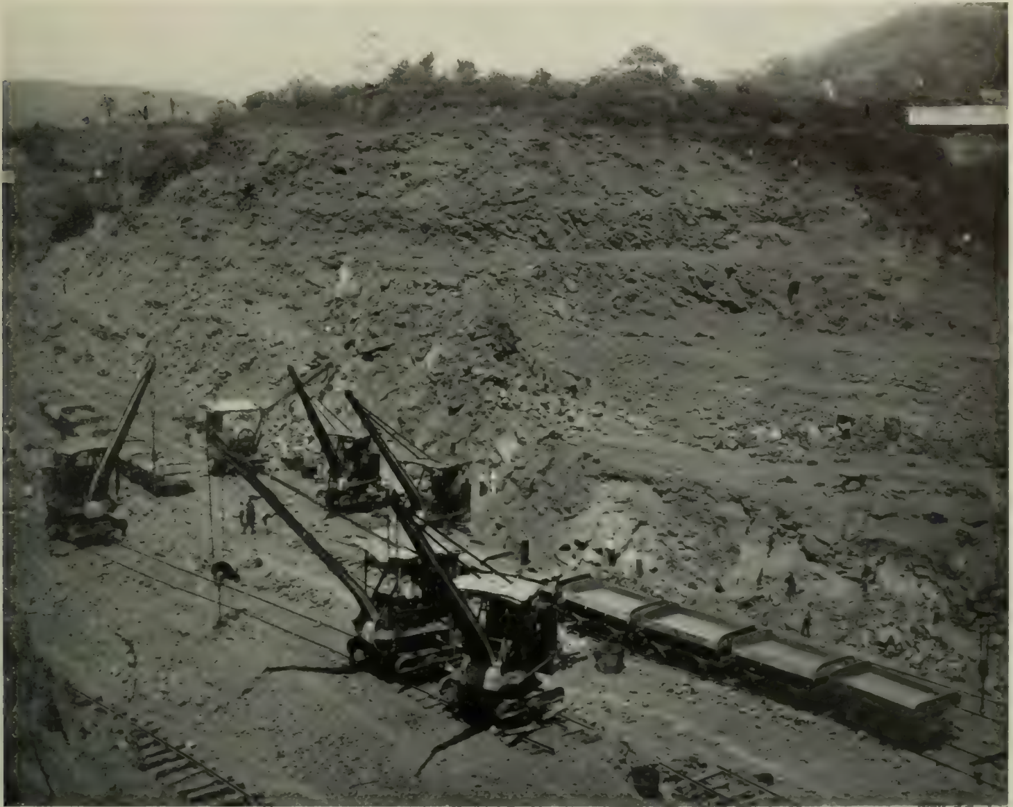
THE METHOD USED BY THE FRENCH COMPANY TO CUT THE PANAMA CANAL
