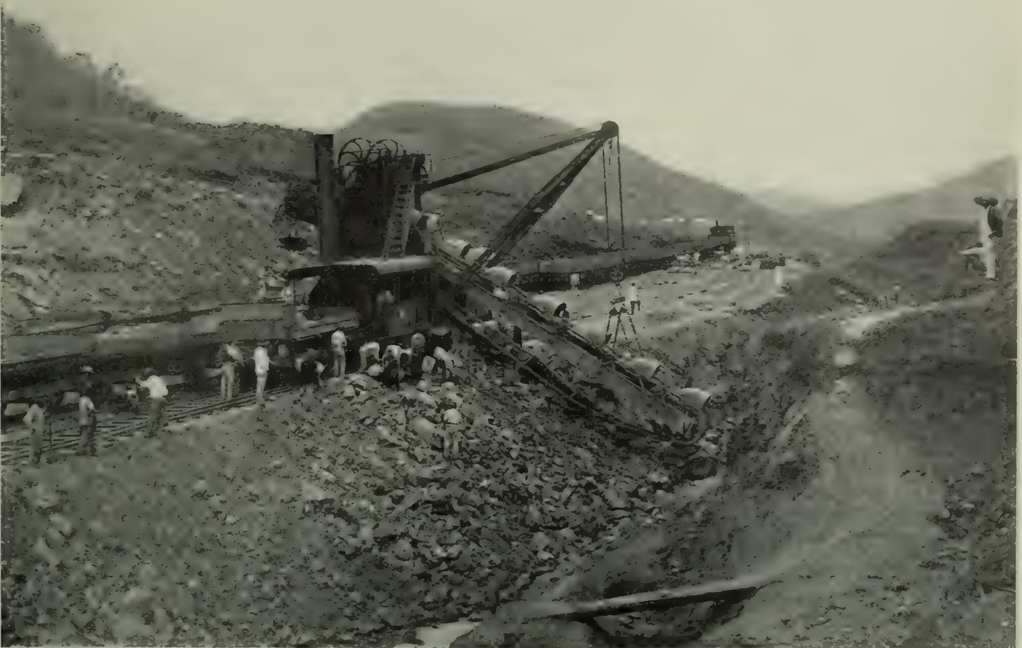
AN EXCAVATOR AT WORK IN THE CULEBRA CUT
