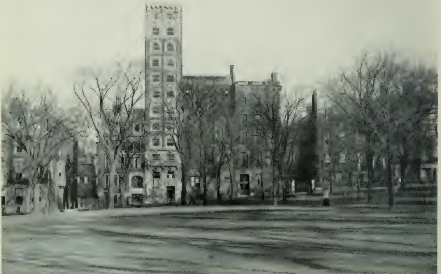
A SKY-SCRAPER INTRUDING ON HISTORIC BEACON STREET
