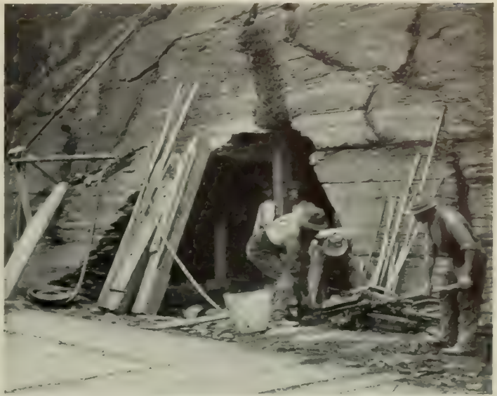
BEGINNING THE TUNNEL Under Mt. Washington
