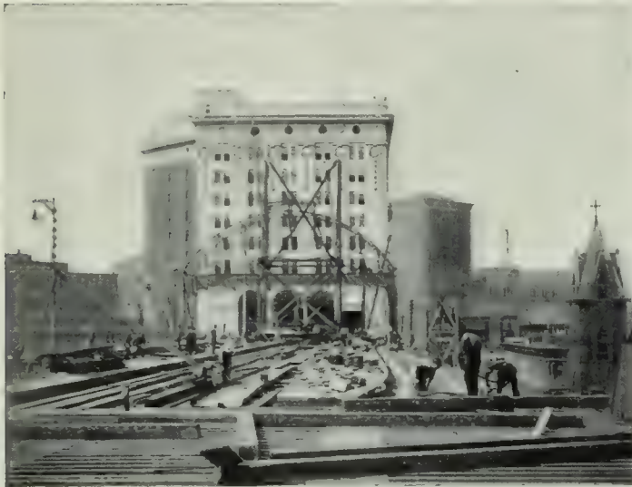
BUILDING THE TRAIN-SHED FOR THE STATION
