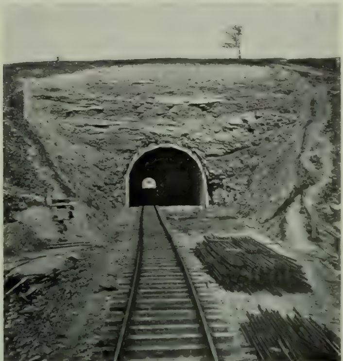
THE TWIN TUNNELS ON THE NEW LINE
