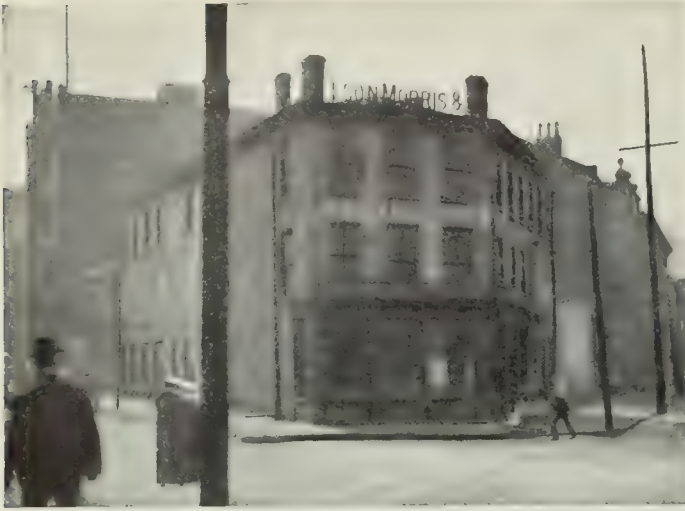
THE SITE OF THE TERMINAL Before work was begun
