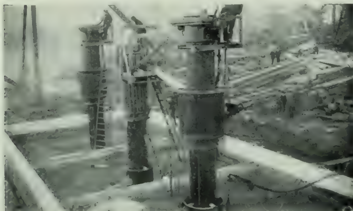
CAISSON WORK ON THE BRIDGE PIERS
