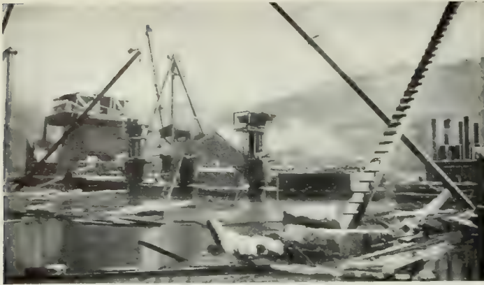
CAISSON WORK FOR THE NEW BRIDGE
