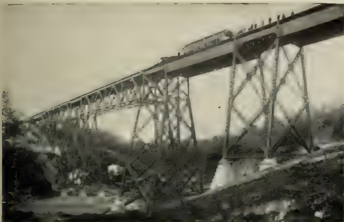
THE WHISKY RUN VIADUCT
