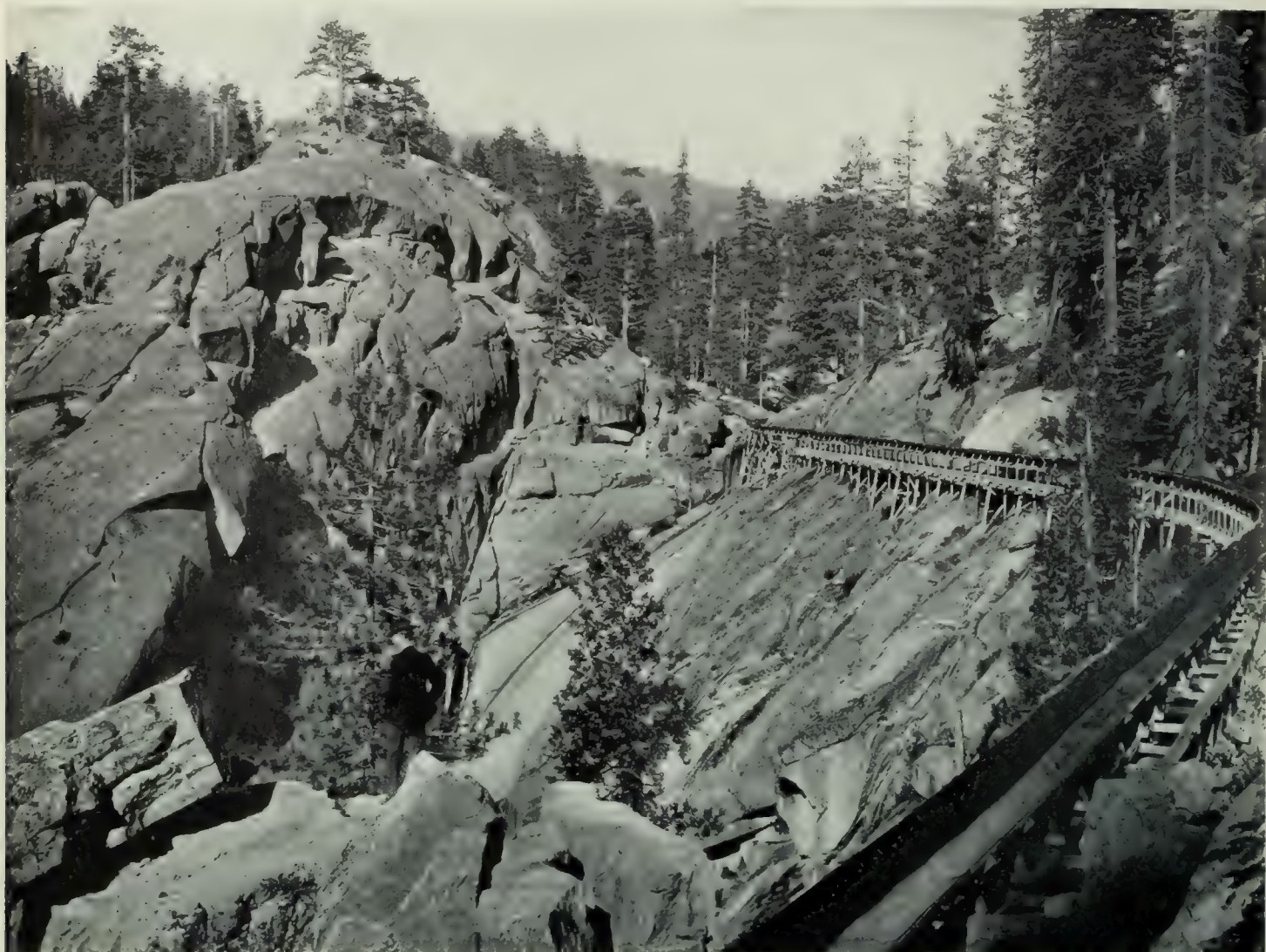
A LUMBER FLUME IN THE SIERRA NEVADA MOUNTAINS
