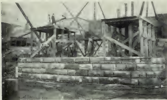
BEGINNING THE MASONRY WORK
