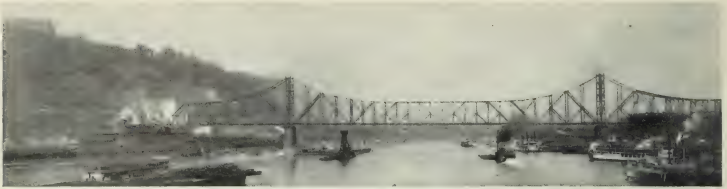
THE STRUCTURAL BEAMS CONNECTED AT THE BOTTOM
