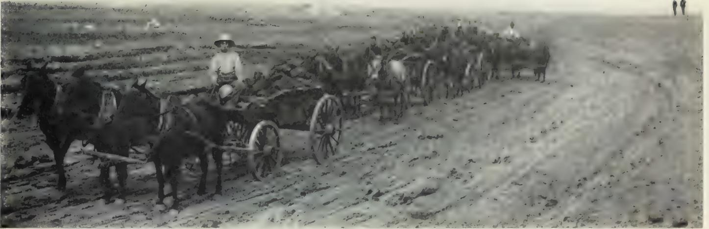
MAKING THE MAIN DITCH FOR THE LARGEST IRRIGATION PROJECT IN NORTH AMERICA
