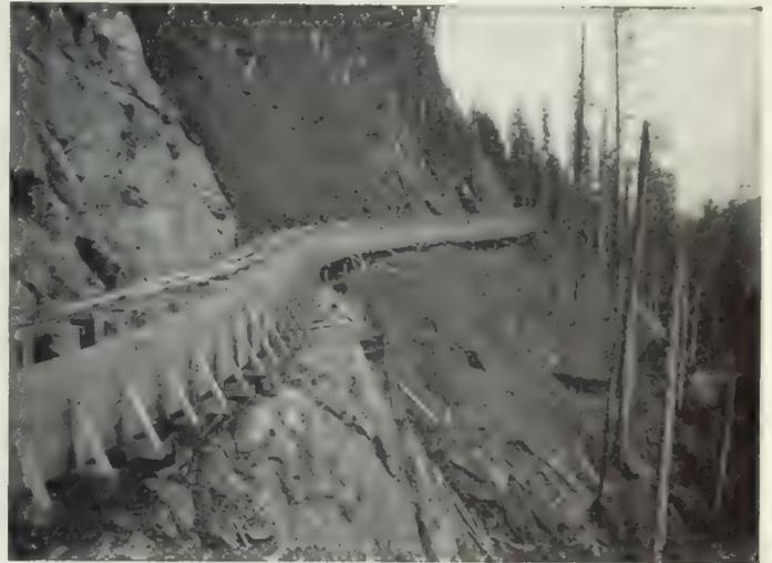
THE FLUME THAT CARRIES THE WATER FROM THE MELTING SNOWS TO THE ELECTRIC POWER HOUSE
