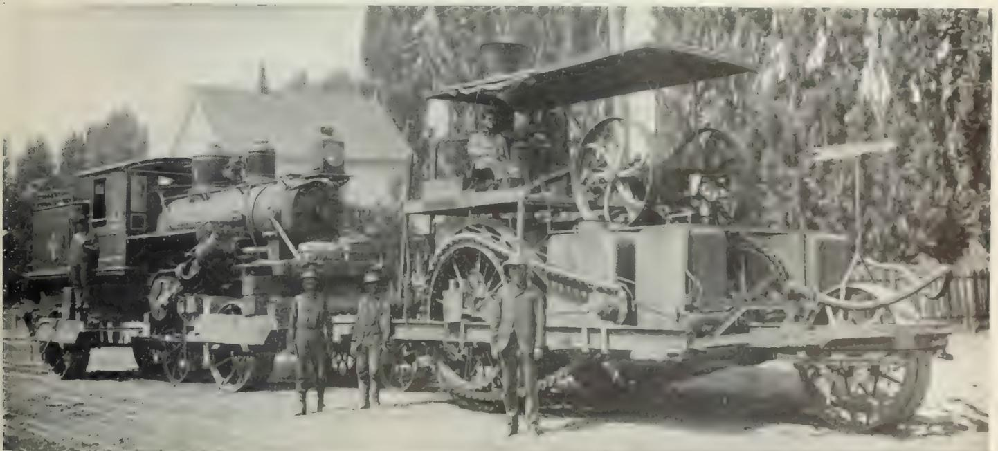
A 60-HORSEPOWER AUTOMOBILE ENGINE HAULING A 36-TON LOCOMOTIVE SEVEN MILES ON GRADES IN COLORADO RANGING FROM 8 PER CENT. TO 12 PER CENT.
