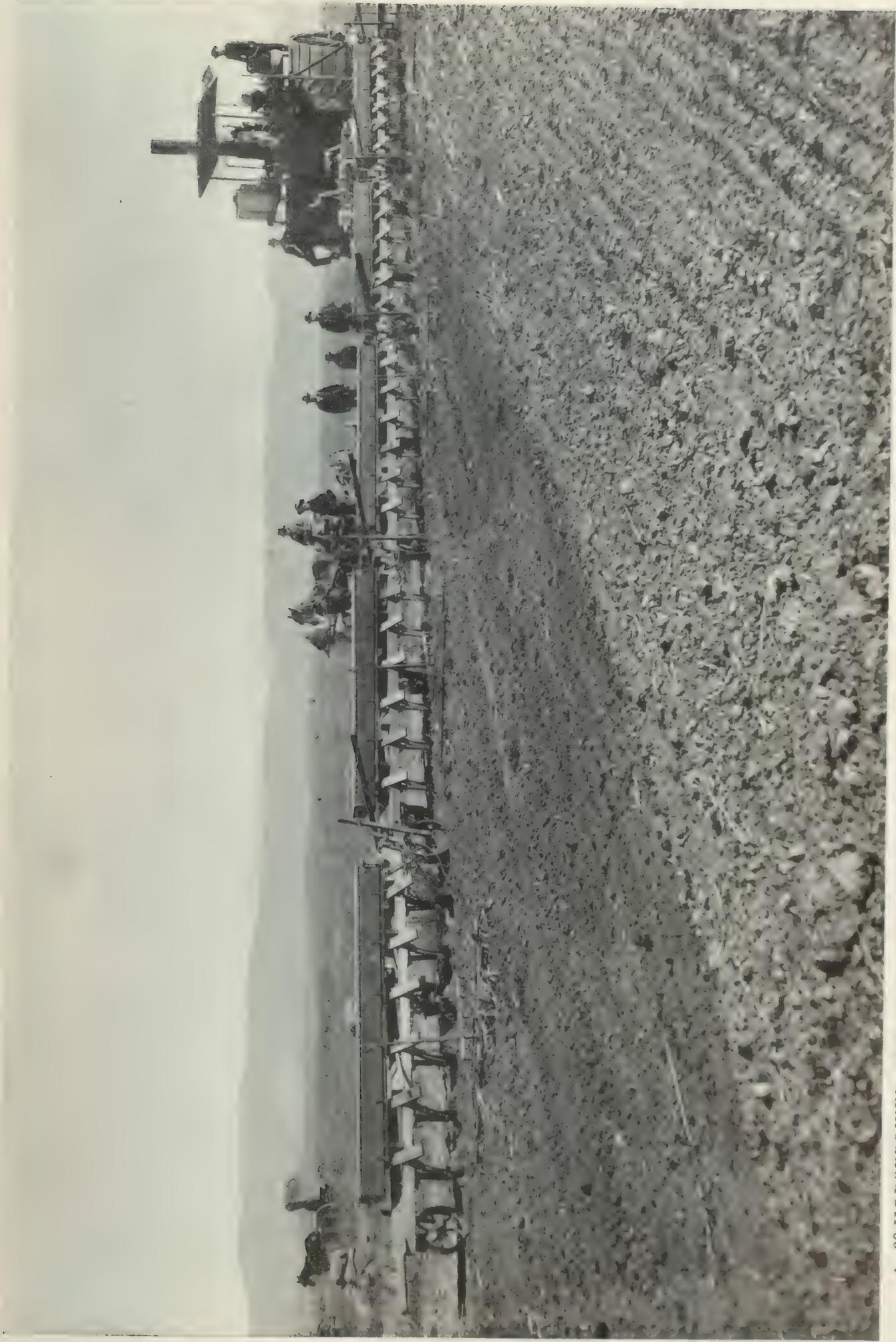
A 60-HORSEPOWER STEAM ENGINE PULLING THIRTY FEET OF GANG PLOWS WITH SEEDERS IN FRONT AND HARROWS BEHIND THE PLOWS. IT AVERAGES EIGHTY ACRES A DAY
