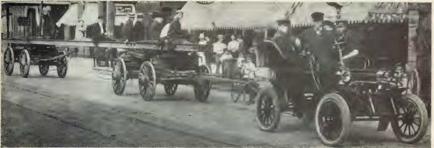
AN ORDINARY AUTOMOBILE PULLING  $5\frac{1}{2}$  TONS OF RAILWAY IRON UP A 4 PER CENT. GRADE IN CANTON, OHIO
