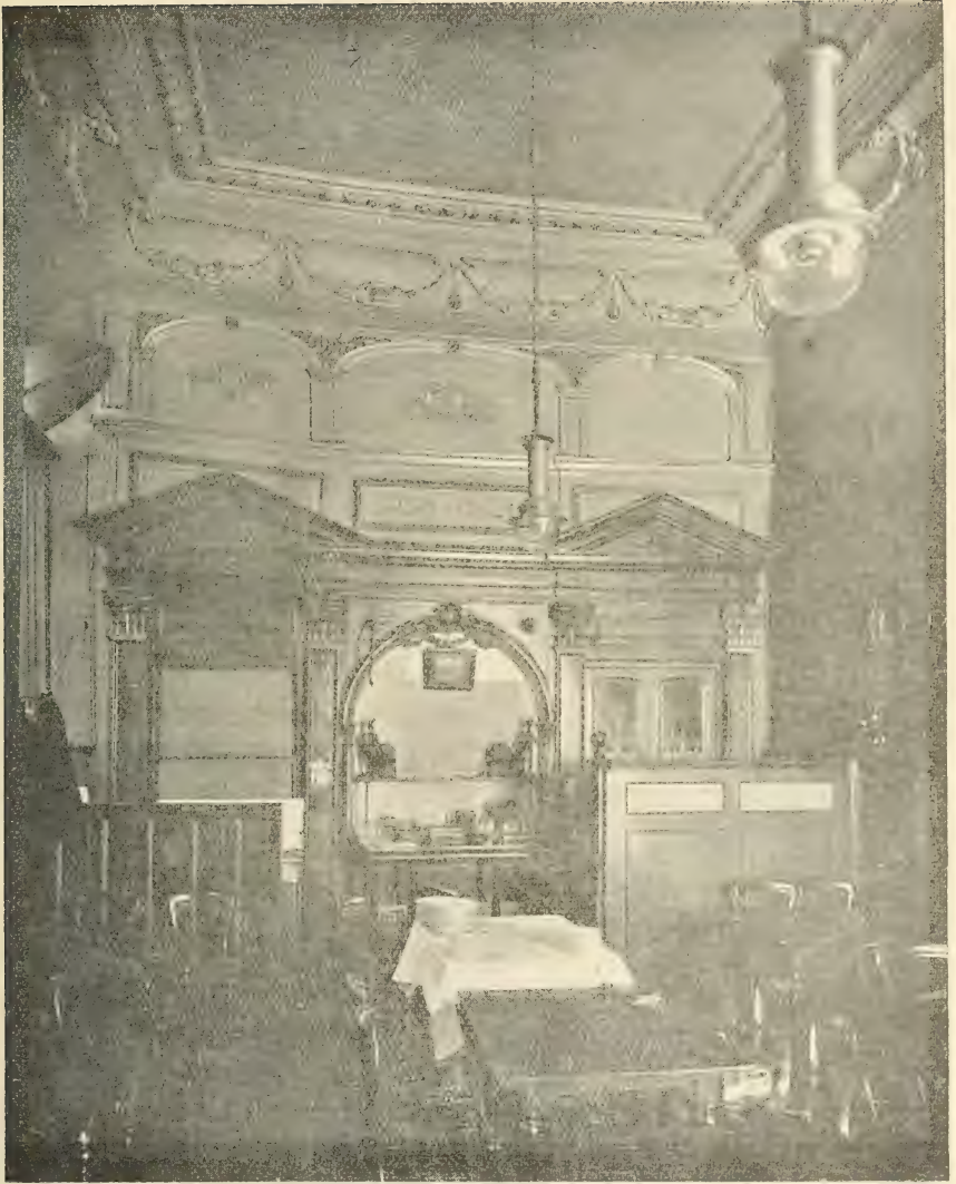
The interior and west view of the Hall in the old building of the Masons' Company, Masons' Avenue, Basinghall street, London. The pediment and other wood-work in the two doorways as well as the decorations in the frieze above with the ornamental plaster work and cornice are as they were during the occupancy of the building by the Masons' Company.
