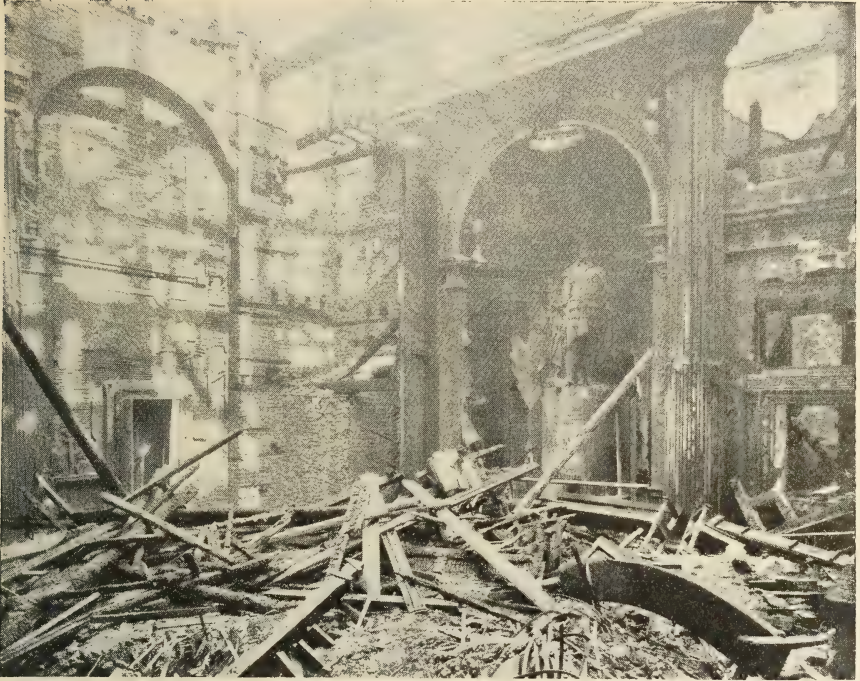
S. E. COR. OF FREEMASONS' HALL. THE FIRE OF MAY, 1883, ORIGINATED A LITTLE TO RIGHT OF OPEN DOOR IN WALL.
