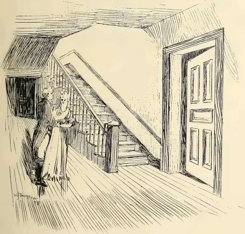
THE HALL AND STAIRCASE LEADING TO THE LODGE ROOM IN THE JONES HOUSE.
