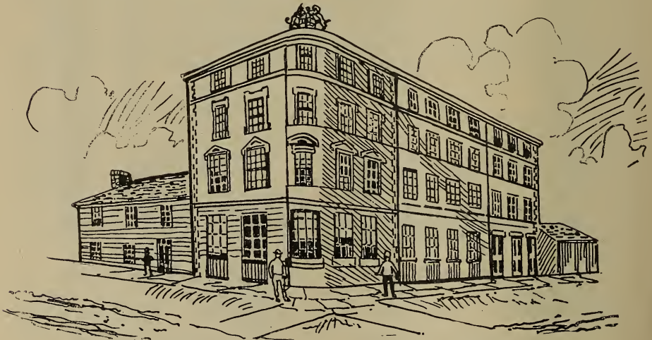
BUILDING, ON THE SOUTH-WEST CORNER OF CHURCH AND COLBORNE STS., WHERE KING SOLOMON'S LODGE MET, 1855-67.
