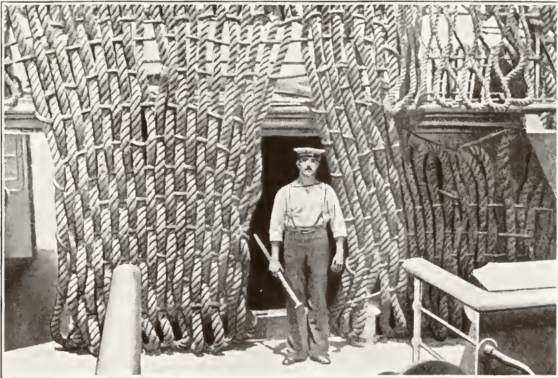
ROPE PROTECTION ON "CARMANIA" AGAINST SHELL SPLINTERS
