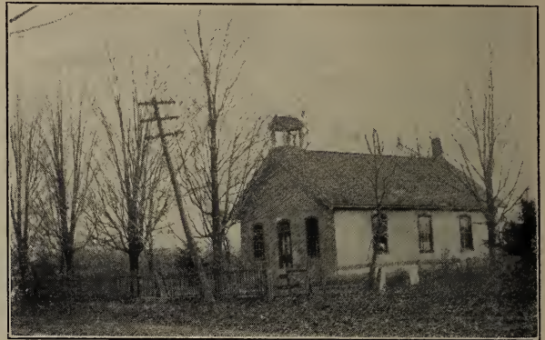
ABOVE THE AVERAGE RURAL SCHOOL. But Opportunities for Improvement in the Delapidated fences, leaning telegraph poles, etc.
