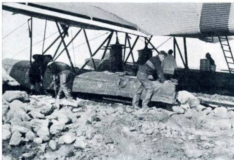
Repairing Floats at Low Tide
