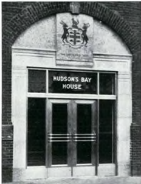
New doorway at the Winnipeg offices.
