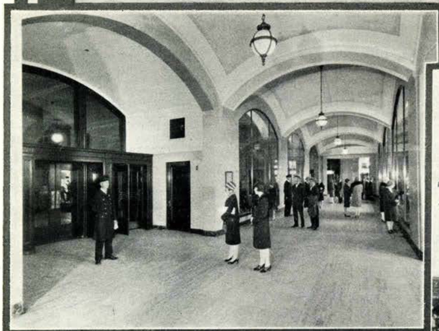
ARCADE, LOOKING WEST
