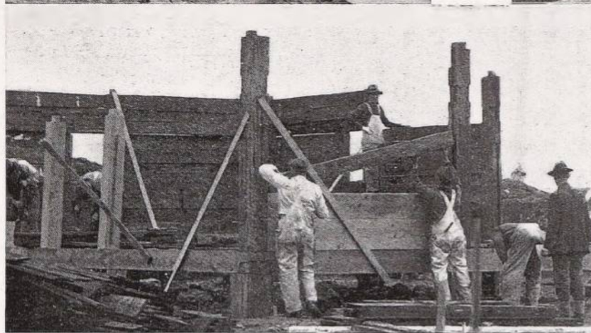
Upper left: Hand split cedar shakes. Above: The grooved upright of original granary. Centre: Reconstructing granary, using the original timber. Bottom: Broadaxe and original hand forged nails.
