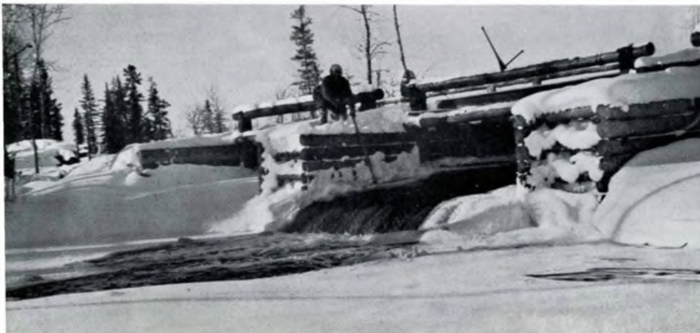
Dam in winter, three sluices closed.
