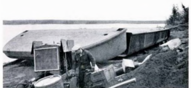
A steel barge being welded together.
