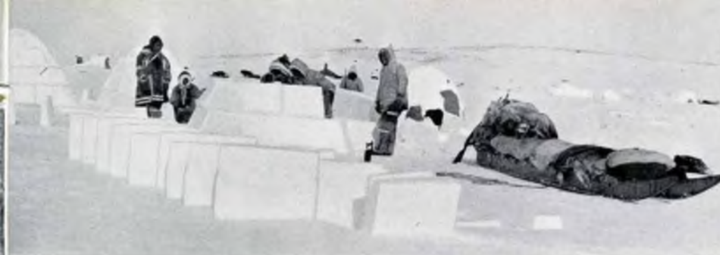
Below: It's child's play! Little Angootiapik on the left is cutting out blocks about ten inches thick and as deep as the saw is long. These are for the windbreak.
