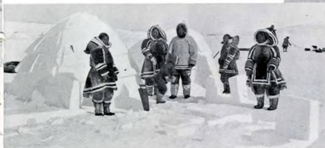
"Permanent" igloos, having a windbreak approach and a porch (with a store-room on the side) leading into the main living room with its raised floor. The window on the left hand house, near the saw, is of ice.
