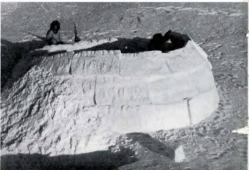
4. As the shadows lengthen, the dome begins to take shape. It will be completed by a key block on the very top. W. Gibson.
