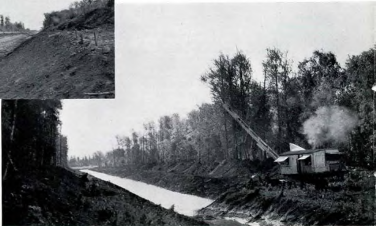
Dragline at work on Cut Beaver canal, which will carry water from the Saskatchewan to flood the muskrat marshes.
