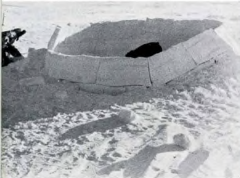
1. Father cuts the blocks out of the wind-packed snow with a saw, and builds them up around himself in a spiral, shaping them with his snow-knife. Mother shovels snow against the outside.
