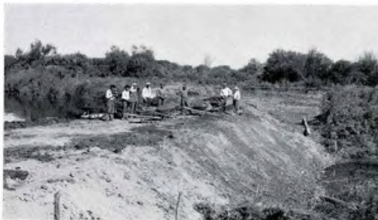
Another dam was built across Willow Creek.
