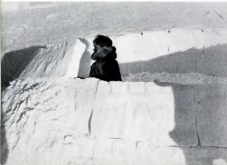
3. Layer number three, and the walls begin to lean inwards.
