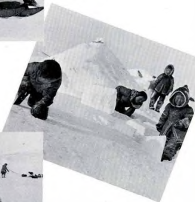
Below: It's child's play! Little Angootiapik on the left is cutting out blocks about ten inches thick and as deep as the saw is long. These are for the windbreak.
