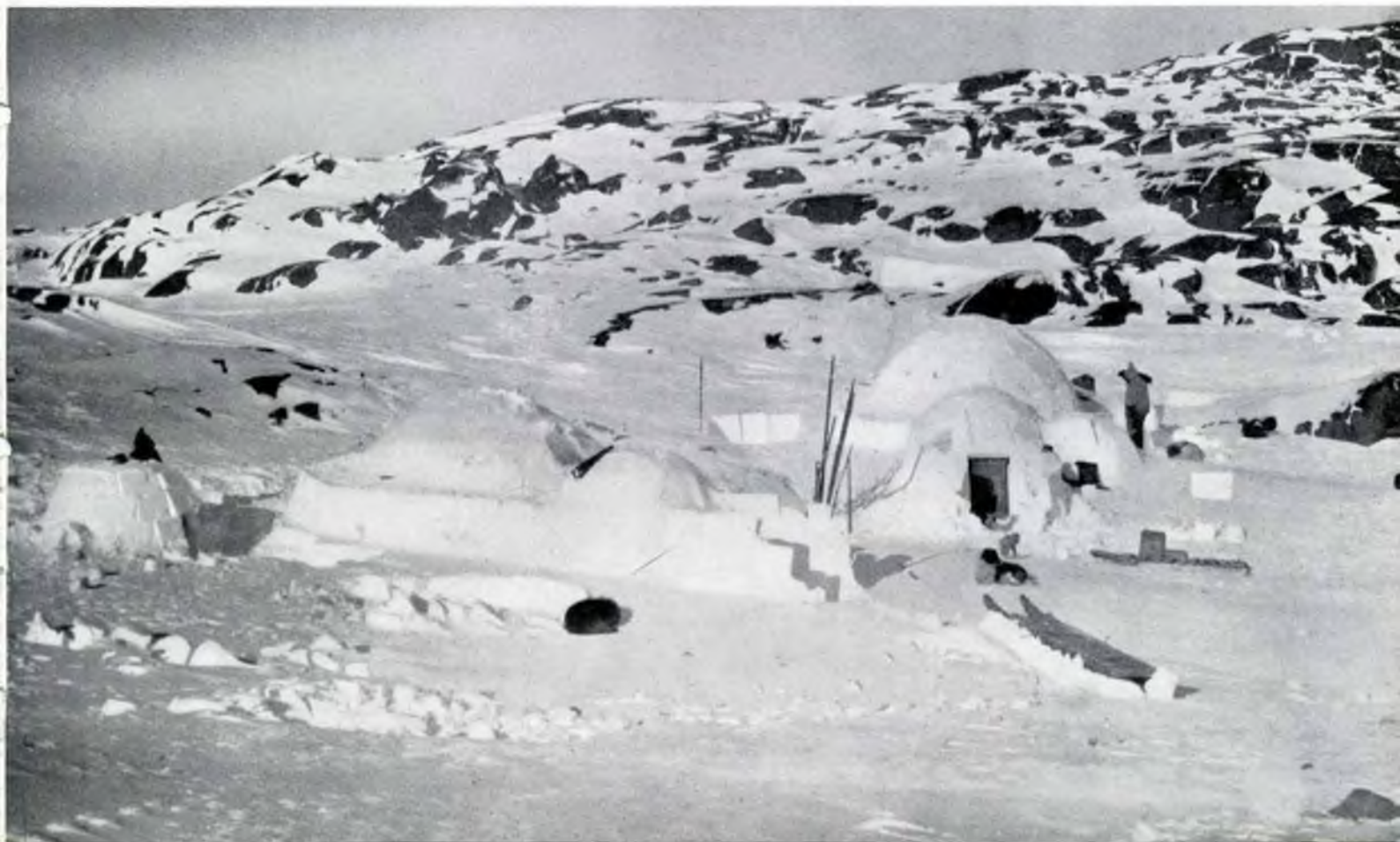
"Permanent" igloos, having a windbreak approach and a porch (with a store-room on the side) leading into the main living room with its raised floor. The window on the left hand house, near the saw, is of ice.
