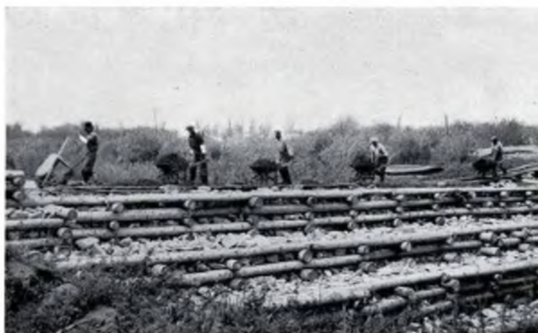
Dumping clay filling into Birch dam.
