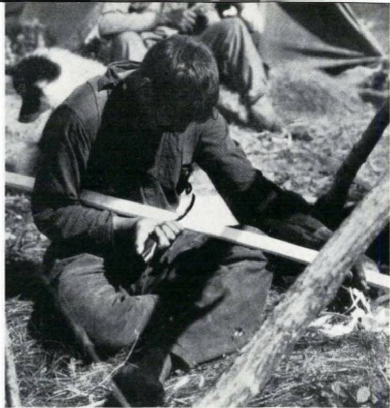
Making a snowshoe frame with a crooked knife. Natl. Mus. of Can.
