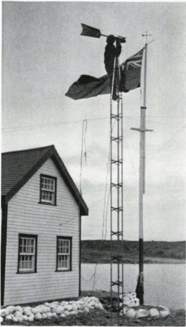
Erecting the Wincharger at Cape Smith, Hudson Bay.
