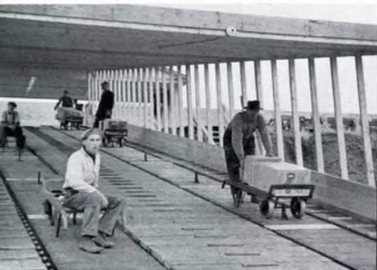
"Bull gang" on the conveyor.
