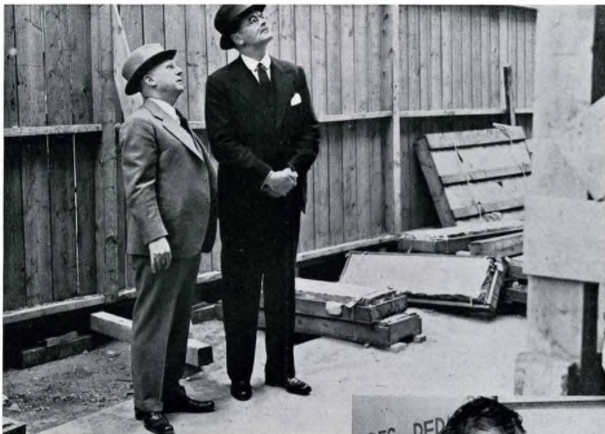
The Governor and A. H. Doe looking over the construction of the final section of the new Edmonton store.
