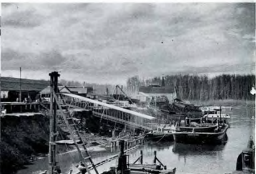
The busy waterfront—pile driver, conveyor and barges.
