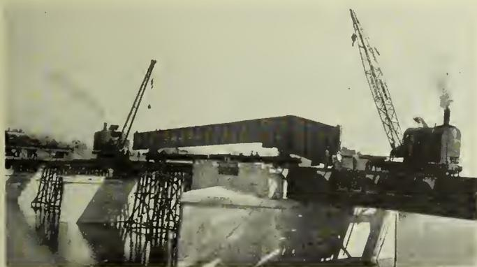
Fig. 16—Erection of Bascule Girder at Norwood.
