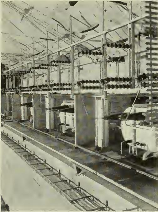
Fig. 2—Rapide Blanc Transformers and 220 kv. Disconnects.
