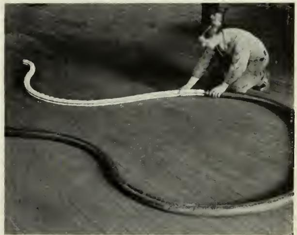
Fig. 3—Inserting Flexible Electric Heater in Curved Pipe Casing.
