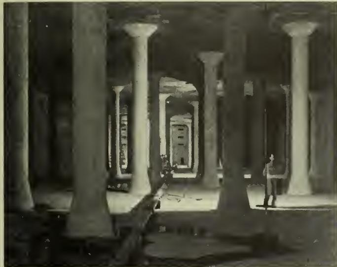
Fig. 14—Settling Basin Looking Towards Mixing Chambers.
