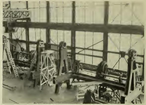
Fig. 15—Assembly of Machinery Girder and Bents.
