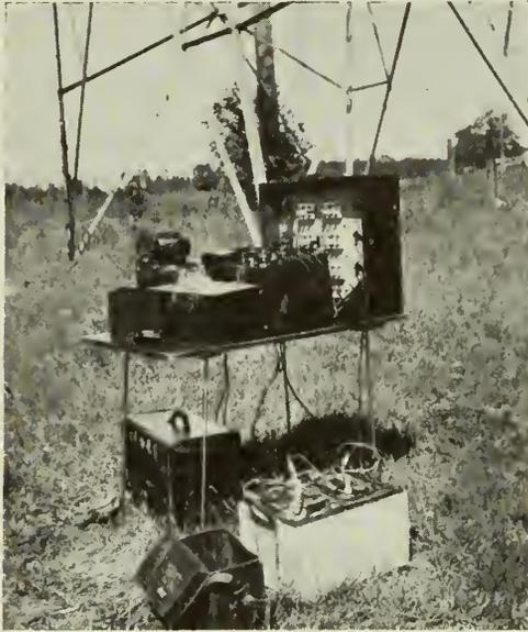
Fig. 7—Equipment for Studying Vibrations of Transmission Line Conductors.
