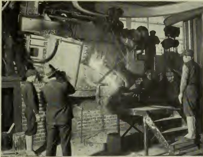
Fig. 2—Pouring from the Electric Furnace.
