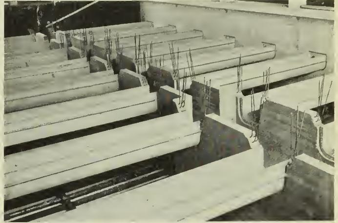
Fig. 11--Concrete Wash Water Troughs in Filter Unit.
