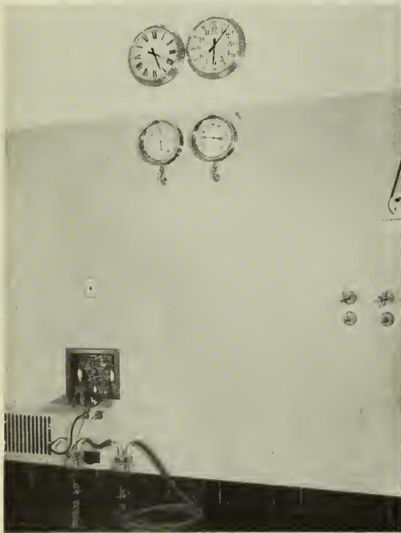
Fig. 7—Vacuum and Compressed Air Services and Electric Clocks in Operating Room.
