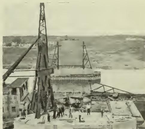
Fig. 18—Placing Trunnion Towers at Sorel.
