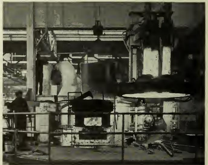
Fig. 1—Charging the Five-Ton Electric Furnace.
