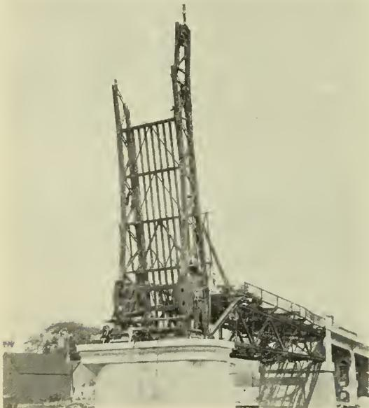
Fig. 20—Erecting Bascule Leaf at Sorel.
