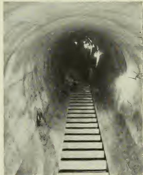
Fig. 8—Steps Forming Ramp in 7-Foot Tunnel.
