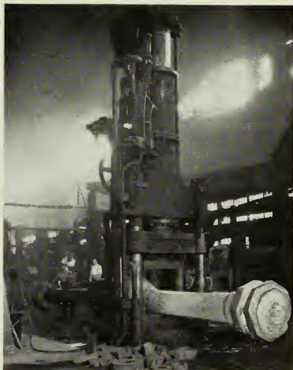
Fig. 1—Mine Hoist Drum Shaft Forging under 600-ton Hydraulic Press from 48-inch Ingot part Forged at this Point.
