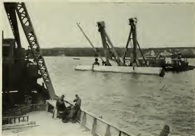
Fig. 5—Placing Intake Pipe, Diameter 96 inches.
