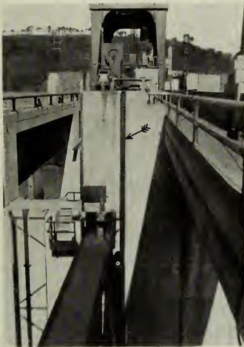
Fig. 2—Safe Harbour Dam with Heaters Installed in Masonry.
