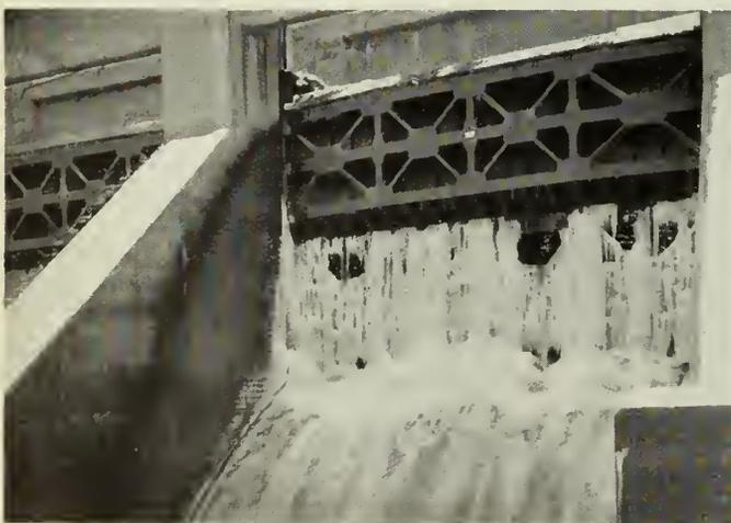
Fig. 1—Troublesome Ice Formations with Unheated Two-Leaf Gates.
