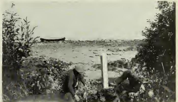
Fig. 1—Typical Surveyor's Post and Stone Mound.
