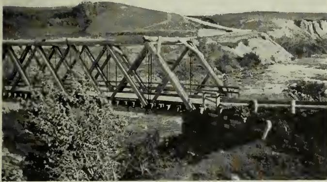
Fig. 4—Wooden Bridge Built of Untreated Timber.
