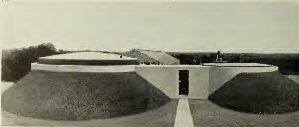
Fig. 6—Dorr Multidigester System. General view of Unit at Cedarhurst, L.I., with primary tank at right and secondary tank at left.
