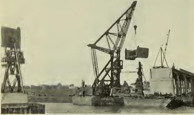
Fig. 19—Placing Trunnion Strut at Sorel.
