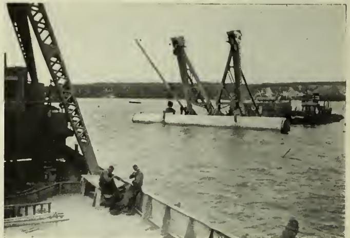
Fig. 5—Placing Intake Pipe, Diameter 96 inches.
