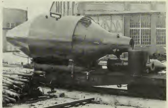
Fig. 11—Welded Salt Evaporator. Length 55 feet, weight 25 tons.
