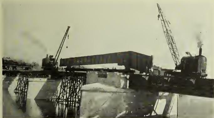
Fig. 16—Erection of Bascule Girder at Norwood.
