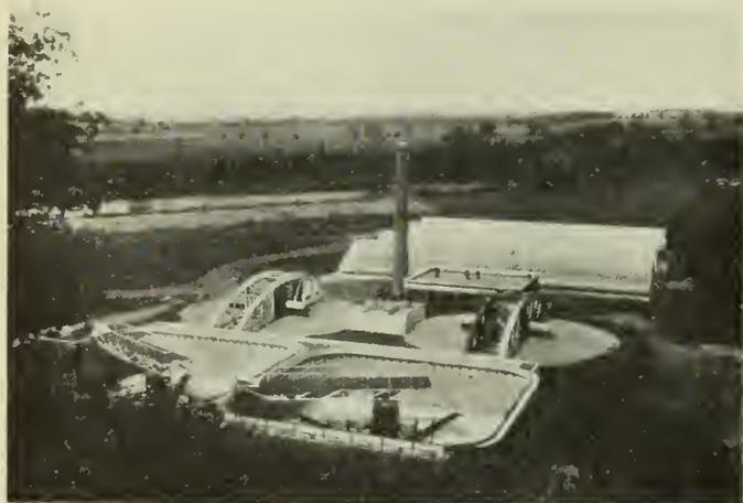
Fig. 1—Separate Sludge Digestion Plant 4 m.g.d., Kitchener, Ontario.
