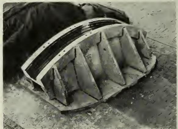
Fig. 9—Welded Cable Saddle for Isle of Orleans Bridge. Weight 3,000 pounds.
