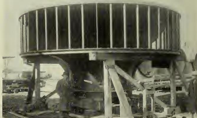
Fig. 6—Inlet to Intake Pipe, Diameter 20 feet.
