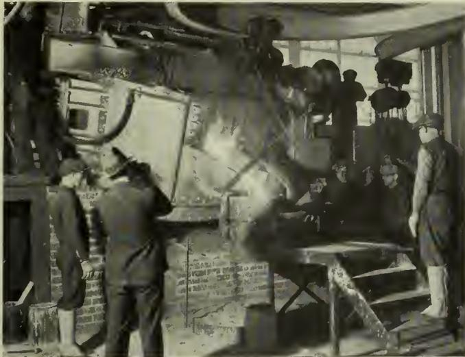
Fig. 2—Pouring from the Electric Furnace.
