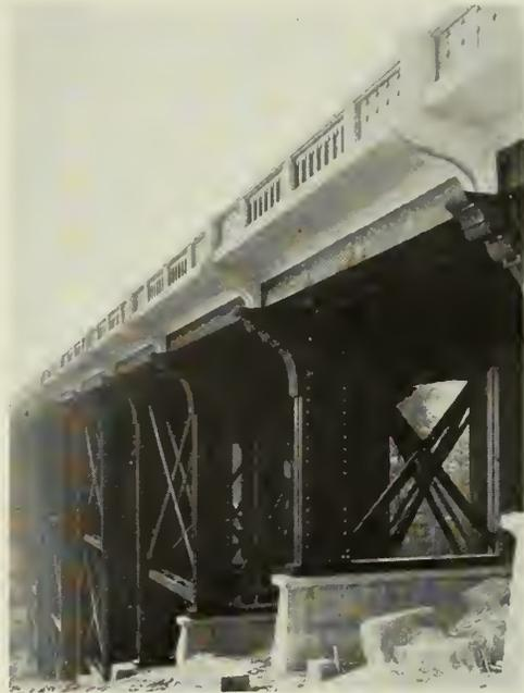
Fig. 7—Composite Type Bridge of Oregon State Highway Department.
