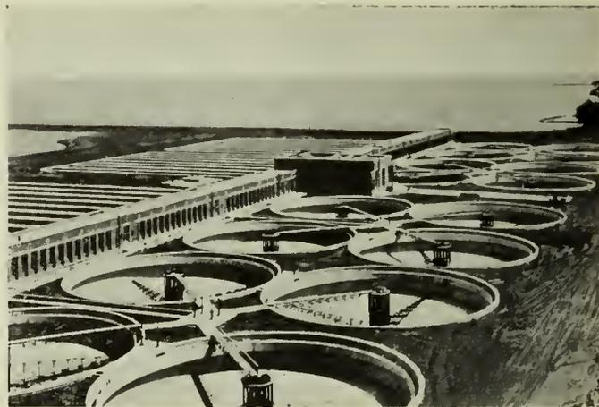
Fig. 4—Activated Sludge Plant for 123 m.g.d., Cleveland, Ohio.
