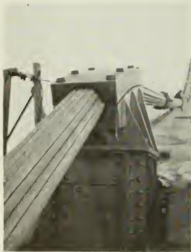
Fig. 10—Cable Bent Saddle.
