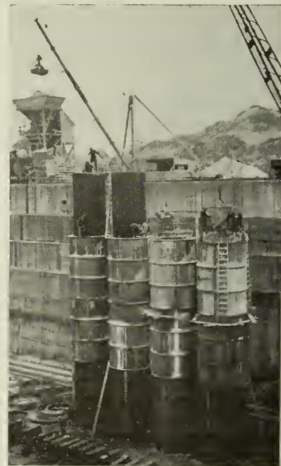
Fig. 5—Cylinder Casting.
