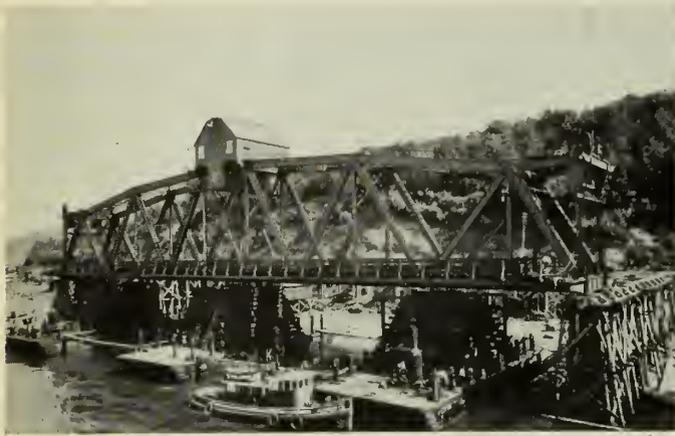
Fig. 22—Scows in Place under Lifting Span.
