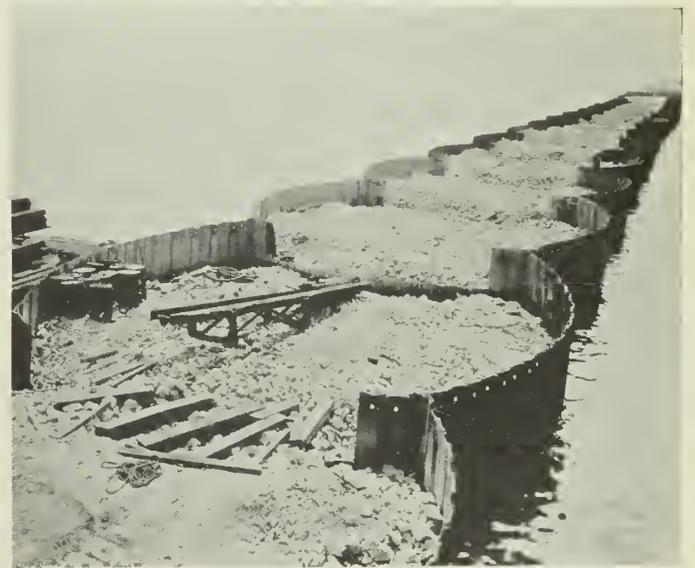
Fig. 6—Cellular Sheet Pile Breakwater, Calumet Harbour.
