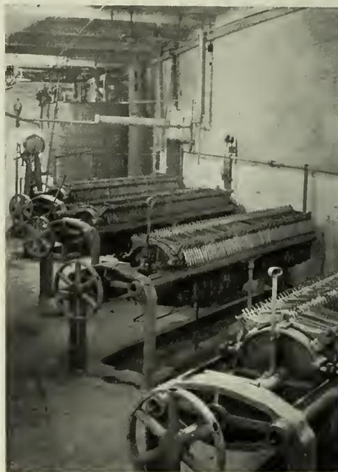
Fig. 3—Filter Presses.
