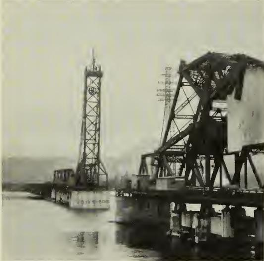
Fig. 13—Hoisting Sheave on North Tower.
