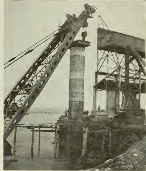
Fig. 7—Cylinder Setting.
