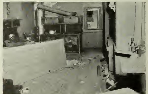
Fig. 4—Effect of Explosion in Basement of Convent.
