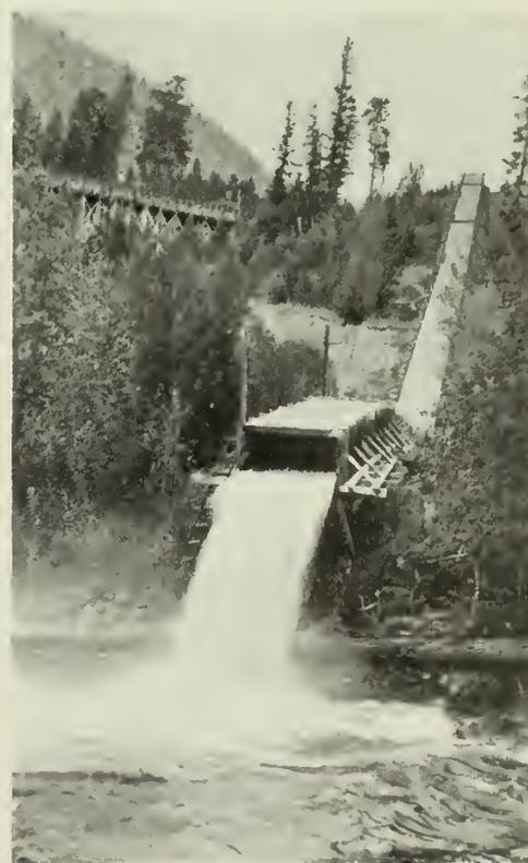
Fig. 3—Flume Wasteway discharging into Barriere River.
