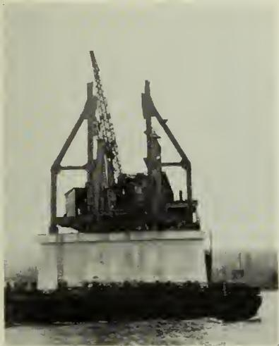
Fig. 19—Erecting Lower Sections of North Tower.
