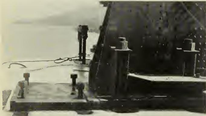
Fig. 18—Bed Plates and Anchor-Bolts on Pier 2B after Vibration.
