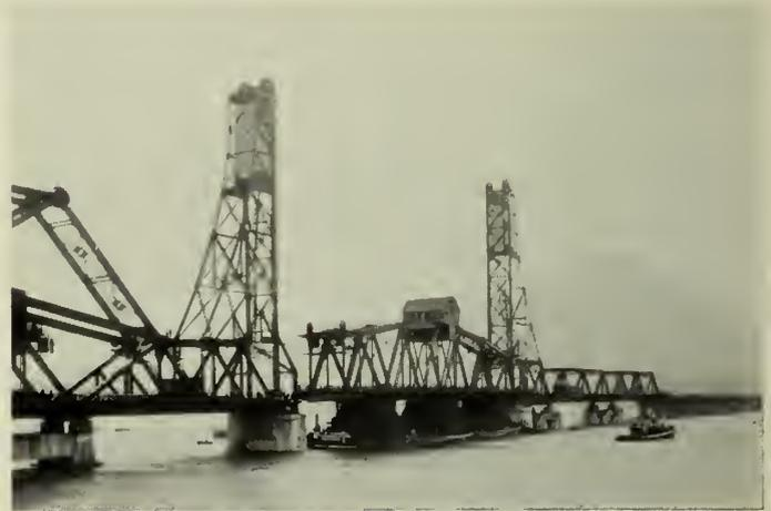
Fig. 23—Lifting Span Approaching Final Position.
