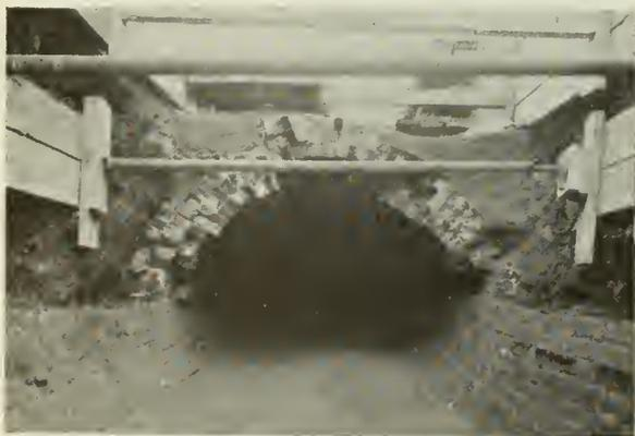
Fig. 6—Effect of Gasoline Explosion on 6-foot diameter Brick Sewer.
