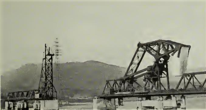
Fig. 20—Erecting North Tower by "Creeper."
