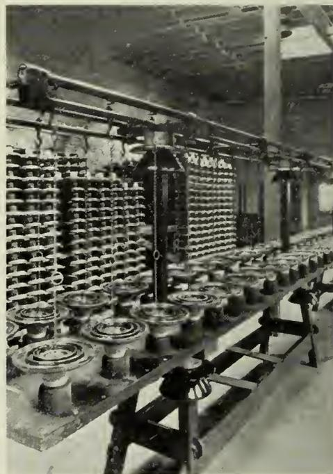
Fig. 13—Pan Test of Unassembled Shells.
