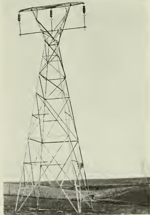
Fig. 5—Steel Tower on Clinton Dubuque 66-kv. Line.
