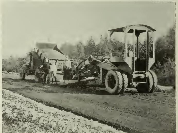
Fig. 5—Laying Bituminous Paving near McKinleys Corner, Lower Onslow.
