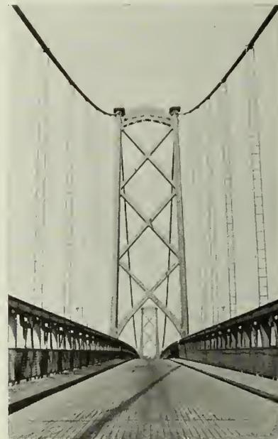
Fig. 12—View of Trusses, Floor Grids, Kerbs and Fences.
