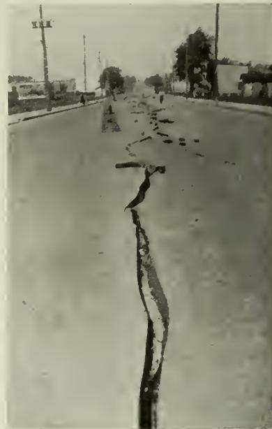
Fig. 7—St. Lawrence Blvd., Montreal, after Explosion in Sewer.
