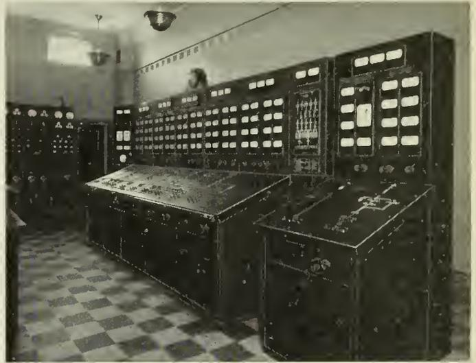
Fig. 13—Control Desk and Metering Board in the Control Room.
