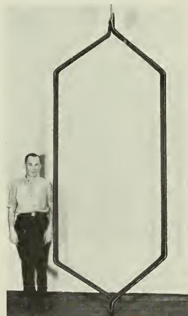
Fig. 5—Stator Coil of the 25-Cycle Motor.
