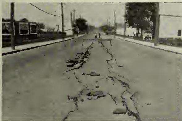
Fig. 8—Street Pavement over Sewer after an Explosion.
