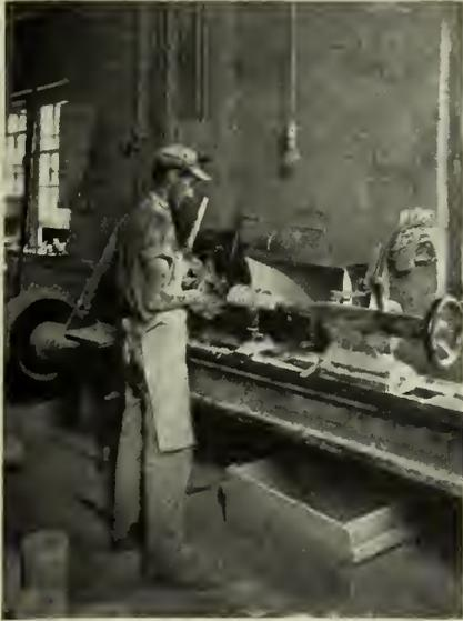
Fig. 9—Operator Turning Transformer Bushing.
