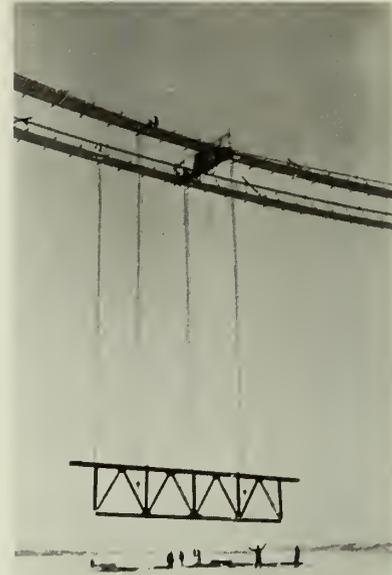
Fig. 11—Erection of First Truss Section.
