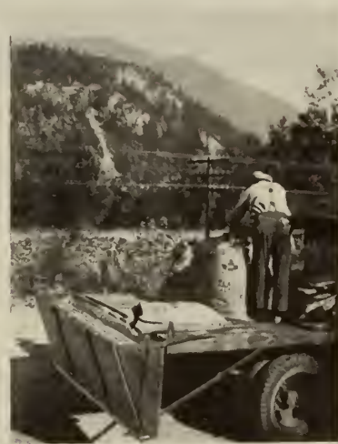
Fig. 6—Method used for spreading calcium chloride.
