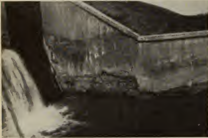
Fig. 1—Typical case of disintegration. Soil strongly alkaline.
