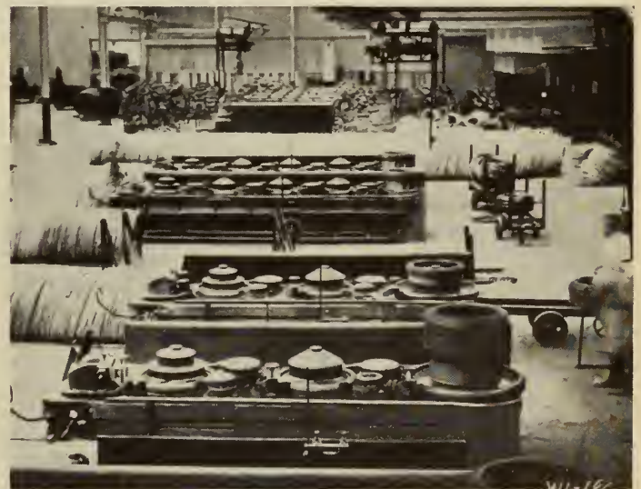
Fig. 3—Modern continuous rod frame
