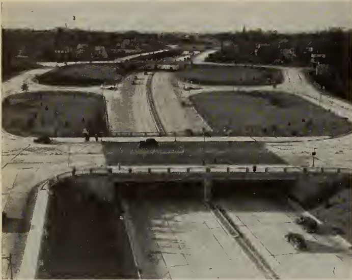
Fig. 3—Entrance to the George Washington Bridge, State of New Jersey
