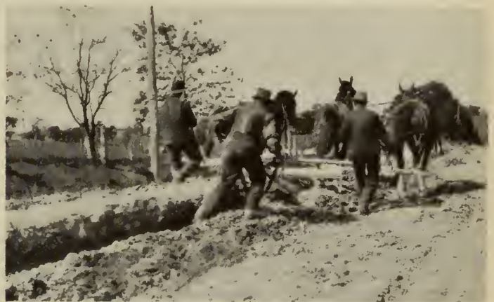
Fig. 6—Highway Work in Ontario, 1918. Ditching Operations
