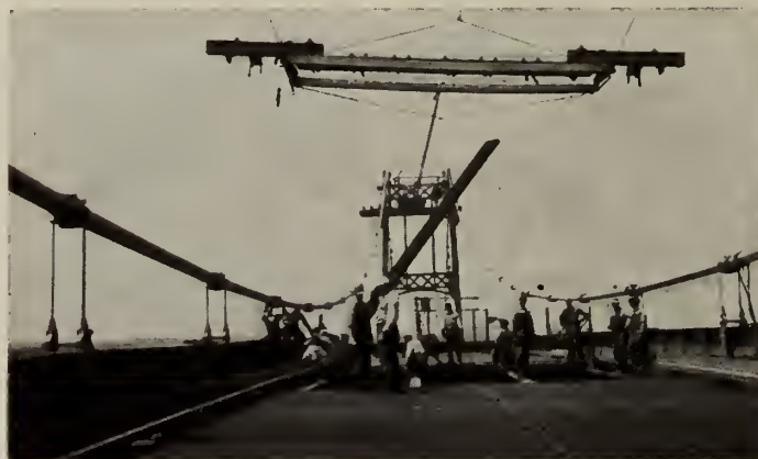
Fig. 10—Erecting I-Beam-Lok Flooring, Suspension Bridge
