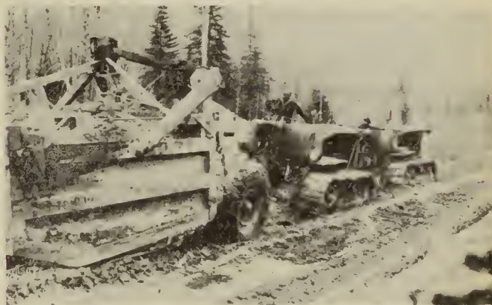
Fig. 10—Highway Work in Ontario, 1938. Grading with Carryall
