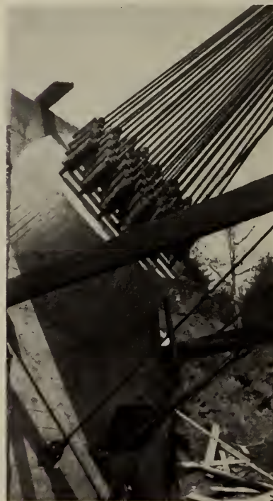
Fig. 7—Anchorage Assembly
