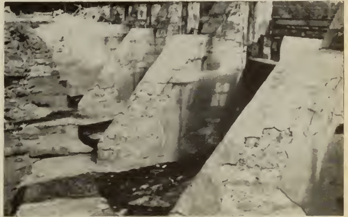
Fig. 2—Showing the deterioration that had taken place in unreinforced gunite placed on the piers of Almaville Dam in 1924. Dam built in 1910
