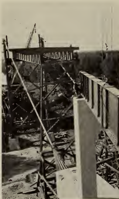
Fig. 6—Erection of North Approach Viaduct Suspension Span
