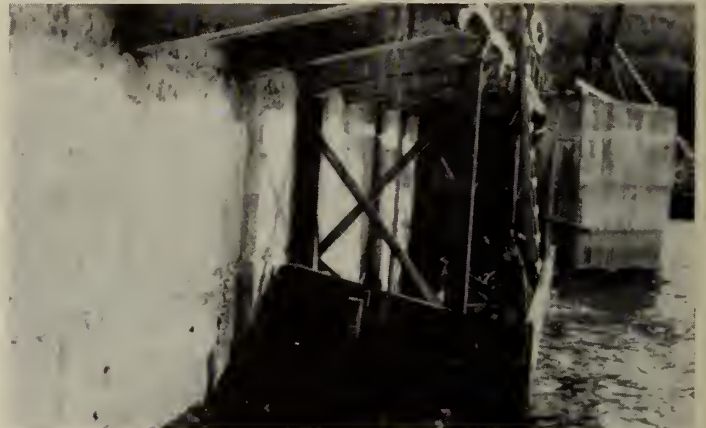
Fig. 5—Moving caisson being used on repairs to Gouin Dam shows the caisson in position against the upstream face of the dam. This dam was built in 1918
