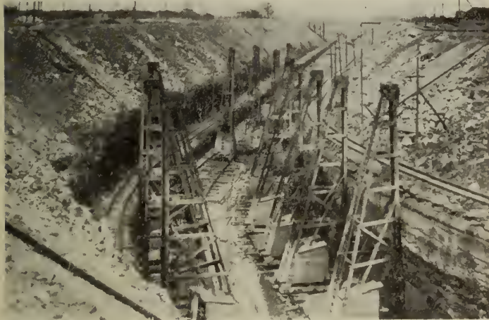
Fig. 1—Queenston-Chippewa development, 1918 to 1922. Battery of Drills working in Rock Cut
