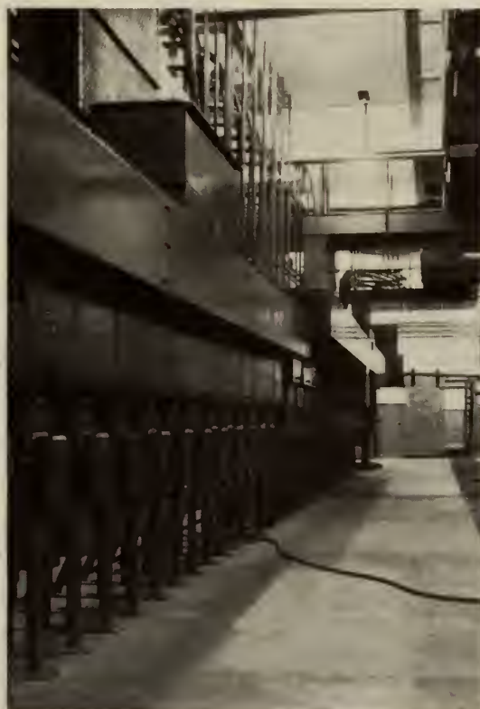
Fig. 8—Metal Clad Switchgear at Substation
