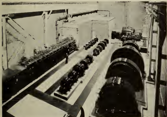
Fig. 3—Motor room for reversing mill shown in Fig. 2. The 7,500 kw. flywheel motor generator set in the right foreground, furnishes direct current power for the 7,000 hp., 700 volt, 40/100 r.p.m. reversing mill motor.
