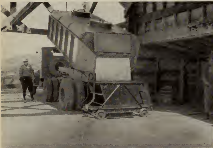
Fig. 3—Rapide Blanc Development, 1931 to 1934. Unloading cement from special semi-trailer truck into bin at mixer plant
