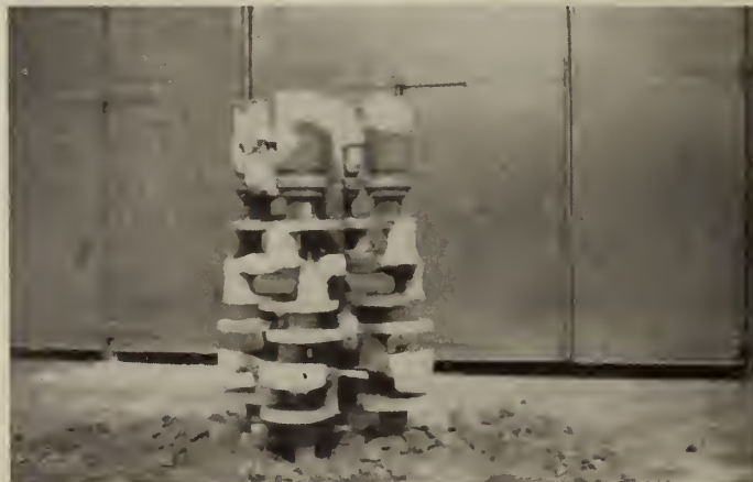
Fig. 1—Crankshaft Cluster
