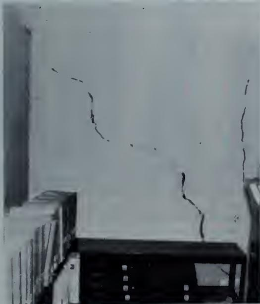
Fig. 1—Cracked wall in the library on the ground floor.
