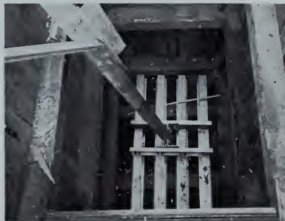
Fig. 3—Steel underground in grillage tower base.
