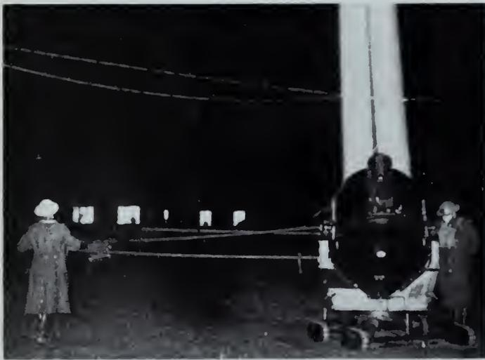
The projector has a long arm at the end of which is a wheel so that bearing and elevation are controllable.
