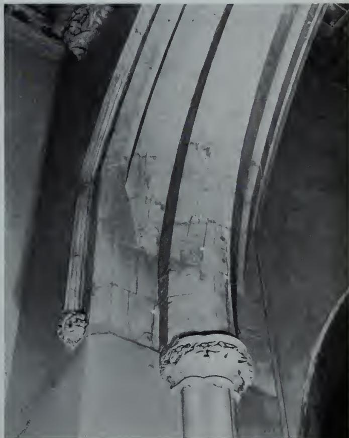
Fig. 1—One of the tower arches. This view shows some of the damage caused by settlement before the original spire was completed.
