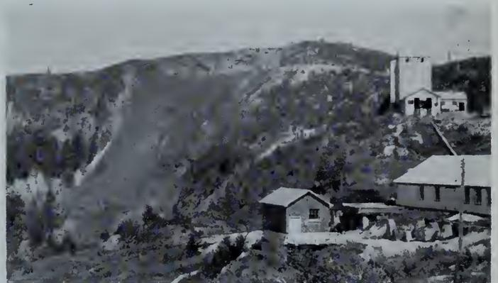
Fig. 1—Helen open pit at top of hill and aerial tram loading plant and bin.
