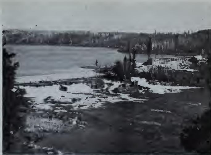
Fig. 3—Rock fill dam in process of construction on Bluefish Lake, as part of the Prosperous Lake water power development.
