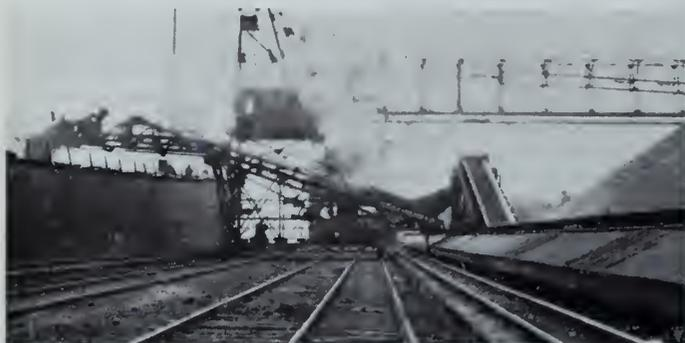
Fig. 6—Algoma Central Railway gantry transferring ore from dock belt to ship.
