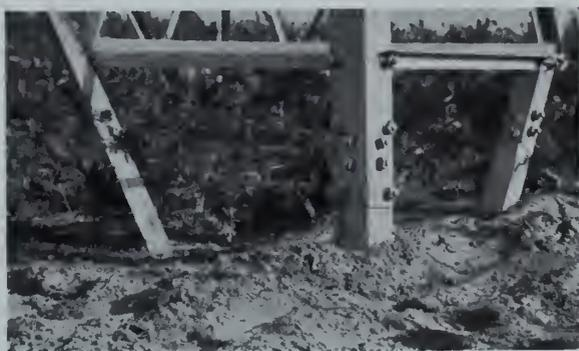
Fig. 4—Steel above ground in grillage tower base.
