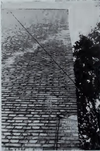
Fig. 3—Rear wall of building, showing the amount of movement previous to underpinning.
