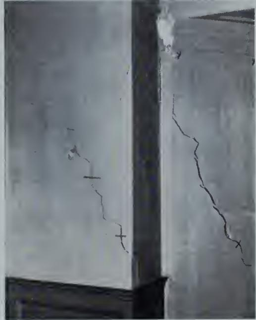
Fig. 2—Southwest corner of auditorium on the second floor, showing damage to plaster partition.
