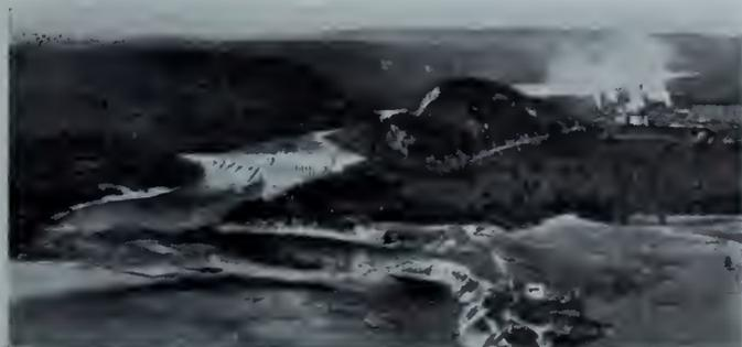
Fig. 15—Aerial view of La Tuque dam showing the two granite knobs and the sand-floored valley to the east (right) under which the pre-glacial valley is buried.
