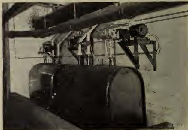
Fig. 6—Fuel oil reservoir and pumps.
