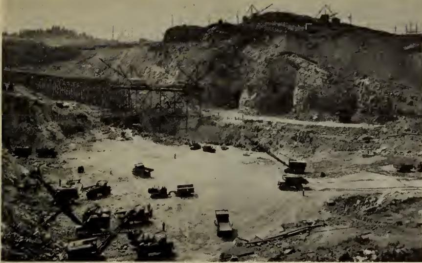
Fig. 6—Tailrace excavation and tunnel portal excavation in the background.
