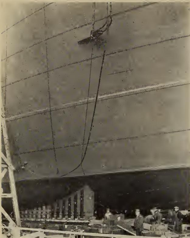
Fig. 11—View of bow of vessel showing starboard fore poppet and connection of drag cable to hull.
