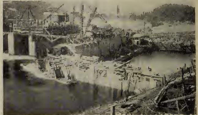
Fig. 16—Second-stage cofferdam cribs in place, looking downstream.
