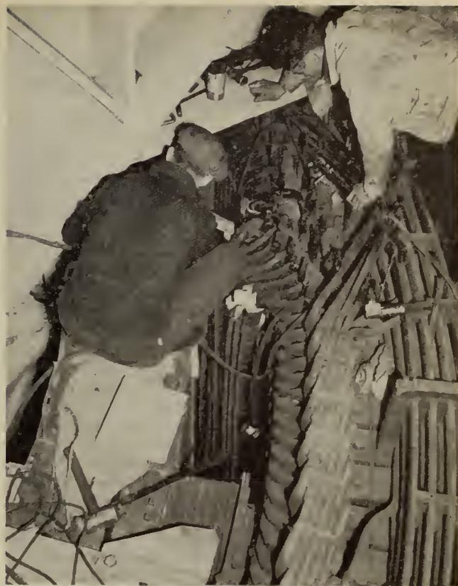
Fig. 8—Interior of the generator showing the replacement of a stator coil.
