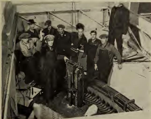
Fig. 7—Interior of the generator showing how a pole may be removed after the hatch covers are lifted off.
