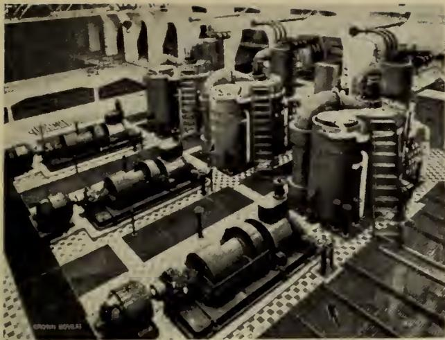
Fig. 2—Three Velox steam generators each for 34.5t/h of steam, with gas turbine driven compressor erected in front of each boiler, at Haifa power plant.
