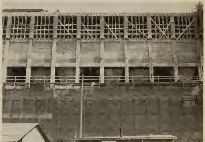
Fig. 8—Coal bunker wall and hoppers.
