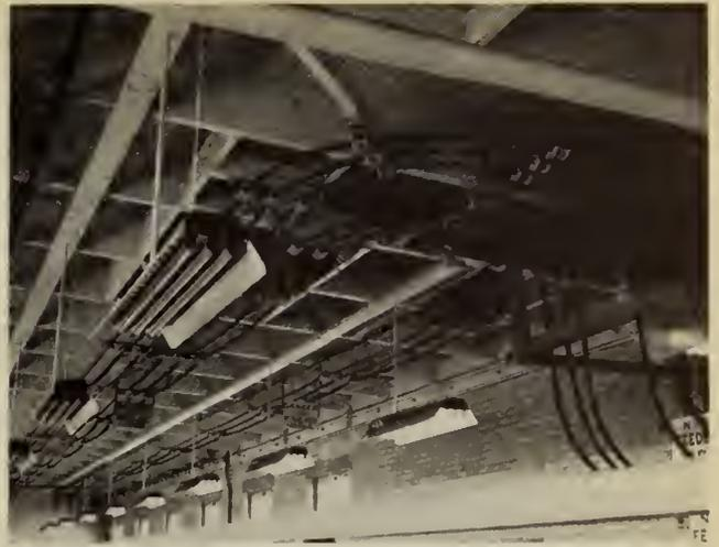
Fig. 2—550 volt feeders in large punchpress building.
