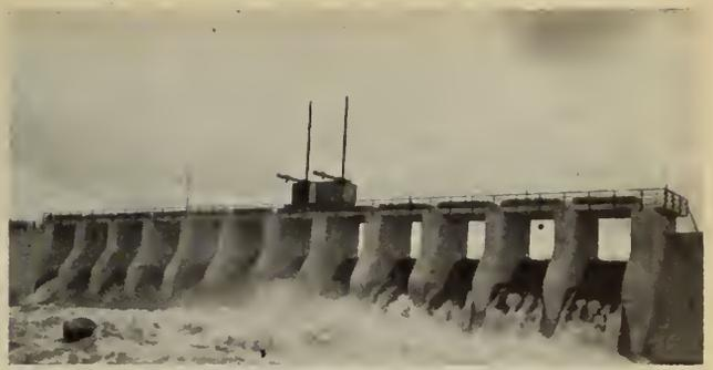
Fig. 4—Waboose dam sluiceways discharging about 6,000 cu. ft. per sec.
