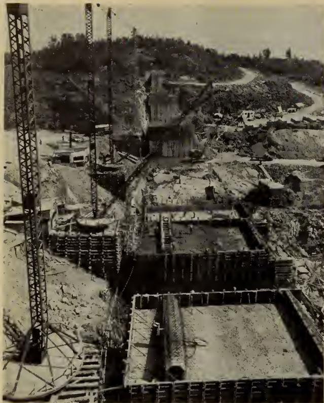
Fig. 11—Pouring concrete at dam No. 3B.
