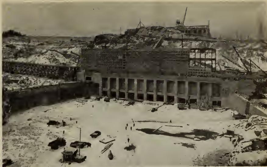
Fig. 10—Looking northwest toward downstream face of powerhouse and tailrace cofferdam from east side of plug.
