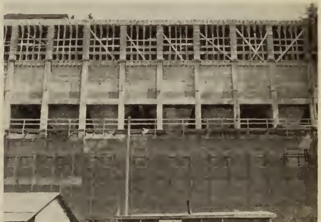
Fig. 8—Coal bunker wall and hoppers.
