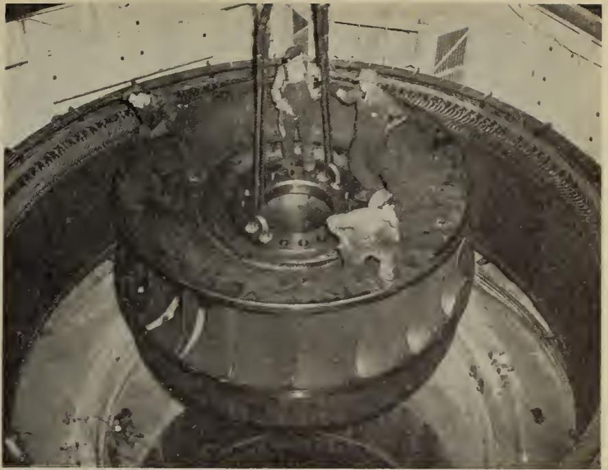
Fig. 5—Lowering the turbine runner into place.
