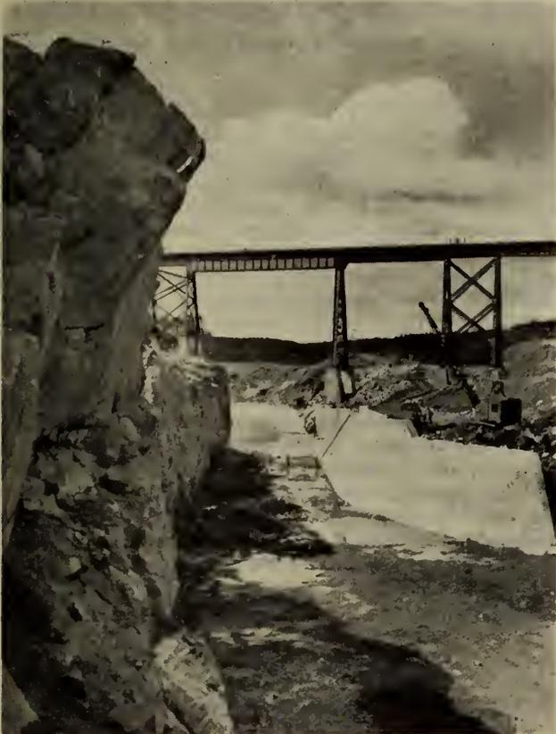
Fig. 7—View of rock cut under new C.N.R. bridge and showing concrete training wall.
