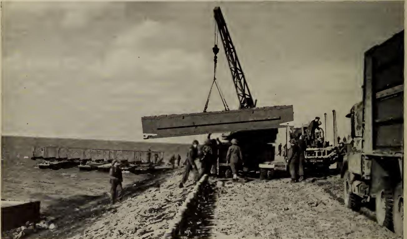
Army crane swings pontoon out into the water as Royal Canadian Engineers prepare for an embarkation across the Scheldt. Operations later included many types of vehicles and smoke screen equipment (Canadian Army Overseas Photo.)
