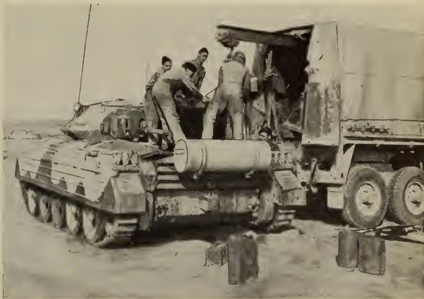
Removing the radiator from a Crusader Tank with the aid of a Break-down Lorry.
