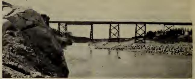
Fig. 6—View showing Jackfish river new channel and bridge. Flow about 2,500 cu. ft. per sec. Note rock covering on right bank.
