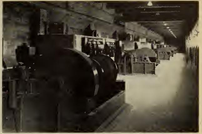
Fig. 15—70-ton hoists for operating intake gates.
