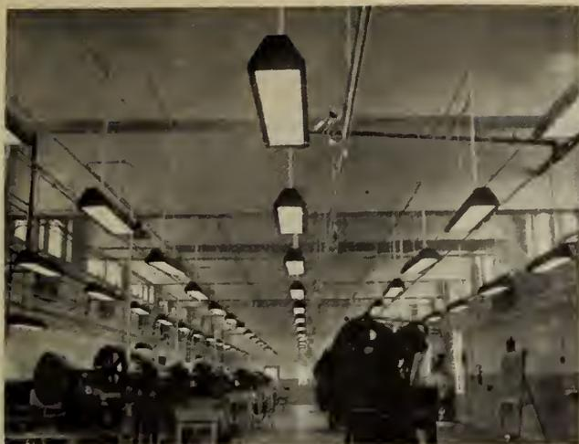
Fig. 8—Special dust-tight fluorescent lighting fixtures.
