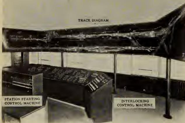
Fig. 2—Interlocking control machine
