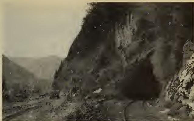
Fig. 7—Railway has tunneled through rock bluff, while highway is built around it. Section 3.
