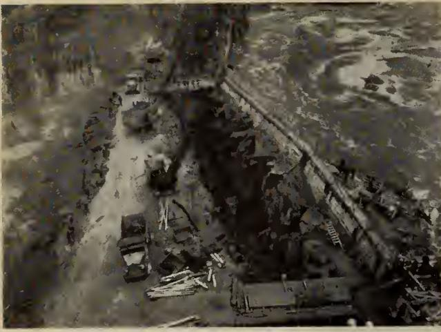
Fig. 8—Excavation of trench behind tailrace rock plug.
