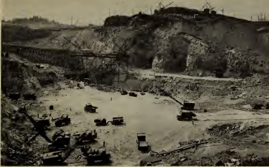
Fig. 6—Tailrace excavation and tunnel portal excavation in the background.
