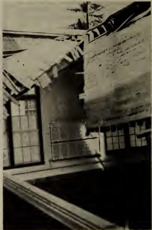
**Broken roof of girls' gymnasium in Cornwall High School caused by collapse of parapet above.**
