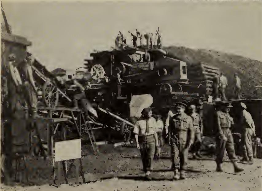
The rock crusher outfit shown at the left is operated by Royal Canadian Engineers in Colombelles, France. It provides surface materials for rebuilding damaged roads, necessary for the traffic of heavy equipment to the front.
