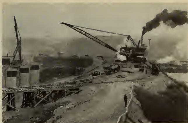
Fig. 3—Removal of temporary earthfill dam upstream from the control works.
