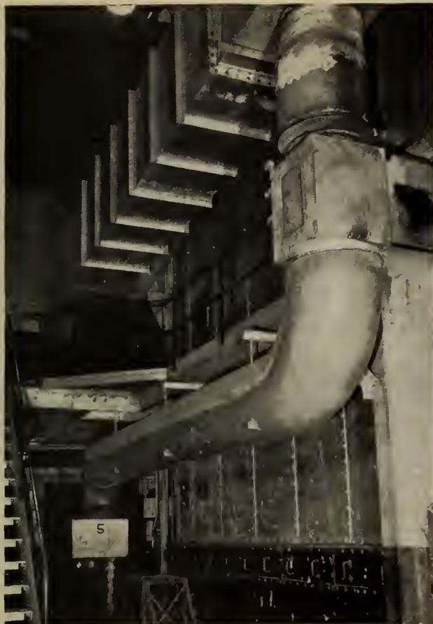
Fig. 4—Auxiliary hot air duct to pulverizer.
