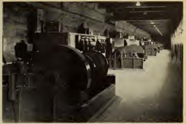
Fig. 15—70-ton hoists for operating intake gates.
