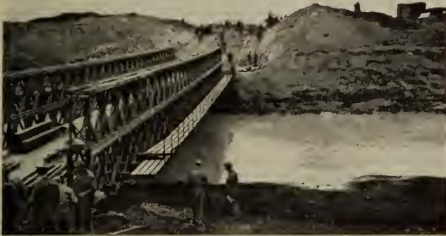
Double-truss, double-storey type of Bailey bridge, with footway.
