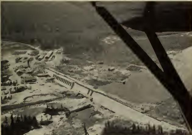
Fig. 3—Aerial view of Waboose dam before closure. Ogoki river flow passing through two openings in spillwall and down channel beyond island. Note cofferdam extending upstream from island.
