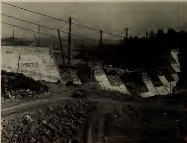
Fig. 12—Dam No. 3B, illustrating the method of pouring concrete in vertical lifts and alternate blocks.
