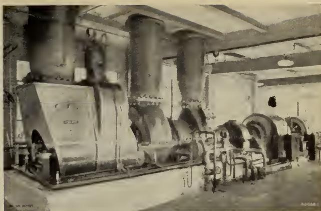
Fig. 7—Gas turbine supercharging plant for the Houdry oil refining process at Marcus Hook, Philadelphia.
