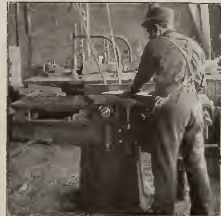
Wing Guard for Jointer
