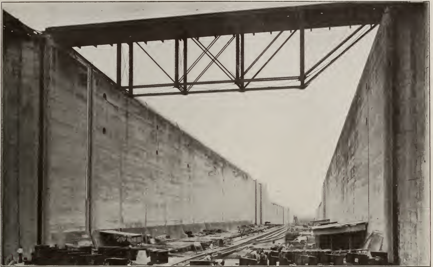
Gatun Upper Locks, East Chamber, Looking north. Beginning Construction of Intermediate Gates.
