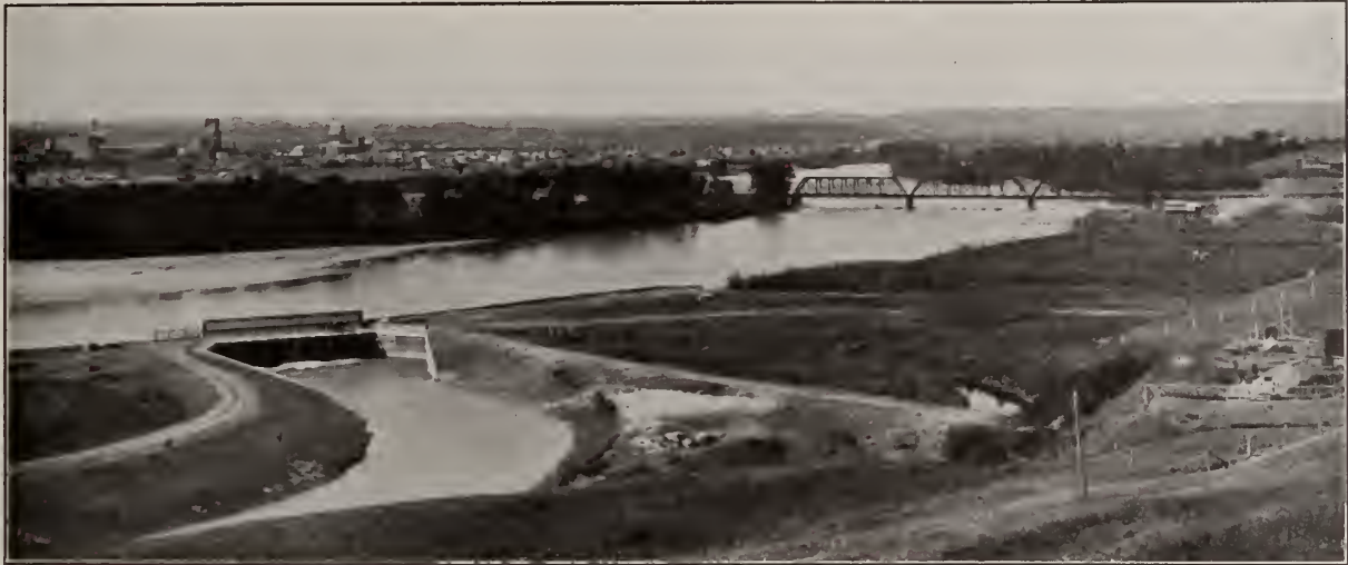
Headgates and Main Canal on C.P.R. Irrigation System.
