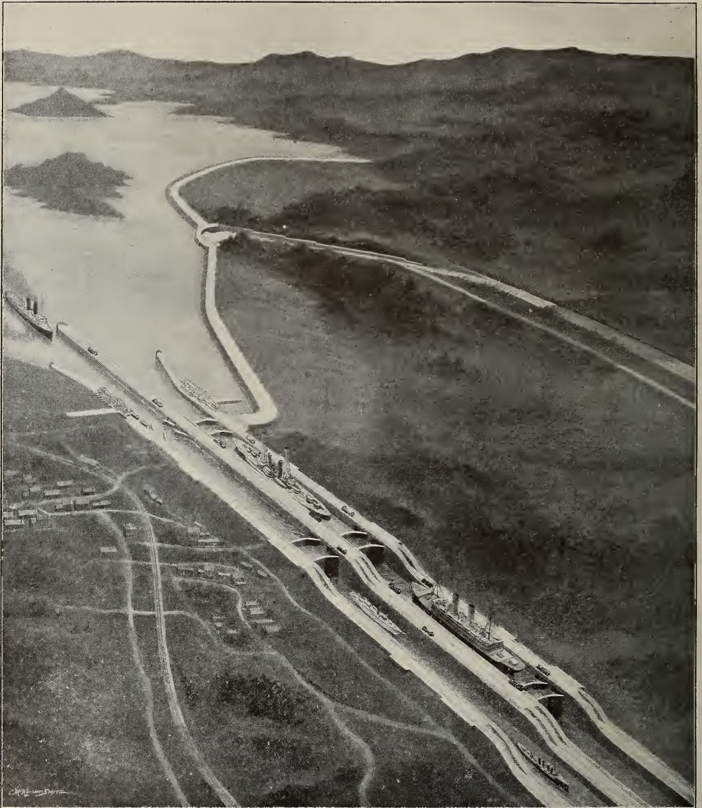
The view shows a section of the Atlantic division of the Panama Canal as it will appear when completed. In the foreground are the Gatun locks, which lie six miles from the Atlantic shore line. The Gatun dam and Gatun Lake appear in the background. Ships will not pass through the locks under their own power, but will be towed by four electric locomotives, running on tracks upon the side of the centre walls.— From Scientific American.
