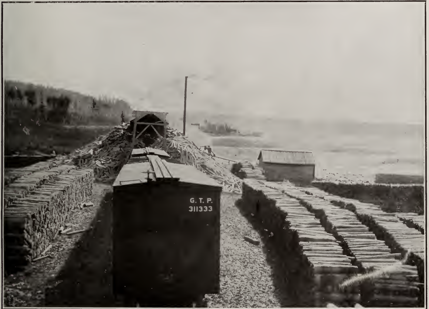
Lumber Mills and Yard, Northern Ontario.
