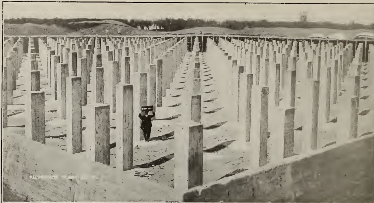
Filter, Masonry Complete, Except Roof.
