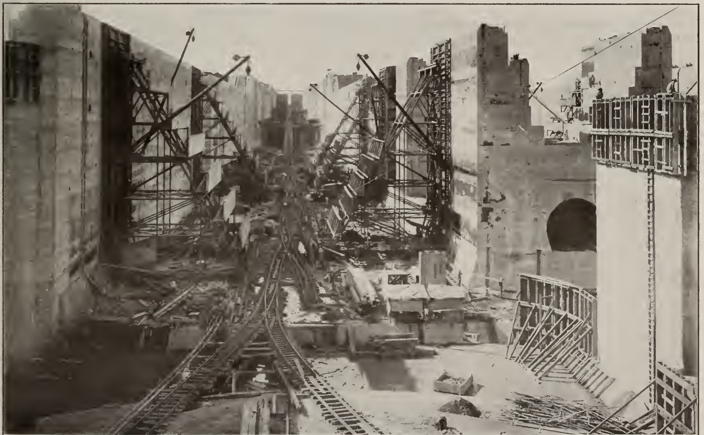
Gatun Lower Locks, East Chamber, Looking South From Cofferdam, Middle and Upper Locks in Distance.
