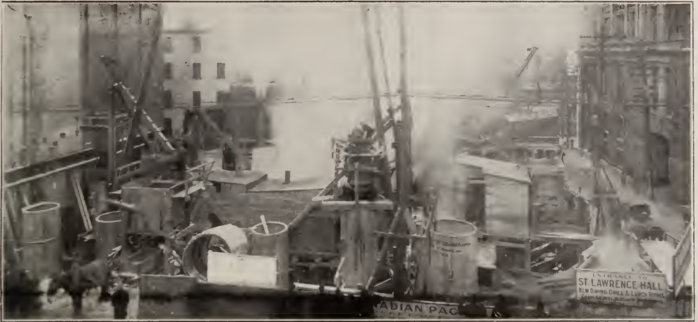
Building up Concrete Piers Above Ground and Sinking Them Down to Rock by Undermining.
