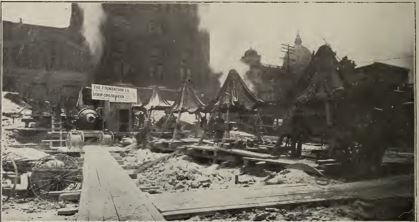
Carrying the Piers of the C.P.R. Windsor Station, Montreal, to Rock by the "Open Method."
