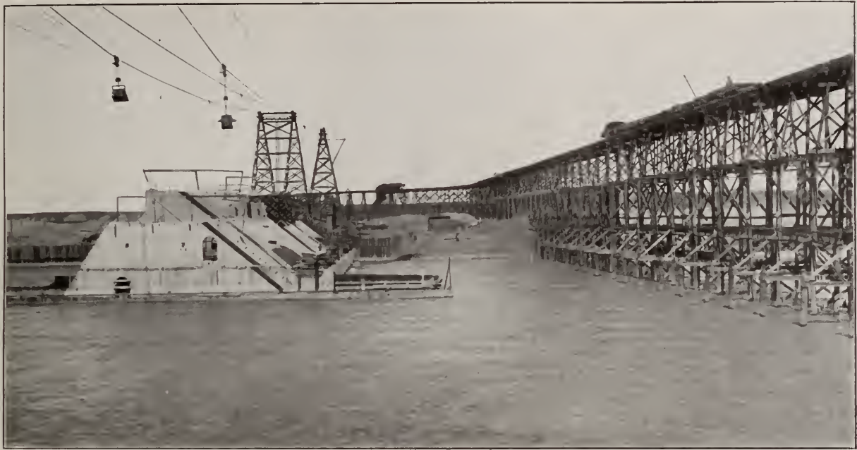
Trestle Work for Dam on Irrigation System. The Key of the Canals.
