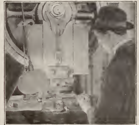
Individual Light for Punch Press
