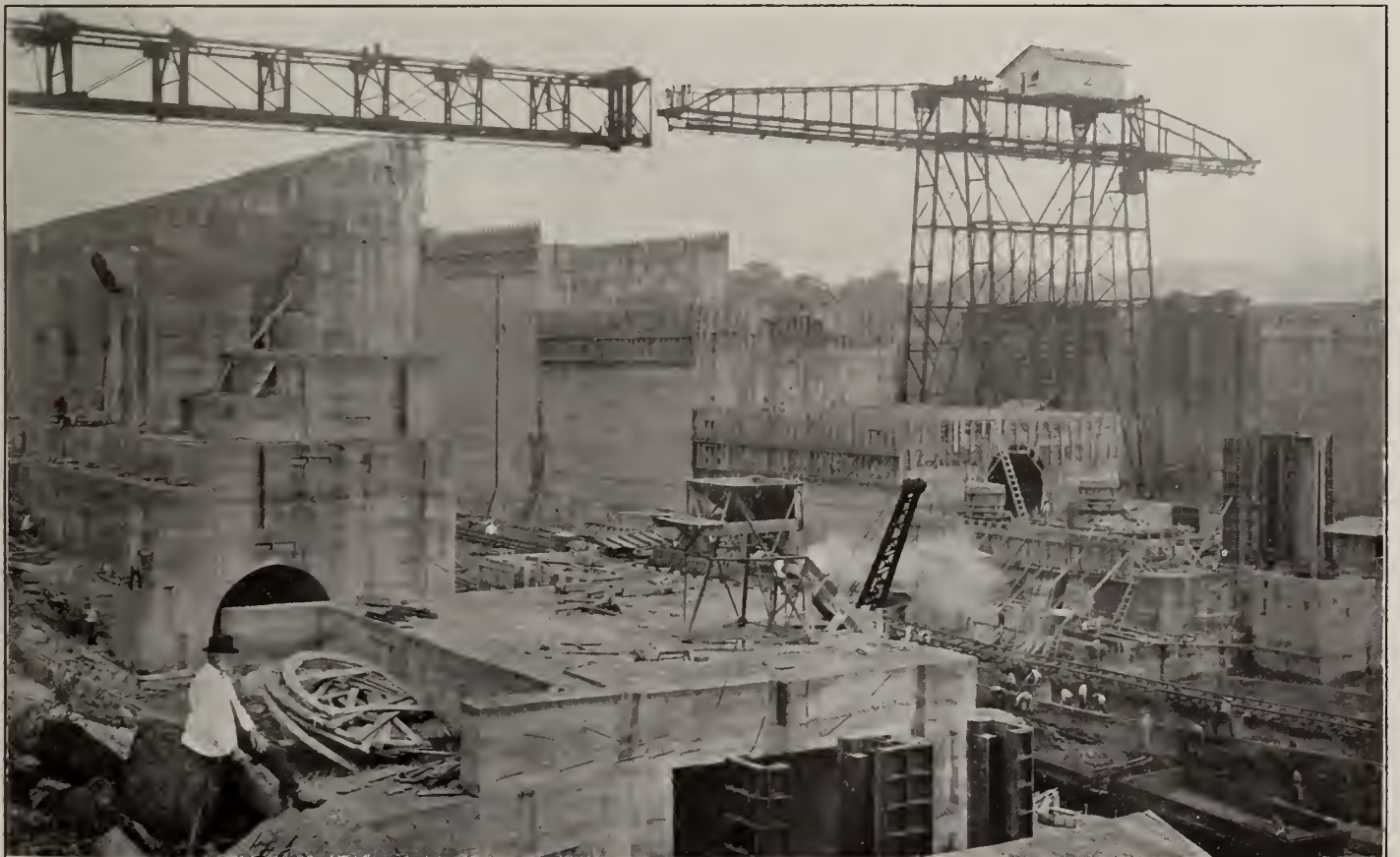
Miraflores Upper Locks, South End of West Chamber, Showing Stoney Gate Valve Frame in Position in West Wall
