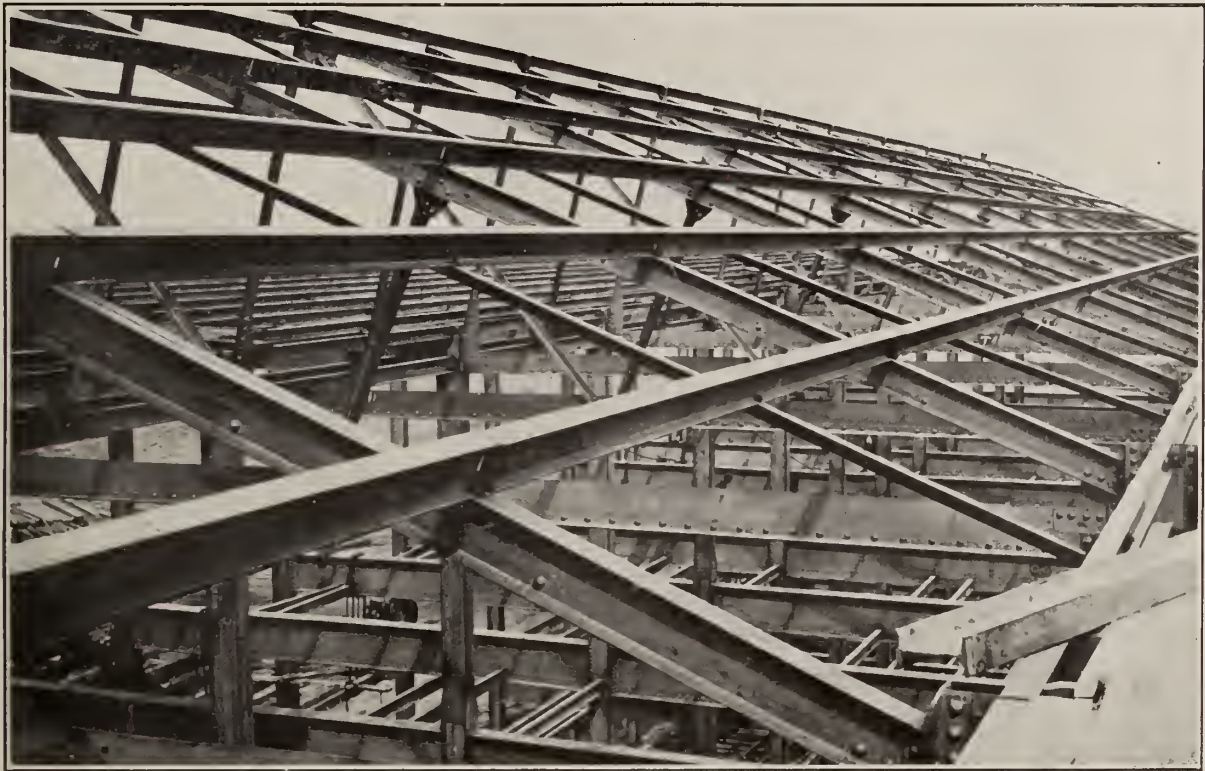
Structural Steel of Roof in New Oliver Factory in Hamilton.
