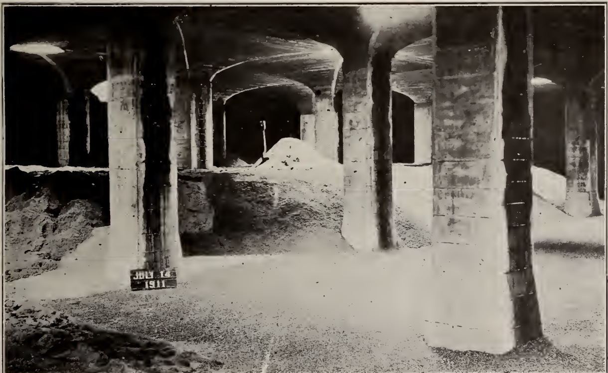
Placing Filter Material in Completed Filter.
