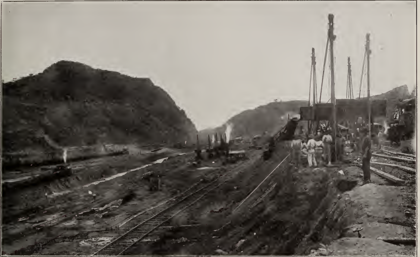
Culebra Cut, Looking South, Showing Well or Churn Drills.
