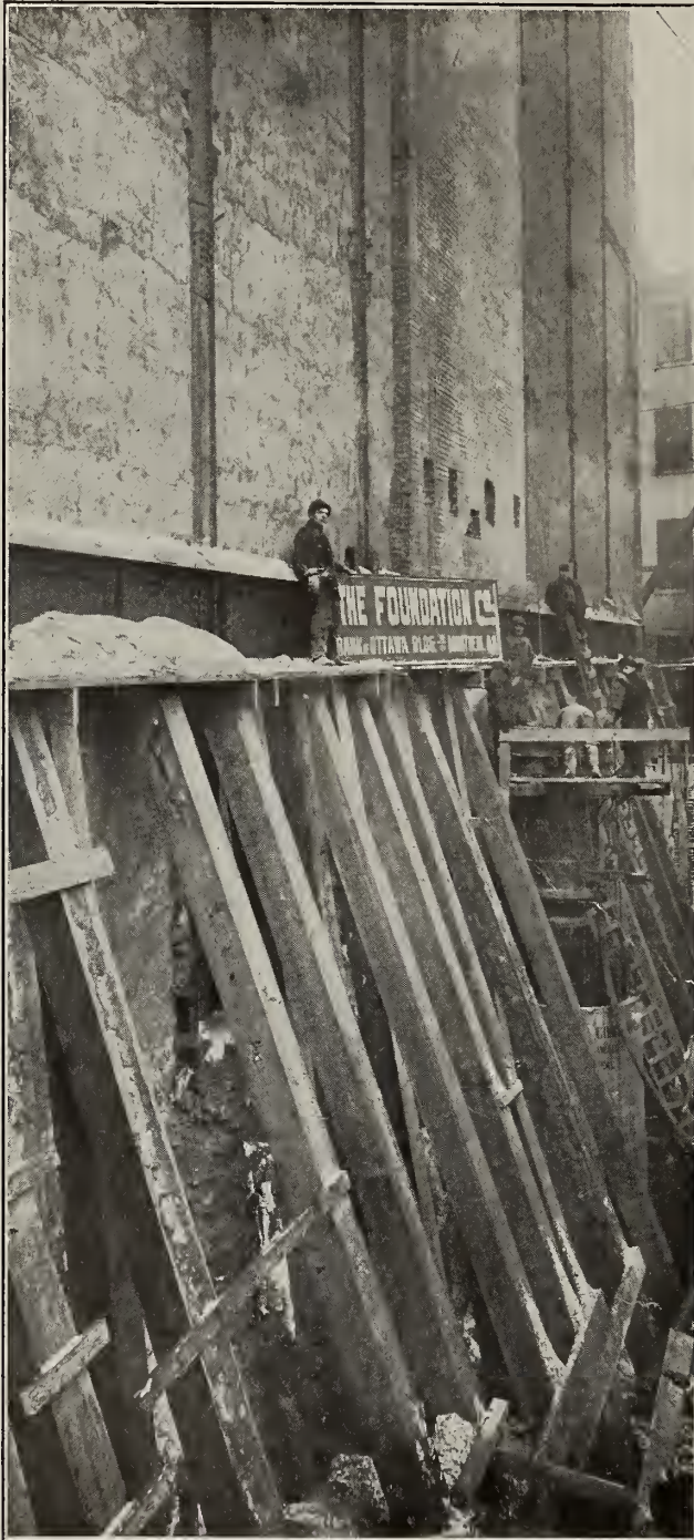
Bracing an Adjacent Wall While the Foundations of a Tall Building are Being Driven Down to Rock.
