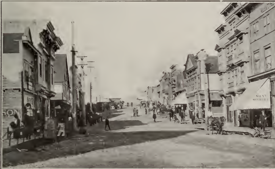
Prince Rupert—Third Avenue West.
