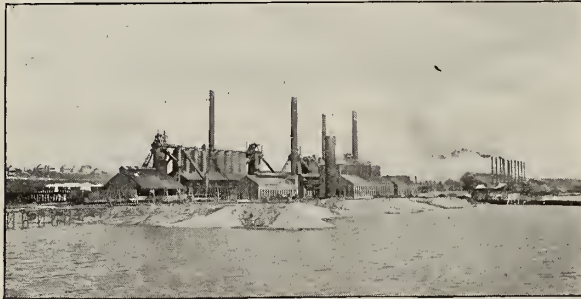
A Steel Plant Down by the Sea.
