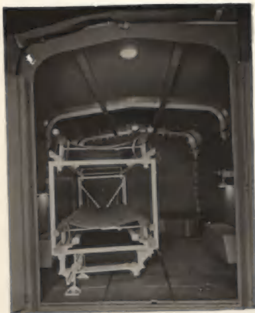
REAR INTERIOR VIEW (SHOWING STRETCHER ENDS RAISED TO LEVEL OF VEHICLE TOP LOADING)
