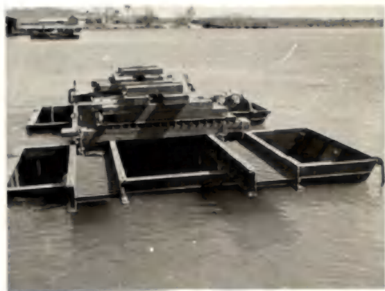
TWO PONTONS JOINED TO FORM A RAFT. SHOWN WITH ROADBEARERS IN PLACE PLUS 24000# OF PIG LEAD
