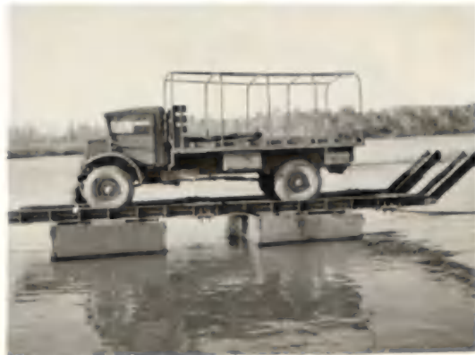
3 TON 4X4, 159" W.B. C.M.F. TRUCK ON TWO PONTON RAFT.
