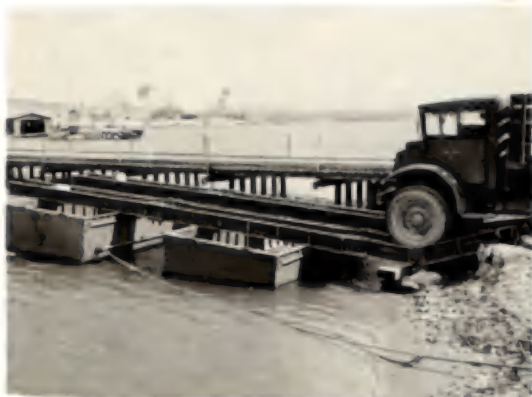
METHOD OF LOADING TRUCK ON TWO PONTON RAFT.
