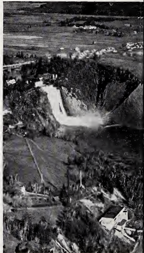
Addition Completed to
