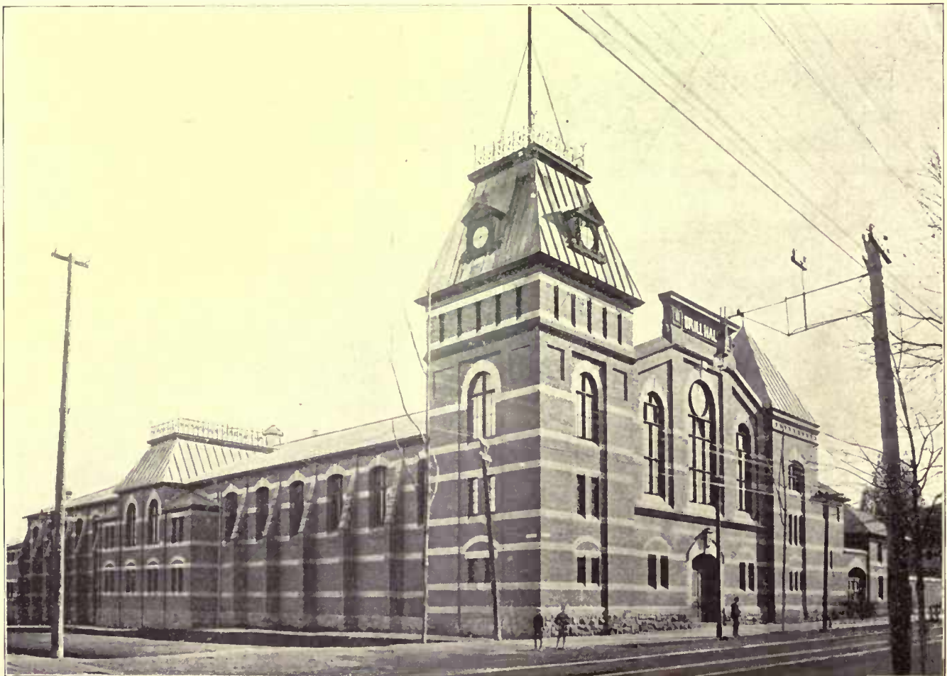
The Drill Hall.
