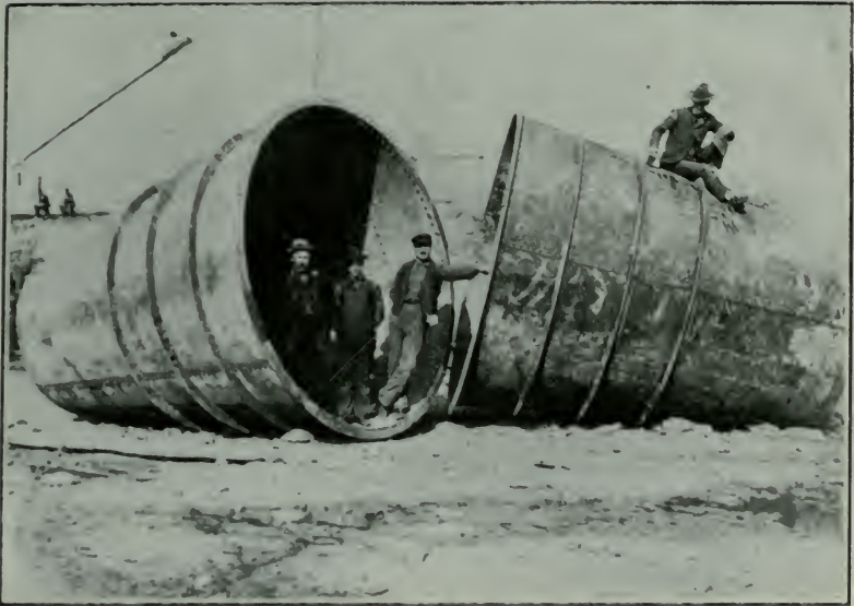
THE HUGE BELLMOUTH INTAKES AT DECEW.
