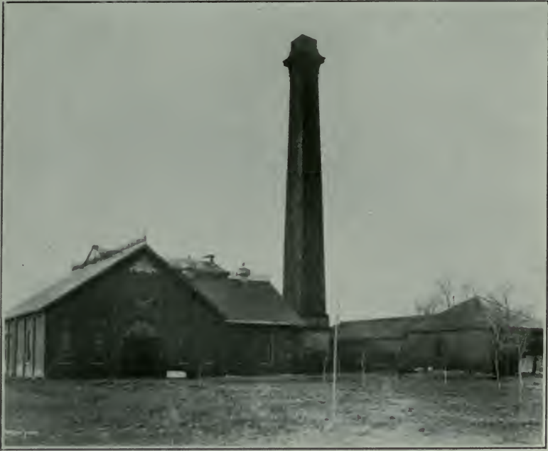
PUMP HOUSE AT THE BEACH
