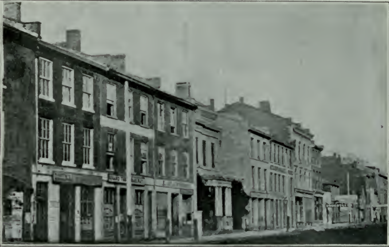
KING STREET WEST FROM JAMES STREET—1853
