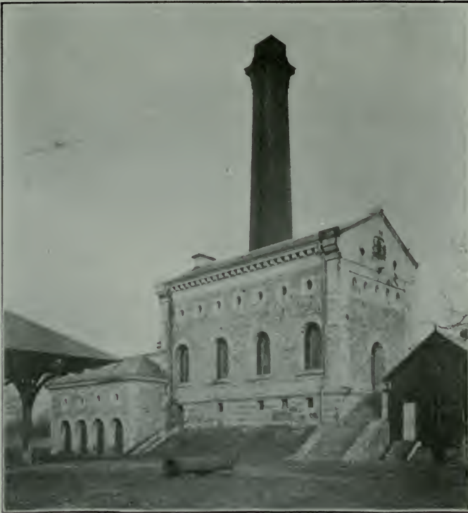
PUMPING HOUSE AT THE BEACH
