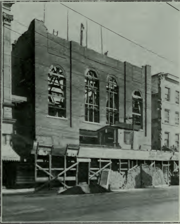
ON JAMES STREET NORTH
