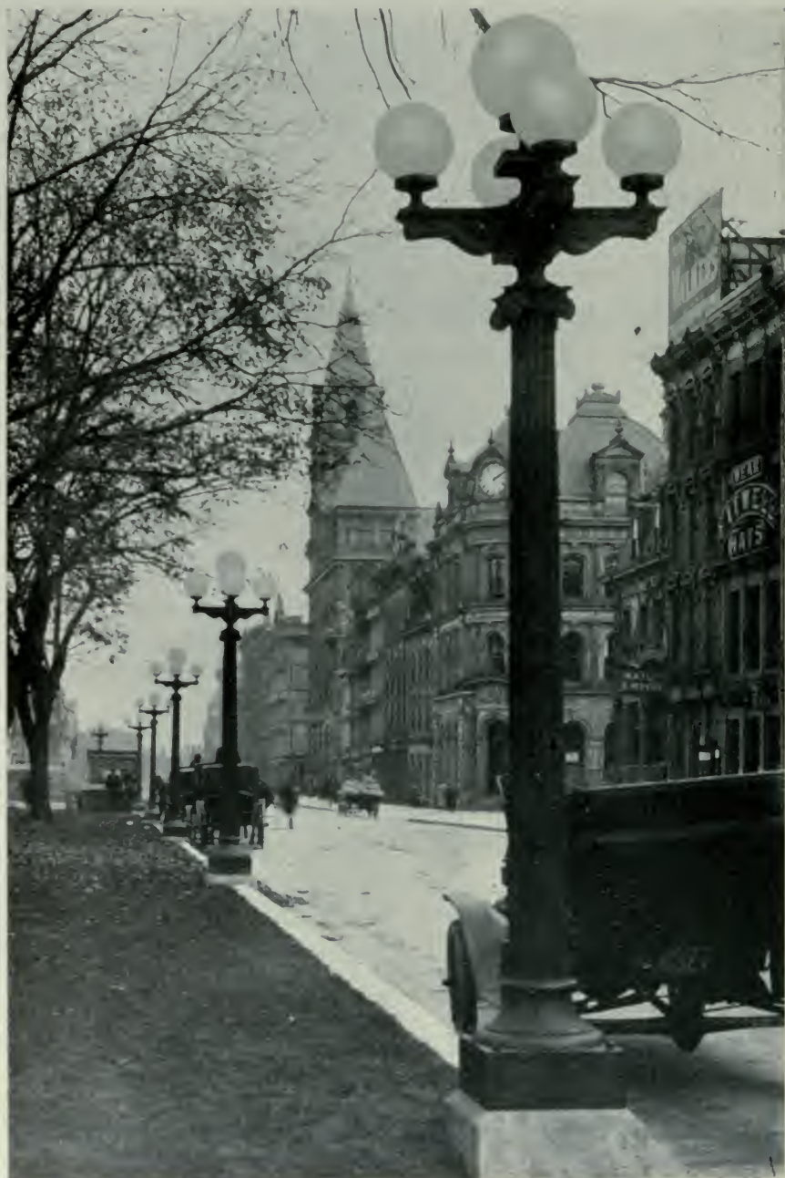
MODERN STREET LIGHTING
