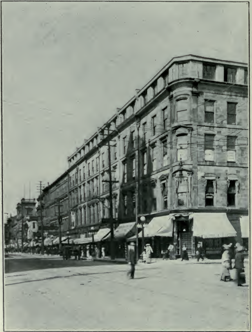
JAMES STREET NORTH, EAST SIDE.
