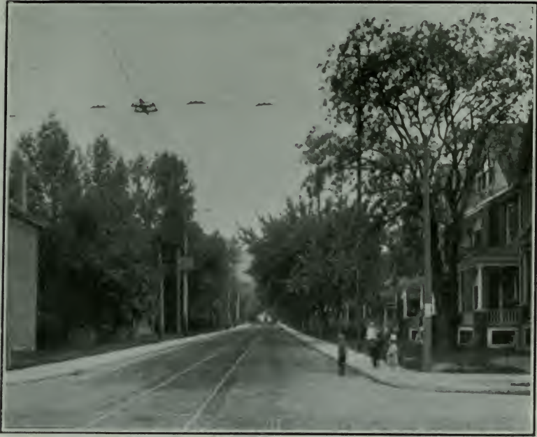
WENTWORTH STREET LOOKING SOUTH
