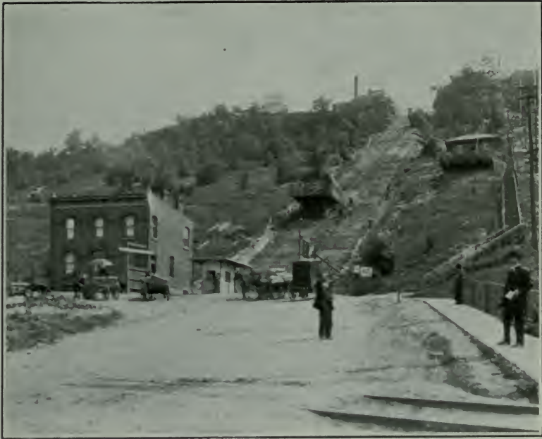
EAST END INCLINE RAILWAY
