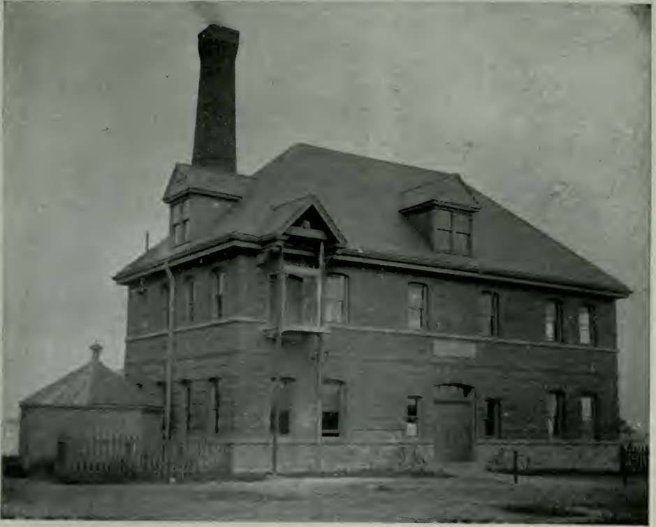
INTERCEPTION WORKS, FERGUSON AVENUE
