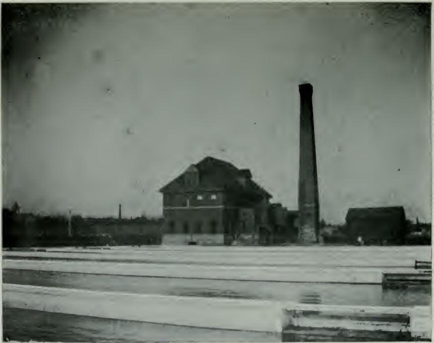
WENTWORTH INTERCEPTION WORKS
