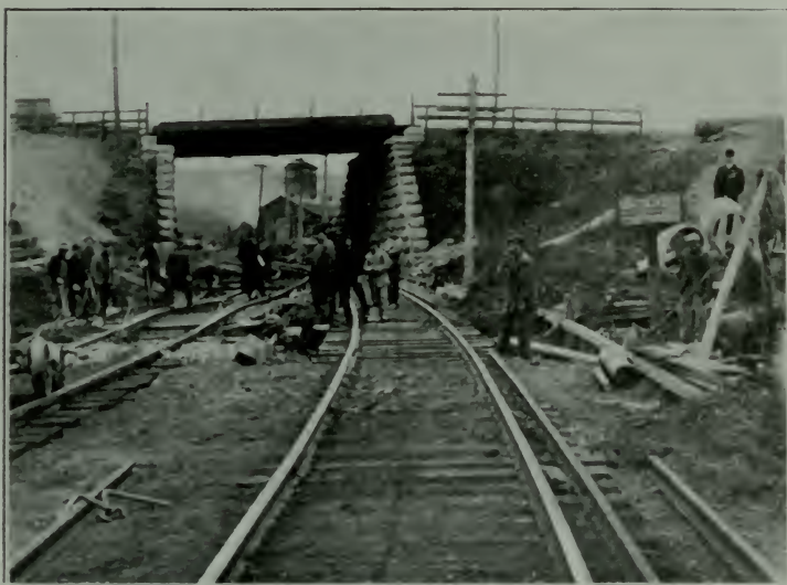
MAIN STREET SEWER UNDER C. P. R.
