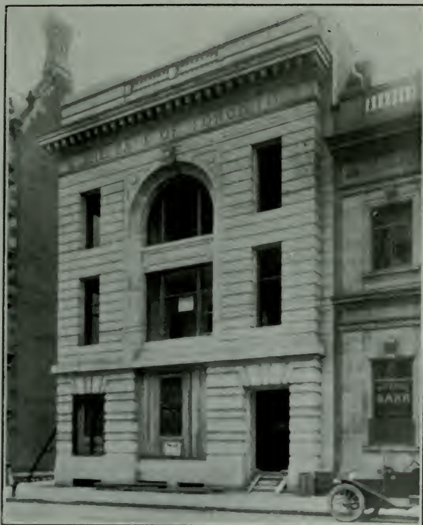
THE BANK OF TORONTO. (Under Construction.)
