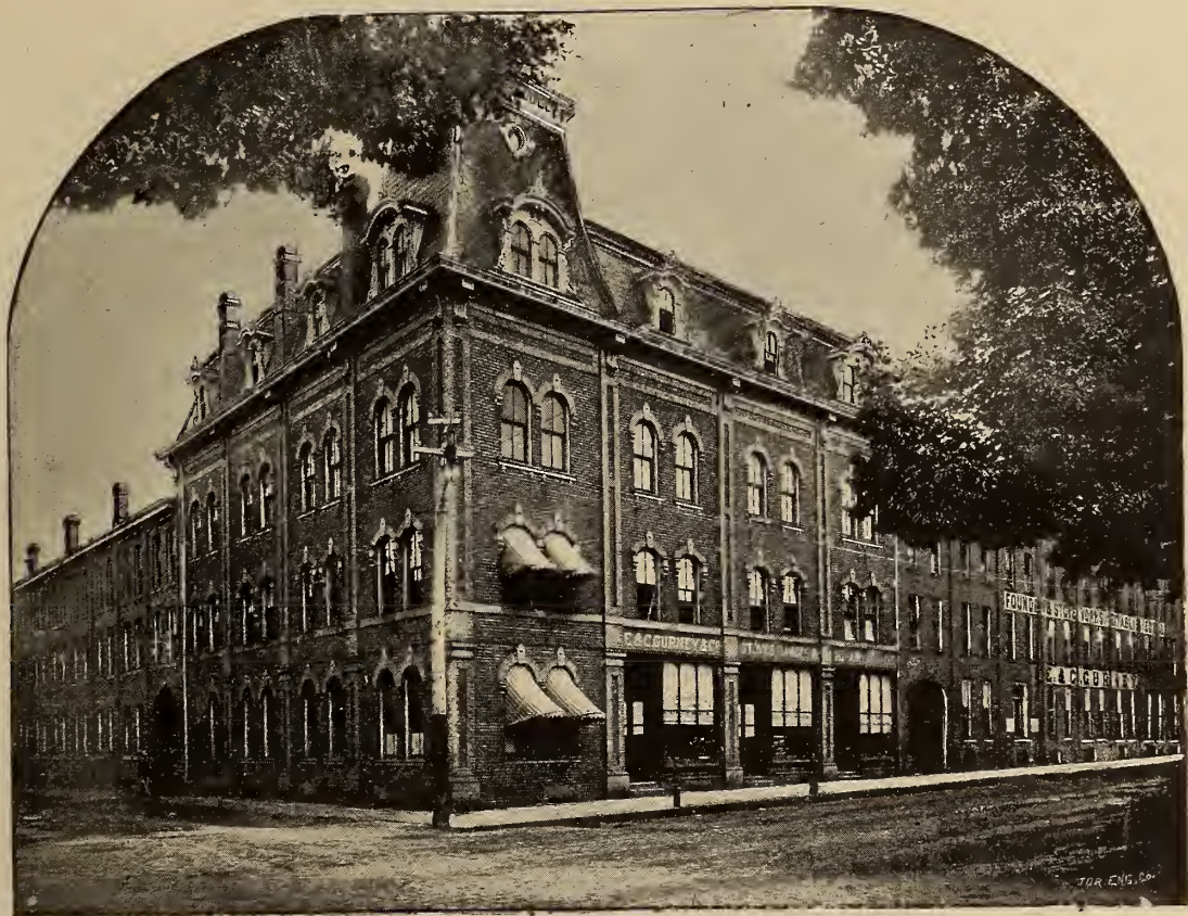
E. & C. GURNEY & CO'S WAREHOUSE AND FOUNDRY.
