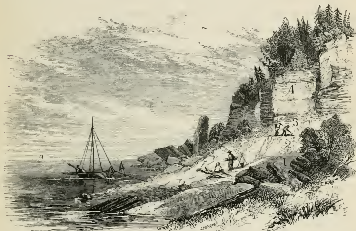
Exposure on Deer Island, near Grindstone Point.
