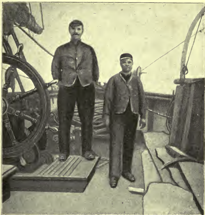
JOHANSEN AND PETTERSON AFTER CLEANING THE BOILERS.
