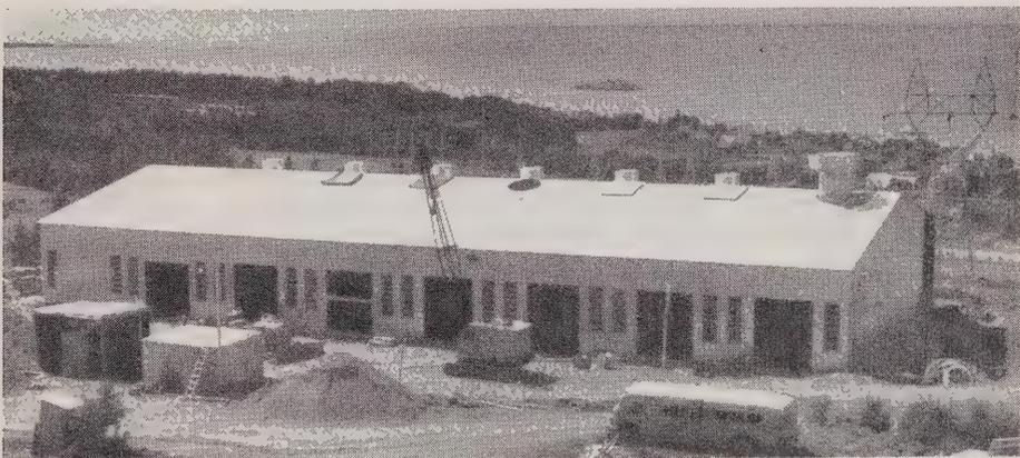
A 36,000 kw. gas turbine plant at Les Boules, Que. will act as a standby plant for the Gaspé Peninsula which is now served by 28 miles of underwater cable, laid in 1954. The present system has been difficult to maintain, due to severe weather and ice conditions. The new plant will also provide extra capacity to meet the winter peak and will act as a synchronous condenser for most of the time. This is Hydro Quebec's first thermal plant.
