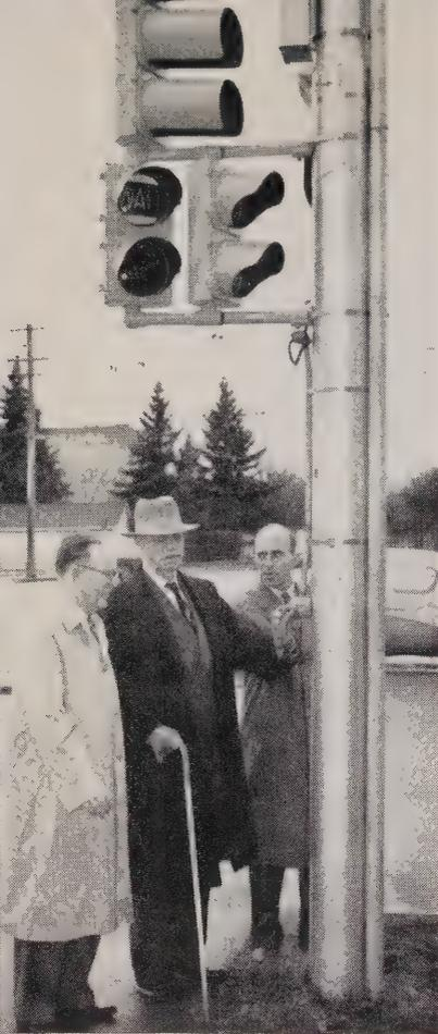
An experiment in the use of "traffic audio-lights" has been tried out in Edmonton, Alberta. A fast "beep" tone, synchronized with the lights, means it is safe to cross north and south, and a slow "beep", east and west.
