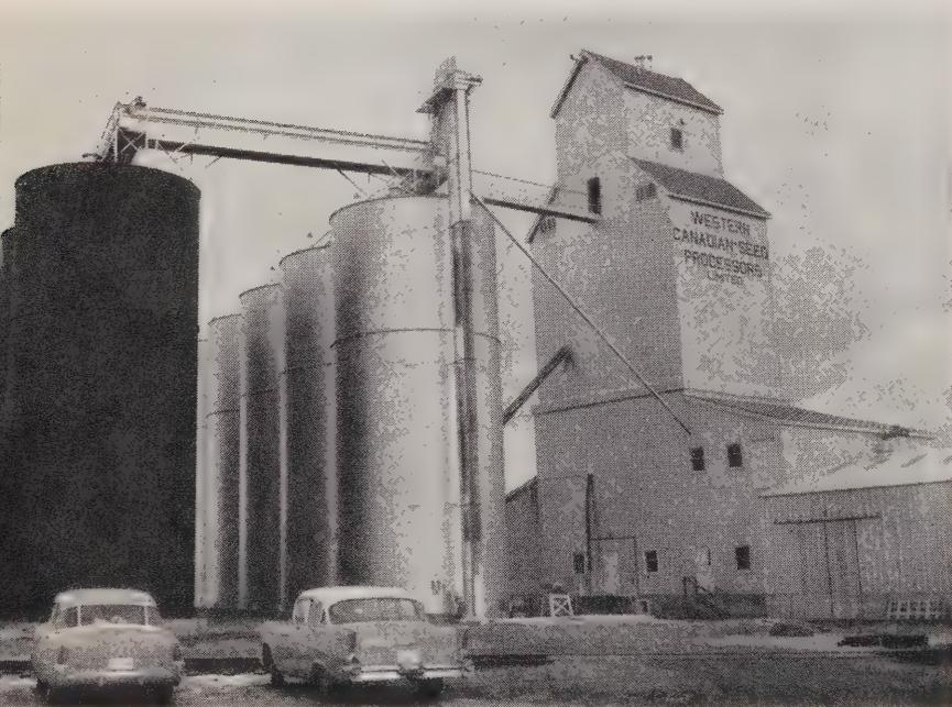
This new oil-seed crushing plant at Lethbridge, Alberta, came into operation in 1960 with an initial capacity of 60 tons of crude oil daily. It also has facilities for seed-cleaning.
