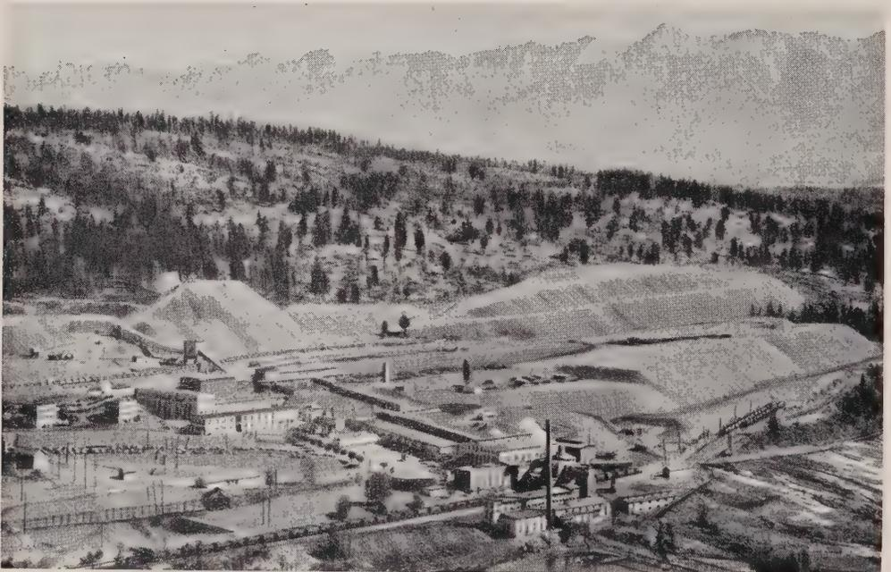
The first of two plants has been completed in a \$20,000,000 iron and steel project to extract iron from the huge piles of tailings from the lead and zinc mine at Kimberley, B.C.
