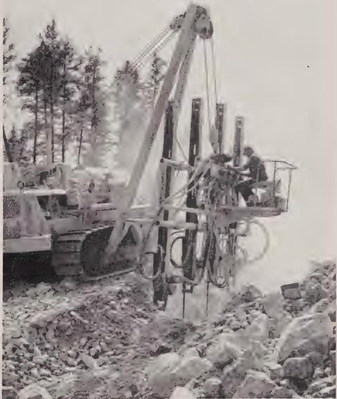
Four shot holes are made simultaneously by this "quad-drill", used in the construction of natural gas pipeline. The holes are tamped with explosives and detonated. In northern Ontario, granite first had to be blasted from the right-of-way to enable equipment to get through and then the five-foot-deep ditch was blasted out, mile by mile.
