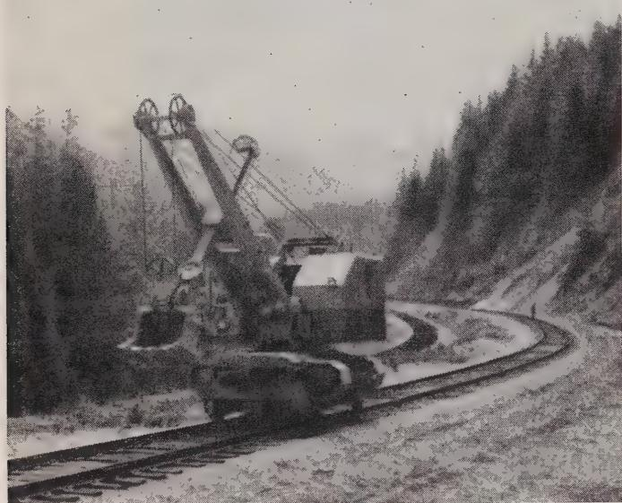
The "rail-aid" moves along railway track under its own power, rolls off its own rail car which it then removes from the track, and goes about its business of cleaning ditches, widening banks, moving ballast, loading or unloading cars, assisting in repair work on trestles or even pile-driving.
