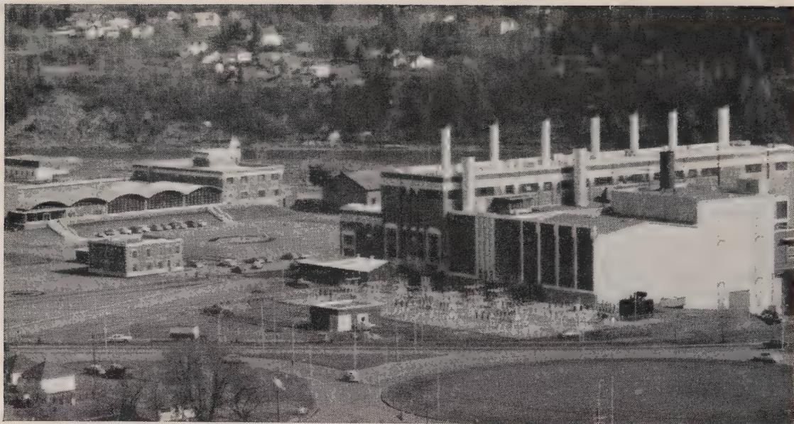
The most spectacular expansion of thermal facilities planned outside Ontario is in Alberta. The present net thermal generating capacity of about 600,000 kw. will be more than trebled by 1970. Recently extended is the thermal-electric plant at Edmonton, flanked by the city's water treatment plant on the left.
