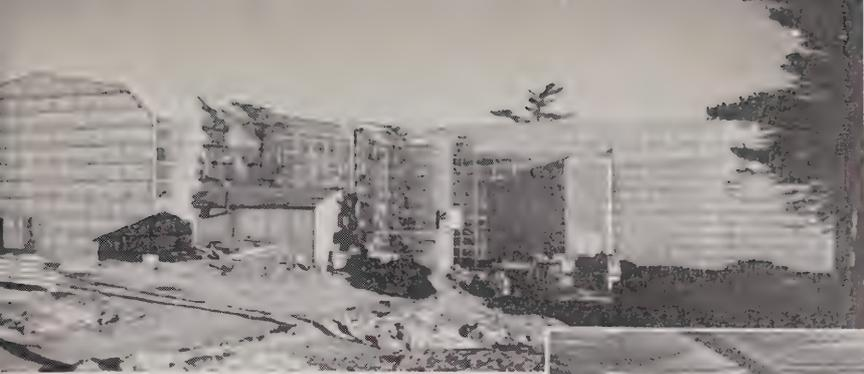
Polyethylene film, supported by laminated wooden frame structure, encloses the new Arts Building at the University of New Brunswick. No interior heating is needed during sunny days, as the film traps the sun's rays.
