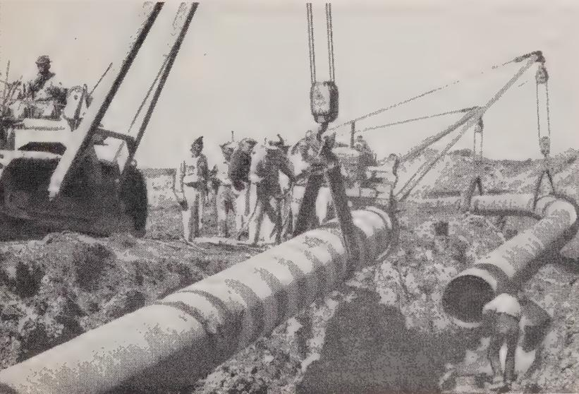
Laying the 51-inch pipeline from Winnipeg to the international border near Emerson, Manitoba. The first gas deliveries through this line to the United States took place in October, 1960.
