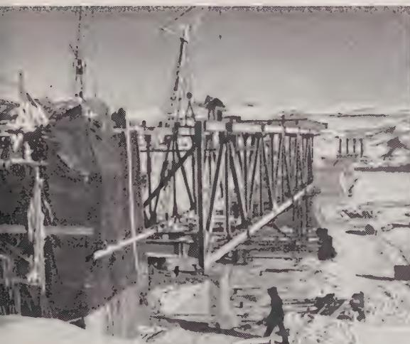
Steel erection on the cantilever section of the Champlain Bridge over the St. Lawrence Seaway continues during winter, thanks to Arctic clothing, safety precautions and improved machines.
