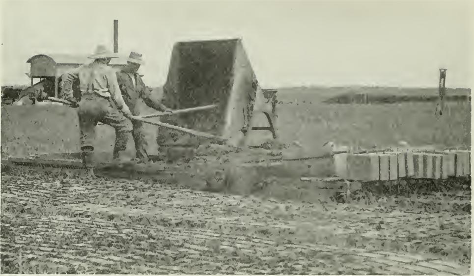
THE PEAT-DRYING FIELD, SHOWING THE METHOD OF AIR-DRYING THE PEAT BRIQUETTES TO FIT THEM FOR BURNING. ONE OF THE HARDEST PROBLEMS OF PRACTICAL PEAT PRODUCTION HAS BEEN THE REDUCTION OF ITS 85% OF WATER TO ABOUT 25%
