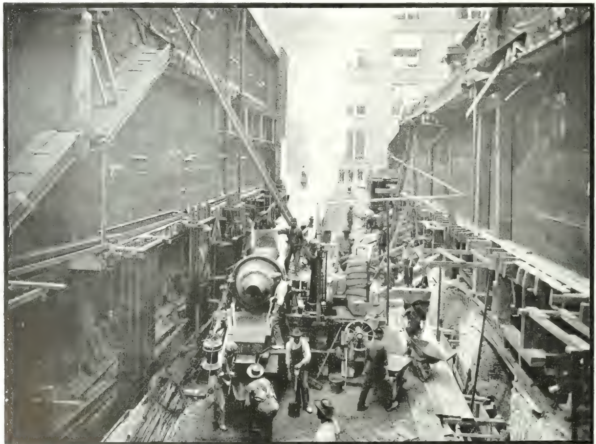
Progress View, Mason & Risch Piano Warehouse, Yonge Street, Toronto. Showing the Concrete Mixer and Limited Space Available in Which to Carry on Operations. On the Left is Seen the Beginning of Column Steel Before Column Boxes Have Been Placed. Bond & Smith, Architects.
