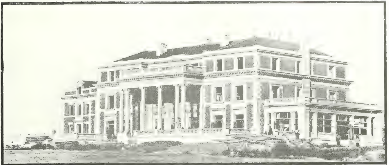
Country Residence on Model Farm of O. C. Barber, Two Miles East of Barberton, Ohio. Built Throughout of Concrete Blocks With a Brick Panel Veneer on the Exterior. The Interior Walls and Partitions Consist of Rough Blocks, Furred with Expanded Metal and Plastered; the Basement Walls Being Tarred on the Outside and Finished With White Faced Blocks Within. Over 42,000 24-inch Blocks Were Required in the Construction of this Building Alone. Harpster & Bliss, Architects.
