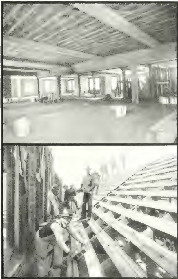
Concrete and Hollow Tile Construction. Upper View: Interior, Showing Complete Floor. Lower View: Method of Laying Tile on Concrete Roof Supports. This Type of Work Bids Fair to Attain Considerable Popularity, both Owing to Economy in Cost and the Light Yet Strong Form of Construction of Which it Admits.
