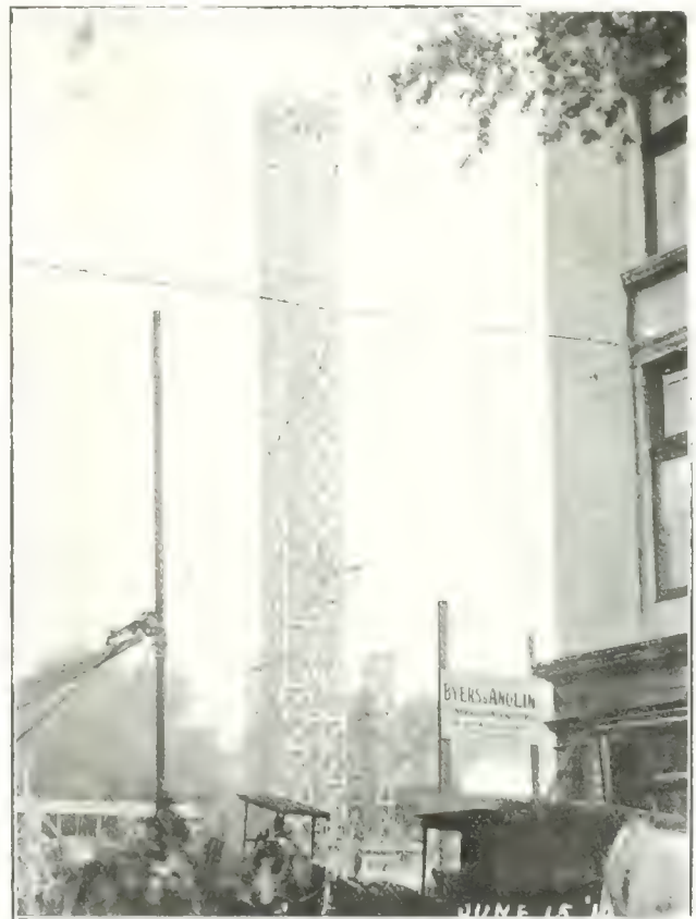
Progress Photograph 3.—Showing Main Tower Nearing Completion, with Stone Tower to Left Immediately Behind, and Sand Tower to Right. The Detail of Excavator Jib, Mast, Swivel Connection and Locking Lever is Seen at Extreme Left.
