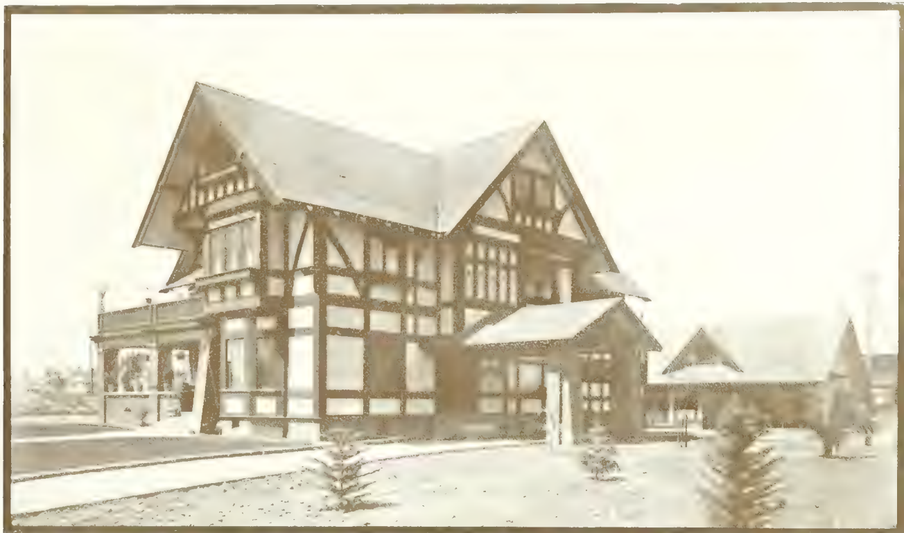
Residence of Dr. W. T. McArthur, Los Angeles—Showing the Carriage Approach and Porte Cochere. The Wall Construction is of Frame with Cement Plaster on Metal Lath, a Type of Construction not Uncommon in Many Parts of California. R. Mackay Fripp, Architect.
