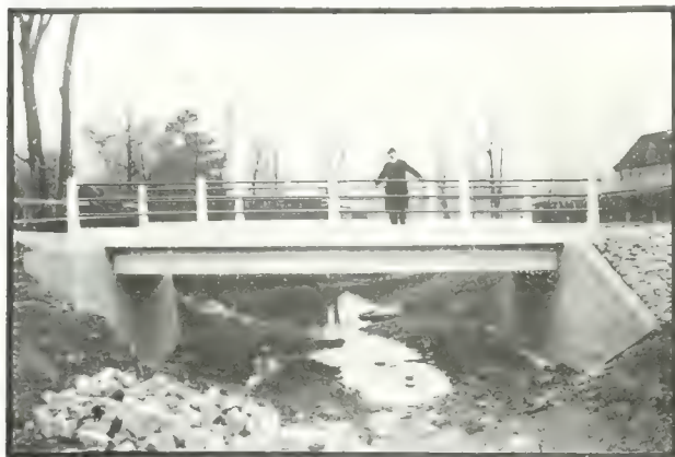
Fig. 2.—Deck Girder Bridge of 33 Feet Span on Beecher Street, Brockville. The "Stubby" Appearance of Short Span Concrete Girders with Solid Parapets is Avoided by the use of a Gas-Pipe Railing. Barber & Young, Engineers.
