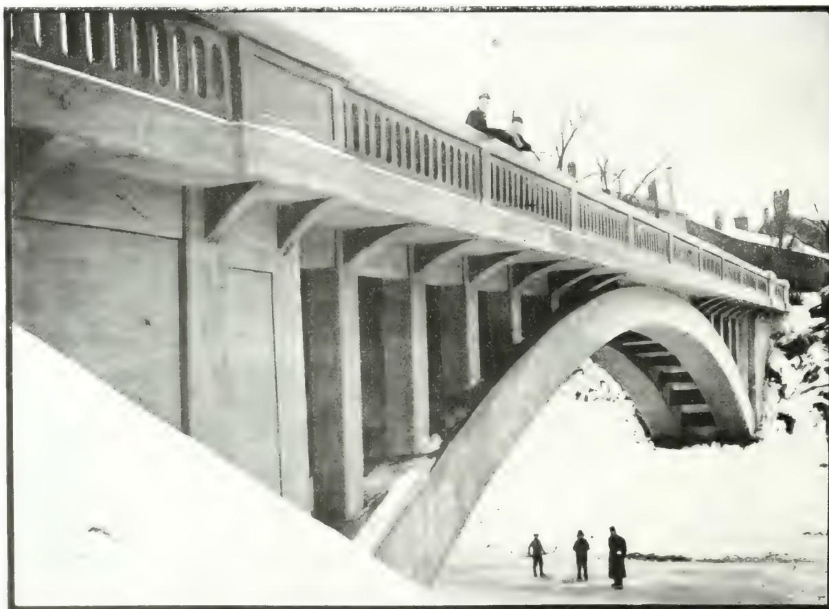
Fig. 6.—The Wadsworth Arch Bridge over the Humber River at Weston, Ont. It is Believed that the Span of this Bridge, 118 Feet 6 Inches, is the Longest Yet Attained in Concrete in Canada, and that This is the Only Completed Example of a Ribbed or Open Spandrel Arch in the Country. Barber & Young, Engineers.
