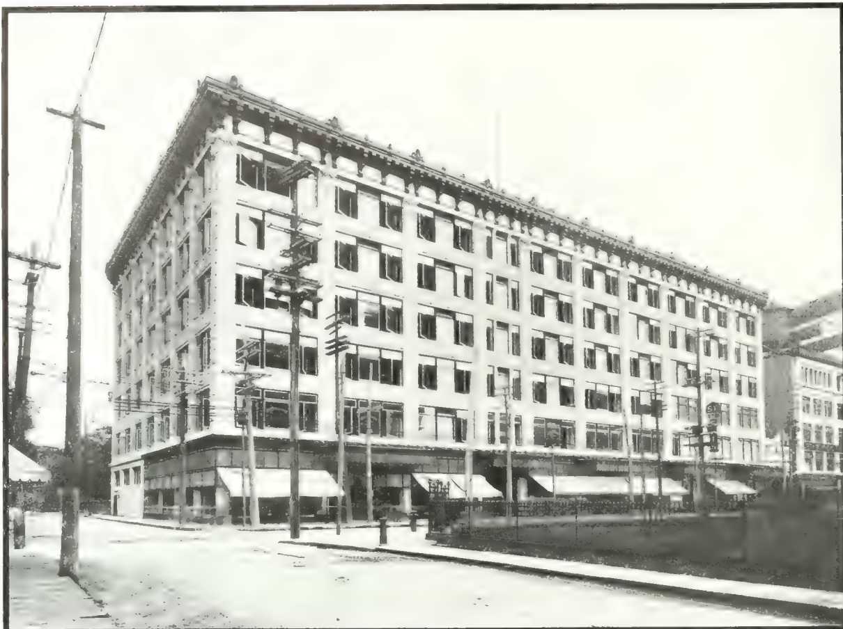
The Jacobs Building, St. Catherine and St. Alexander Streets, Montreal. Built of Reinforced Concrete with Terra Cotta Exterior Facing, and Notable as Largest Building of this Type of Construction in Canada. Mitchell and Creighton, Architects.
