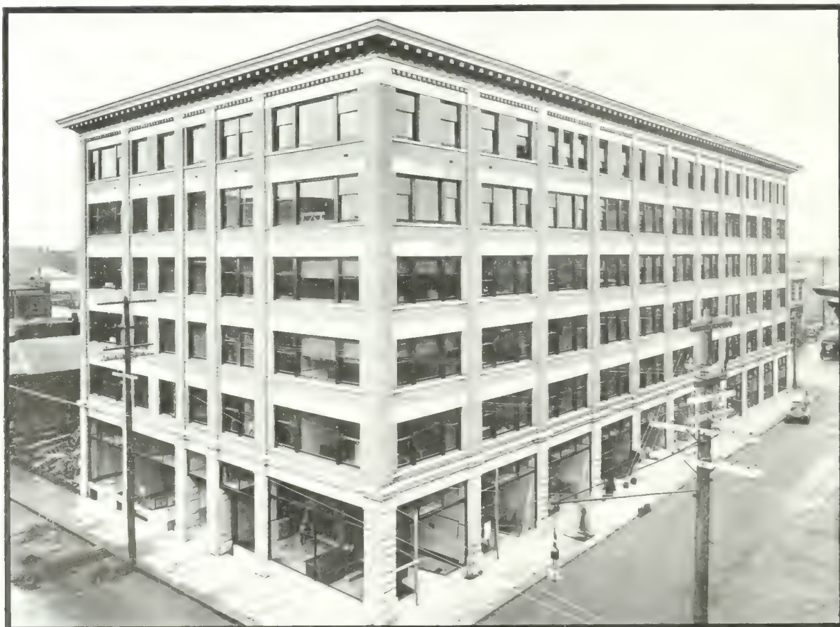
Pemberton Block, Vancouver, B.C. A Large Reinforced Building Which is Interesting as an Example in which the Floor System Extends to Form the Outer Wall Beams, and in this Manner is incidentally Made to Serve as a Simple Decorative Feature for the Brickwork. G. C. Mesher & Company, Architects.
