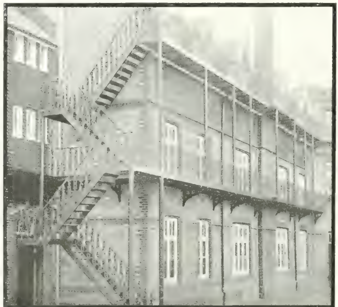
Possibly after a few more such catastrophes, people on this continent will become a trifle more serious in insisting upon proper fire protection and proper public inspection, by honest, efficient and public spirited officials. The above is a fire escape on a three story college in England, erected according to the requirements of the London County Council.
