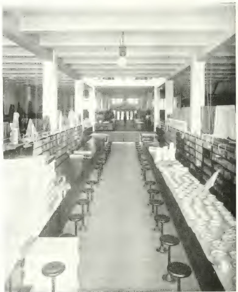
View of Interior on Ground Floor—Showing the Arrangements of the Beams, Columns and Girders. C. P. Meredith, Architect.
