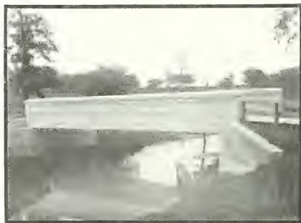
Fig. 3.—Through Girder Bridge of 50 Feet Span at Unionville, Ont. A Less Economical Type than the Deck Span of Fig. 2, but Necessitated Where the Clearance Above the Water is Restricted. Jas. McDougall, Engineer.
