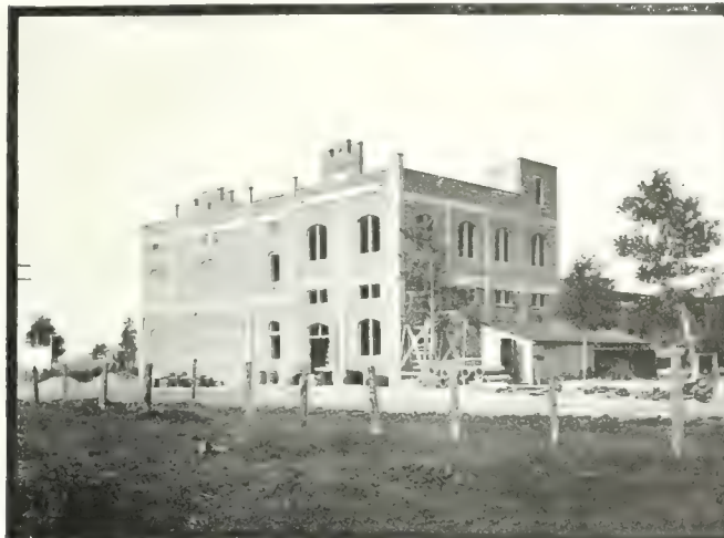
Sudbury Brewery, Sudbury, Ont. A Reinforced Concrete Building in which the Floors are Designed to Carry the Outside Brick Walls. The Views Show the Erection of Form Work and the Structure Practically Completed. Bishop Construction Company, Contractors.
