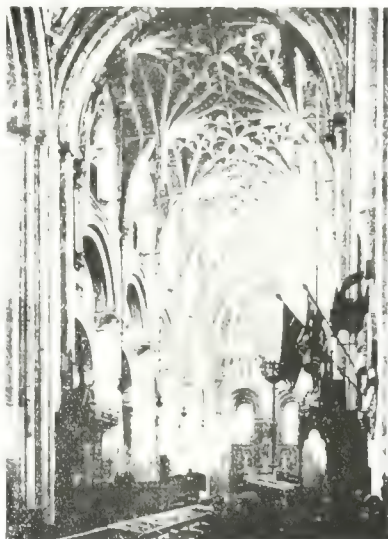
Upper Two Views—Vaulting at Oxford Divinity School, A.D. 1445-1480. Lower Two Views—Vaulting at Oxford Cathedral Choir, A.D. 1478-1503. These are Good Examples of Lierne Rib Vaulting . It Will Be Noted that the Pendants of Each Transverse Arch are But Two of the Voussoirs of the Arch, Greatly Elongated. (From Bond's "Gothic Architecture.")
