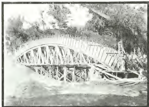
Fig. 8.—The Wadsworth Arch Bridge, with the Rib Forms Erected. These Forms were Supported by Distributing Trusses Resting Upon Timber Bents Founded on the Rocky Bed of the River. Barber & Young, Engineers.
