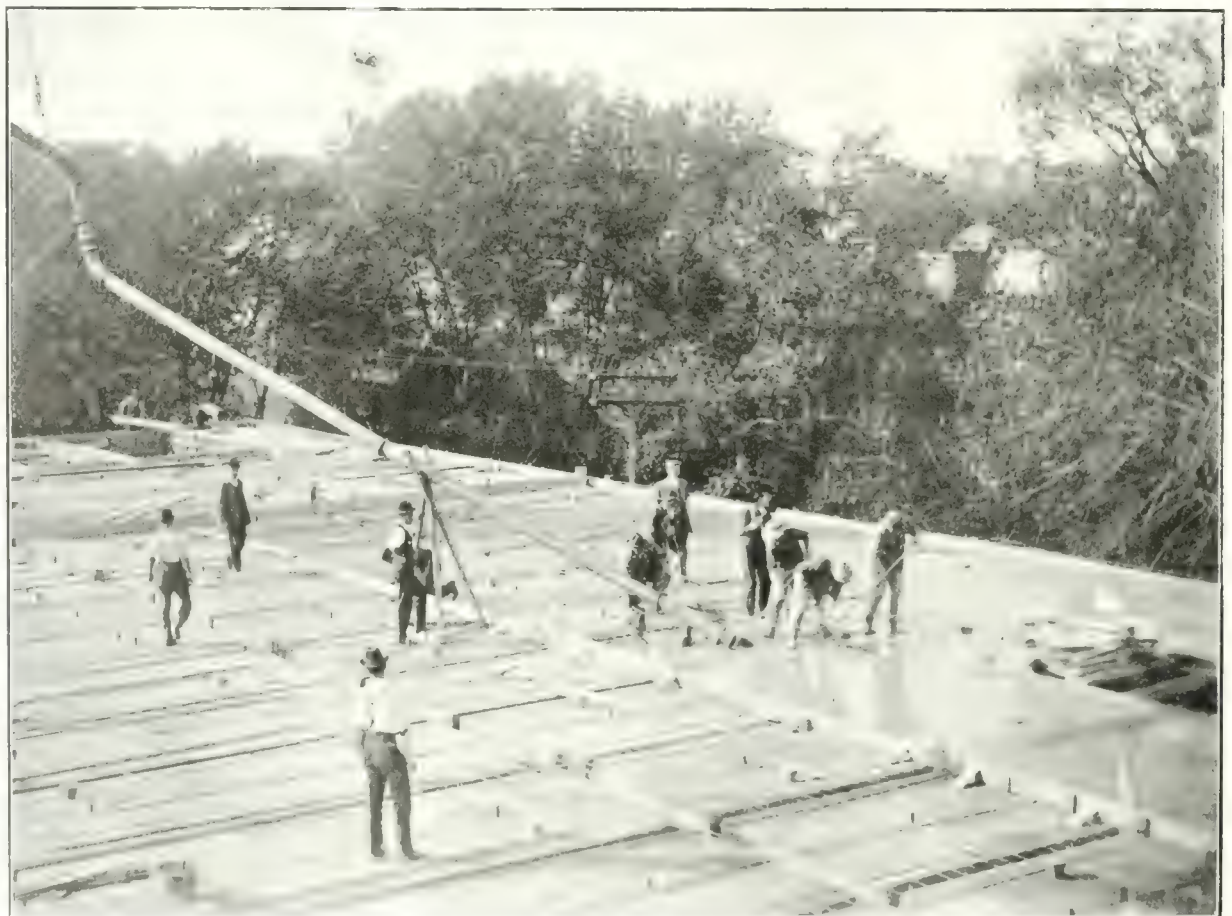
Progress Photograph 5—Showing the Delivery Pipe and Flexible Elbow Used in Pouring the Concrete, and the Method of Breaking Off the Work.
