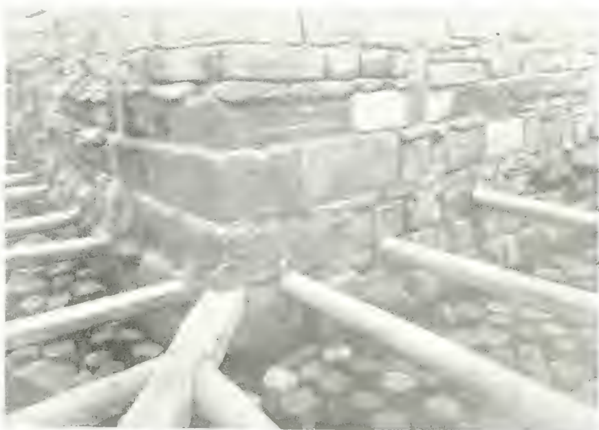
Widening the Foundation, Showing the Old Masonry Work and the Piling for the New Section.
