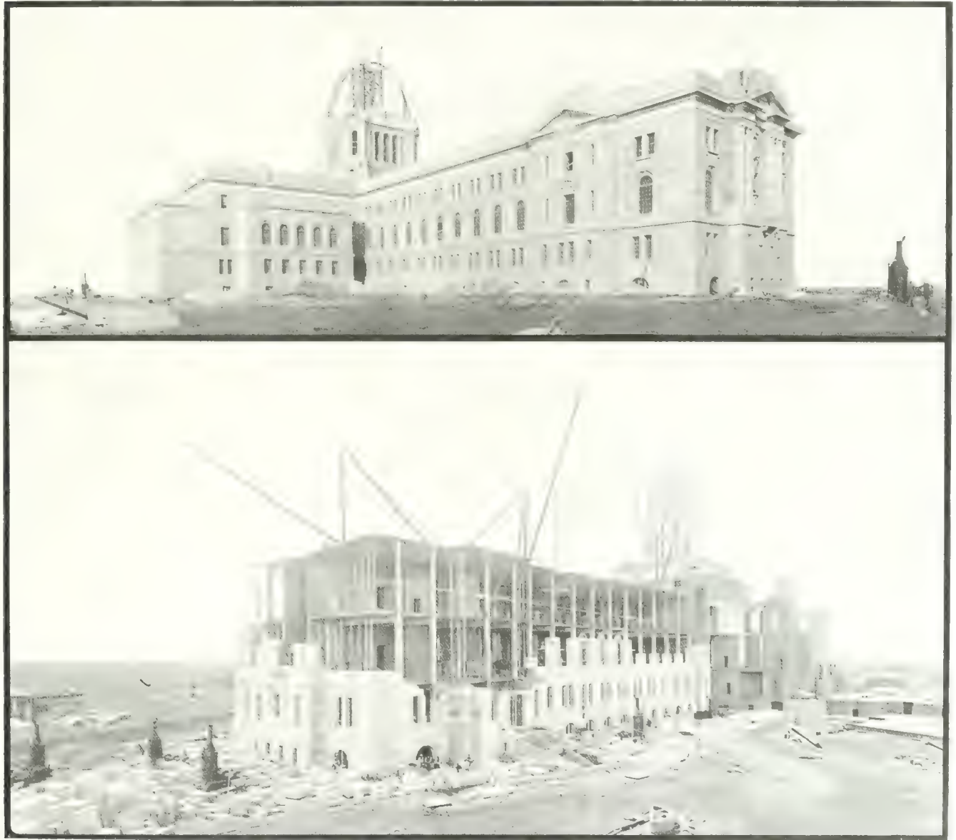
The Saskatchewan Parliament Building, Now in Course of Erection at Regina. The Largest Reinforced Concrete Building in the Canadian West, and the Only Legislative Building of this Type of Construction in the Dominion. The Upper View Shows the Exterior Walls of Stone Practically Completed, and the Lower View the Internal Construction when the Outside Masonry was Only Partially Carried Up. E. & W. S. Maxwell, Architects.
