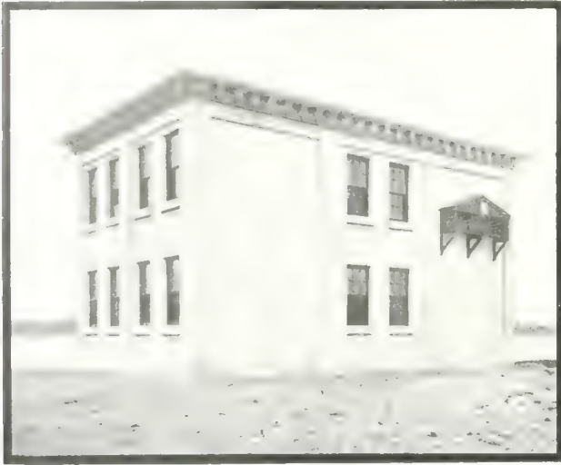
Transformer House at Port Colborne, Ont. An Example of Stucco Work on Monolithic Concrete Construction. J. A. Jamieson, Engineer.
