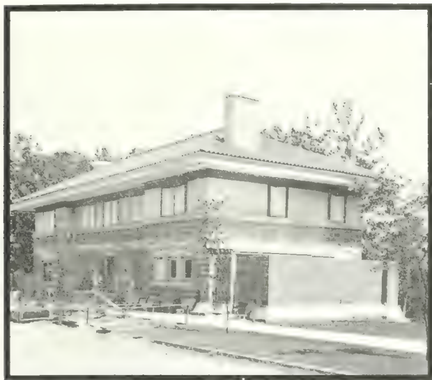
A Concrete Block and Cement Stucco Residence. Showing the Lower Portion Before the Plaster is Applied and the Upper Story Finished.
