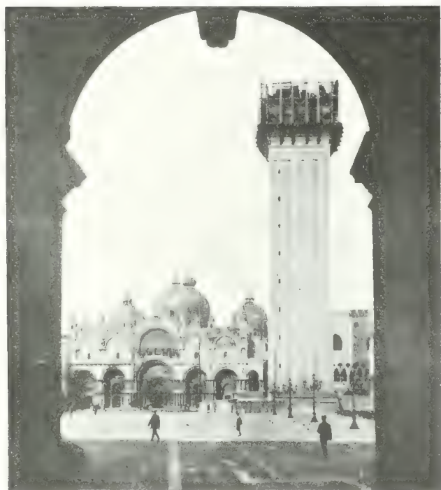
The New Campanile, Venice, as it Appeared Three Months Back, Ready for the Placing of Its Pyramidal Apex.
