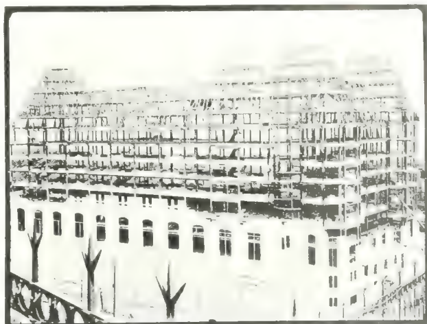
Chateau Laurier, Ottawa's Splendid New Hotel, Now Nearing Completion, and in Which the Structural Parts Throughout are Protected by a Patent Welded Fabric and Concrete Plaster Applied to Metal Lath. Ross and McFarlane, Architects.
