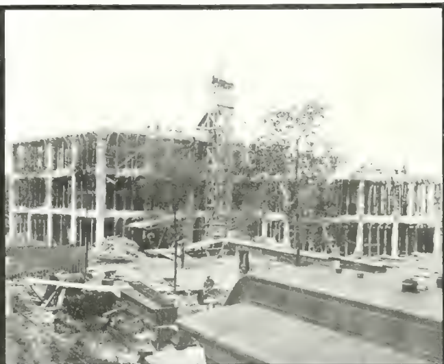
Reinforced Concrete Factory of the Peabody Manufacturing Company, Walkerville, Ont. Showing the Completed Structure and the Form Work when the Building was in Process of Erection. Bishop Construction Company, Contractors.
