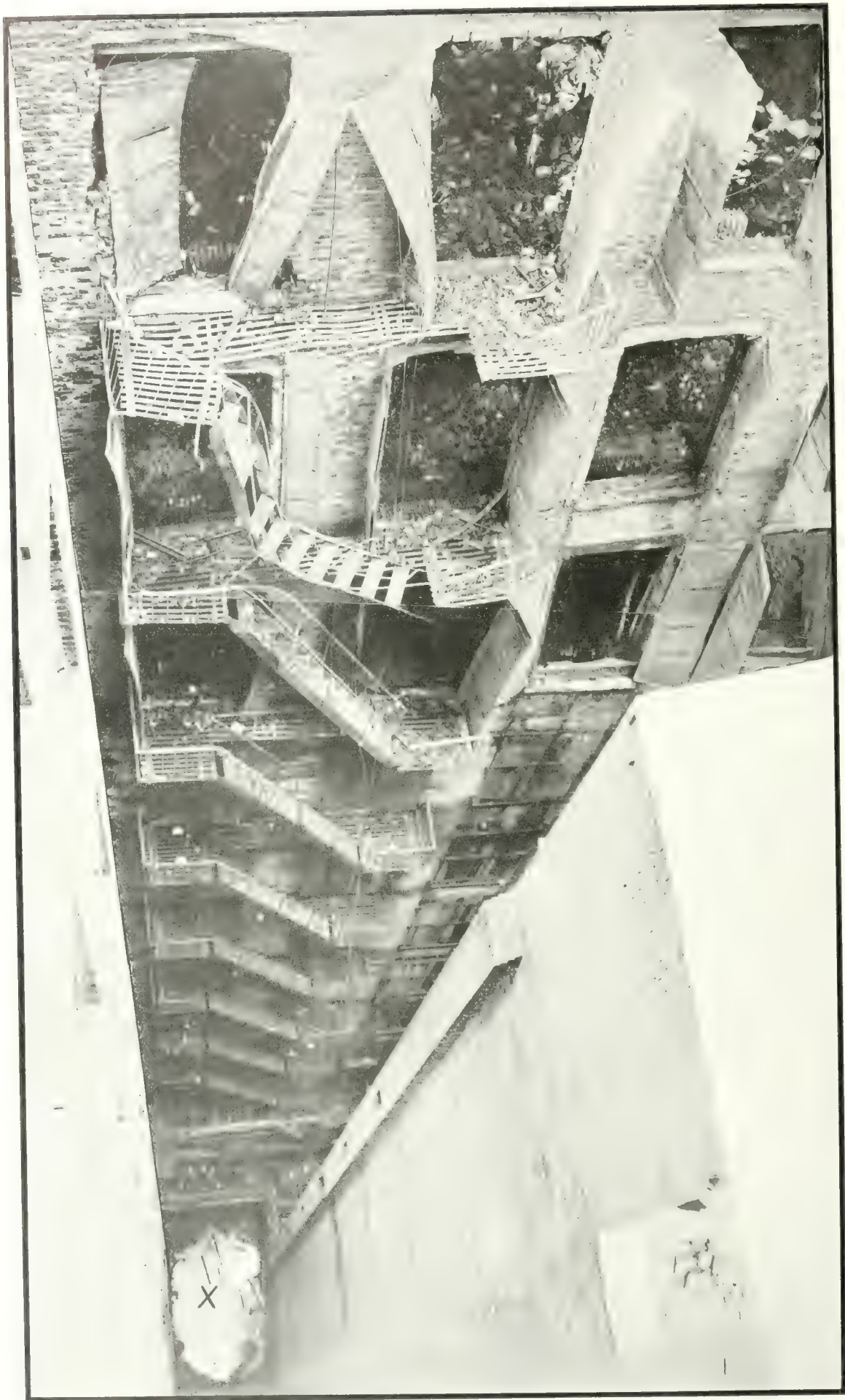
A ten story fire escape in the loft building, Washington Place, New York, in which 141 girls lost their lives. This is a photograph of the fire escape from roof to first story. This miserable excuse of fire escape protection was one of the chief causes of the large number of fatalities in this fire. More than a score of girls fell from these supposed life savers, and their bodies were found in the pit at the bottom of the fire escapes, marked X. These so-called fire escapes are quite equal and in many cases superior in efficiency to what is to be found on our average loft or factory building in either Toronto or Montreal, or in fact anywhere throughout either Ontario or Quebec where large factories are to be found. The City Architect of Toronto, or the Building Inspector of Montreal have to their credit many of such fire escape bungles as the one shown above. The fact that no serious catastrophe has occurred is not a result of the efficiency of the inspection of these departments, but because of good fortune. The fact that this was a ten story building does not change matters a bit, a drop from the fourth or fifth floor would be equally as fatal.
