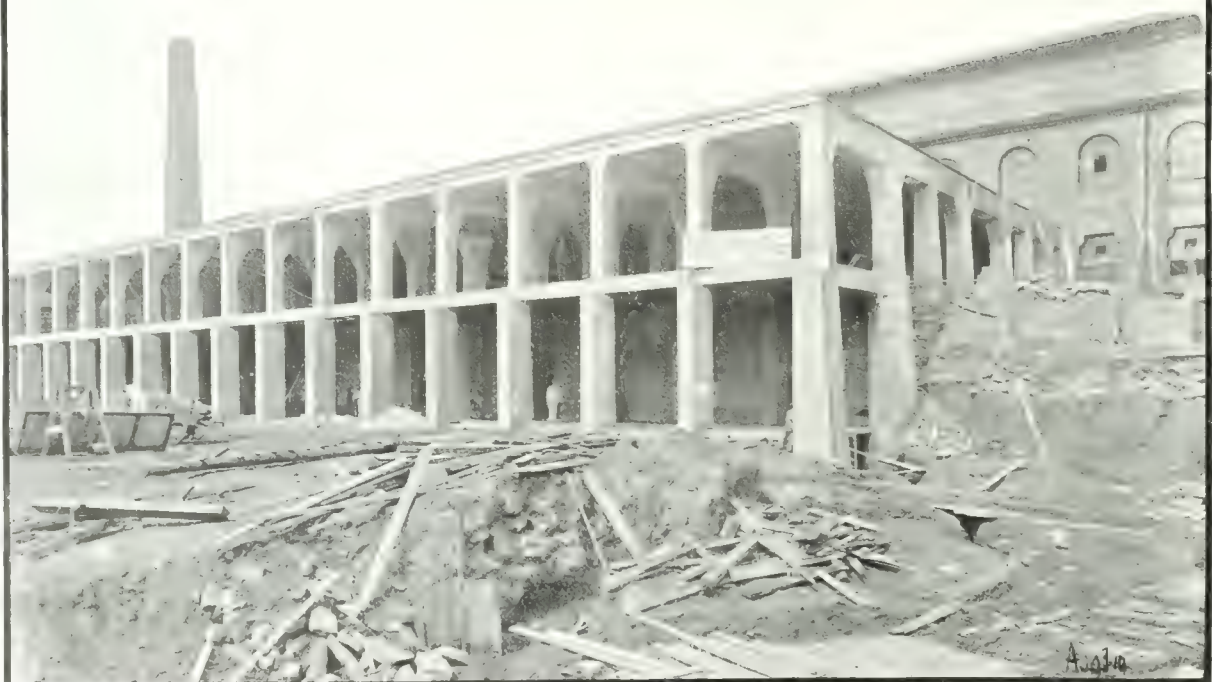
Concrete Viaduct, Windsor Street (C.P.R.) Station, Montreal. Showing Form Work, and Section of Finished Structure, Which is Designed to Carry the Heaviest Type of Locomotives and Passenger Cars. W. S. Painter, Chief Architect. Bishop Construction Company, Contractors.
