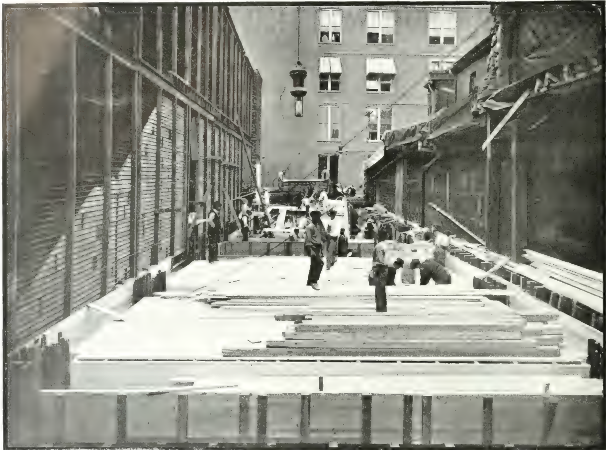
Progress View, Mason & Risch Piano Warehouse, Yonge Street, Toronto. Showing the Hy-Rib Wall (partly plastered) Which was Put in Position to Enclose the McKendry Millinery Store on the South Lot Before the Brick Work of the Intervening Party Wall was Carried Up. Bond & Smith, Architects.
