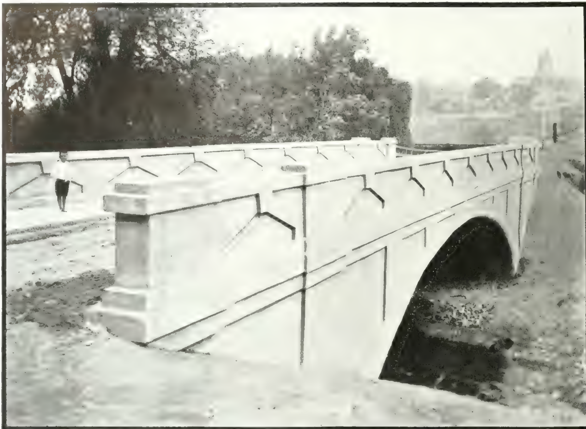
Fig. 5.—Arch Bridge of 60 Feet Span, on Timothy Street, Newmarket. This Structure Being a Permanent Bridge in a Growing Town, Special Care was Taken to Secure a Pleasing Appearance by Accentuating the Arch Ring, Relieving the Spandrels by Pilasters and Employing a Special Decorative Feature in the Railing. Barber & Young, Engineers.
