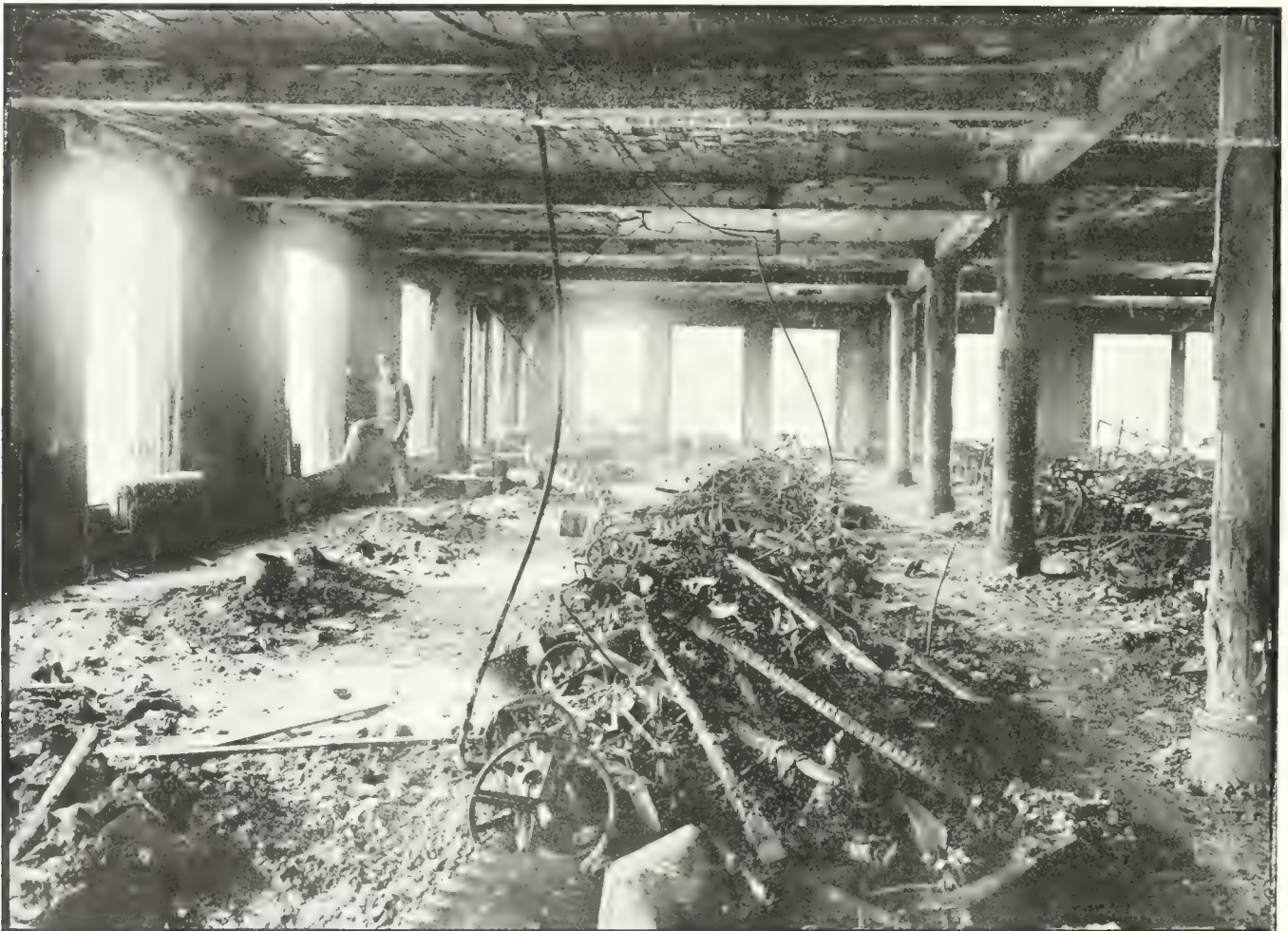
Ninth floor of Loft Building, Washington Place, New York, where a large number of the victims were trapped. Many bodies were found under sewing machines and their postures showed that they were endeavoring to shield themselves from the heat. This illustration forcibly demonstrates the efficiency of modern fireproofing. The twisted pipes and remains of sewing machines show conclusively that a tremendous heat was developed. It further proves that because a building is fireproof, fire fighting and fire protective devices cannot be eliminated. These three stories in which 141 lives were lost remain intact as far as the construction is concerned—the contents fed the flames.
