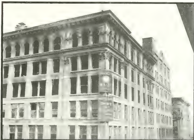
This illustration of the upper three stories occupied by the Triangular Waist Co., taken after the fire, shows how the building proper still remains intact. It is absolute proof that the contents of a fireproof building, filled with inflammable goods, requires life saving and fire fighting apparatus just as much as a non-fireproof building, as far as the protection of life is concerned. If this building had been equipped with a sprinkler system, history would not have had to record such a shameful holocaust.
