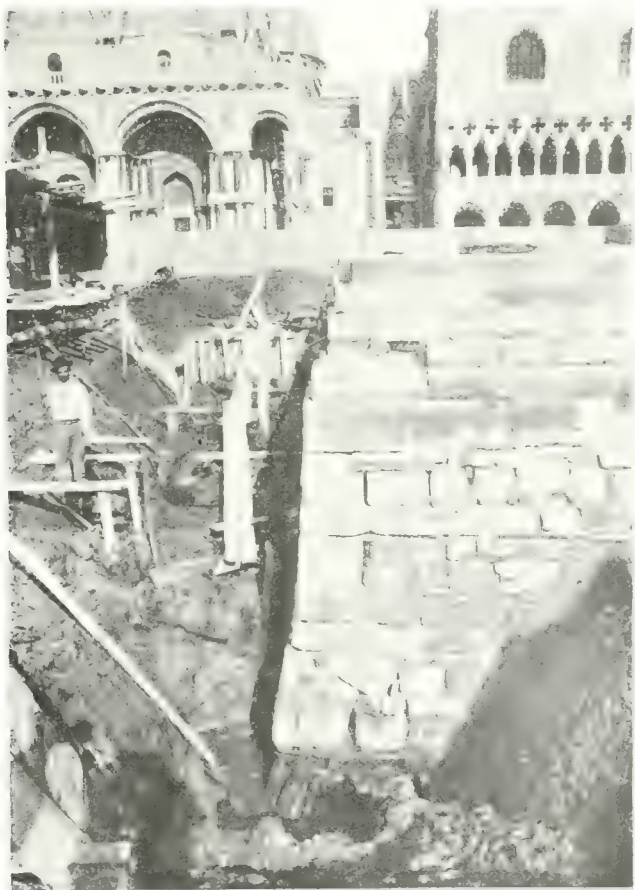
Excavating the Ground Around Foundation of Campanile, Preparatory to the Work of Restoration.
