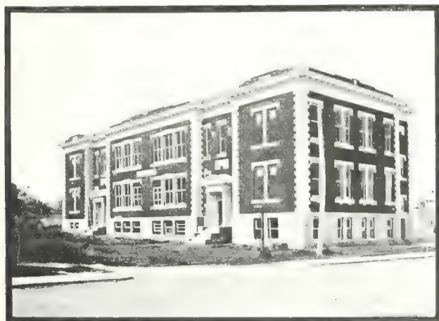
Querbes School, Outremont, District of Montreal, in Which Concrete Plaster on Metal Lath has been Extensively Adopted, Owing to the Fire-Resisting Properties of this Form of Construction, and the Sanitary Advantages Which it Affords. Joseph Perrault, Architect.
