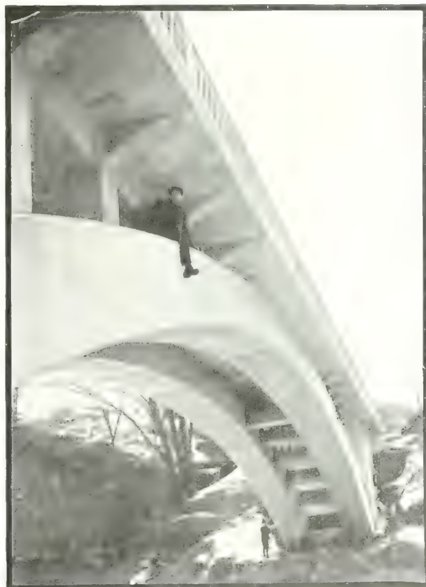
Fig. 7.—A View of the Wadsworth Bridge, Weston, from Underneath. The Massiveness of the Ribs and the General Size of the Structure is Apparent by Comparison with the Figures in the Illustration. Barber & Young, Engineers.
