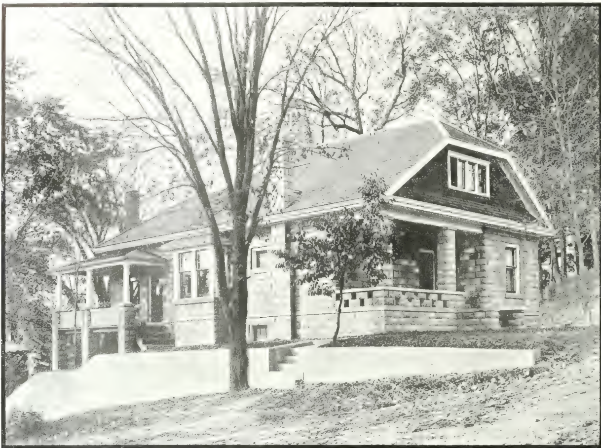
Residence of Rev. William Potter, Dundas, Ont. A Six-Room and Attic Dwelling Structure Constructed of Concrete Blocks, and Erected at a Complete Cost of $2,600. M. H. Hewitt, Architect.
