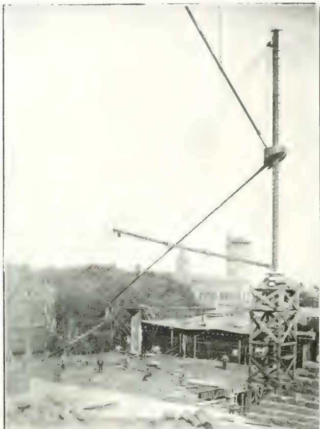
Progress Photograph 7.—Showing Distributing Tower at Work.
