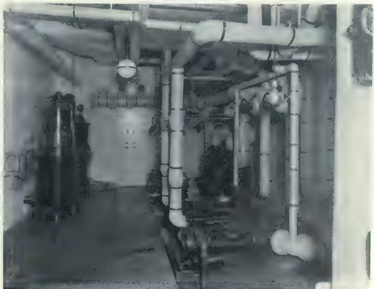
FIGURE IV. VACUUM CLEANER, BOILER FEED AND HOUSE PUMP.
