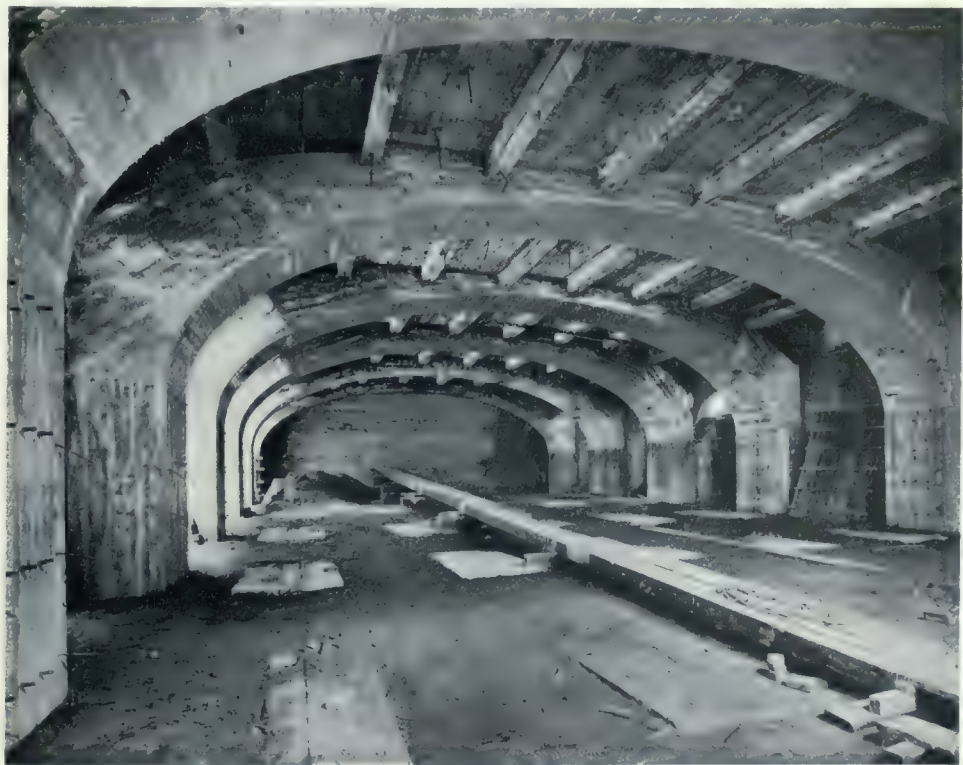
VIEW OF AUDITORIUM SHOWING CONSTRUCTIONAL ARCHES.
