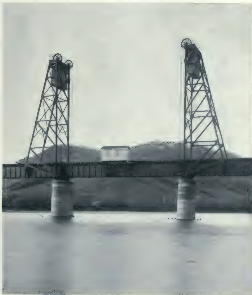
DETAIL OF VERTICAL LIFT AT KAMLOOPS.
