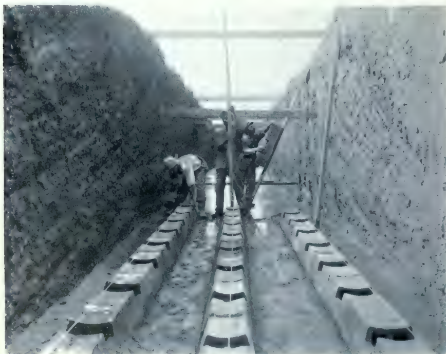
BASE DRAIN TILE LAYING TO RECEIVE STEAM AND HOT WATER MAINS ON TOP. TILE MADE AT GOVERNMENT CLAY PLANT.
