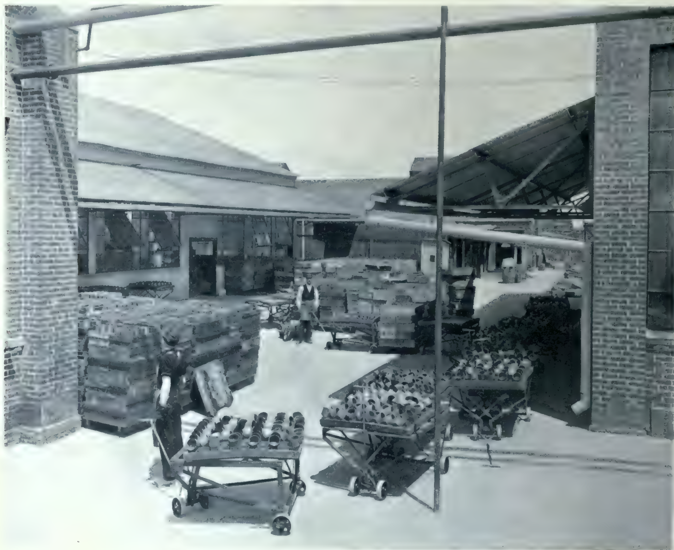
METHOD OF COOLING CASES AFTER ANNEALING, CANADIAN CARTRIDGE CO., LTD., HAMILTON, ONTARIO.
