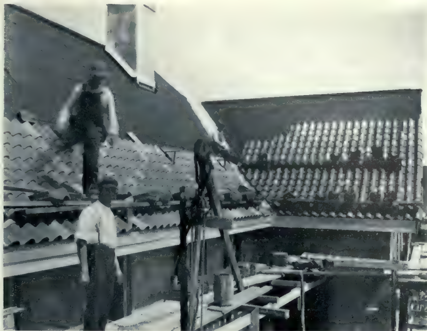
LAYING SPANISH ROOFING TILE MADE AT GOVERNMENT CLAY PLANT.
