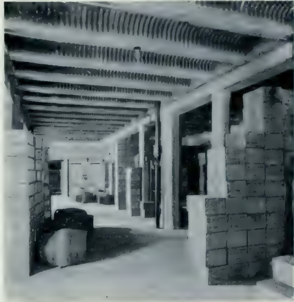
FIREPROOF CONSTRUCTION FEATURES OF D. O. ROBLIN WAREHOUSE.
