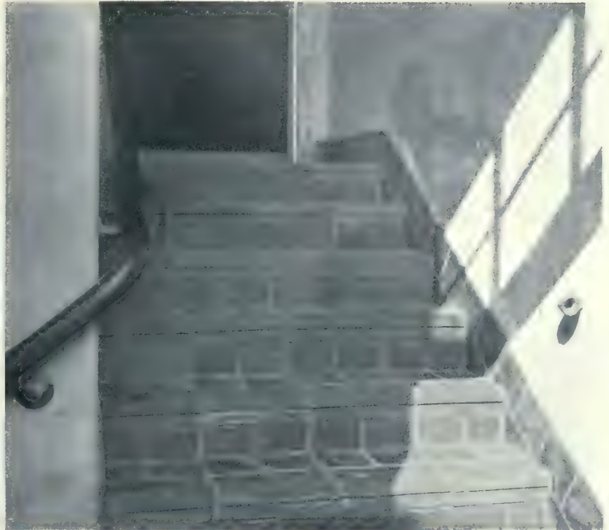
TYPICAL STAIRCASE, SHOWING USE OF SPECIAL STEP NOSING, STRINGER AND OTHER TILES MADE AT GOVERNMENT CLAY PLANT.
