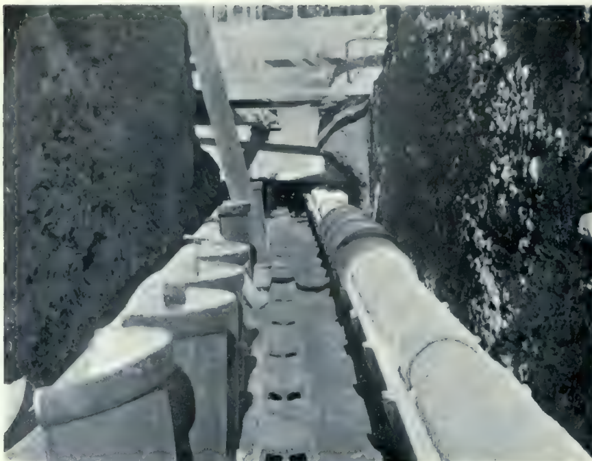
HOT WATER AND STEAM MAINS INSULATED WITH CONDUITS.
