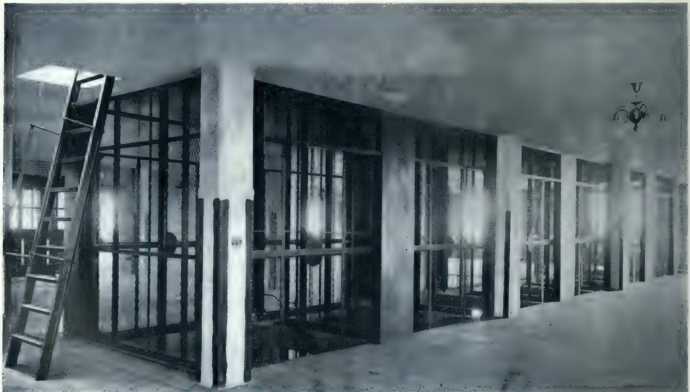
ELEVATOR SHAFT, CUSTOMS EXAMINING WAREHOUSE, MONTREAL, QUE.
