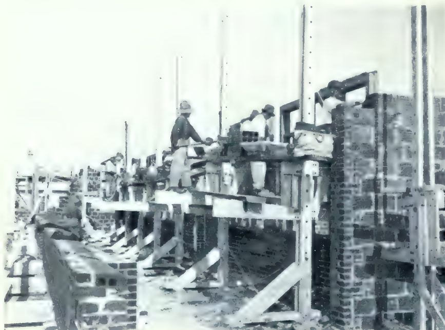
GILBRETH SCAFFOLD BEING RAISED WHILE BRICKLAYERS CONTINUE THEIR OPERATIONS.
