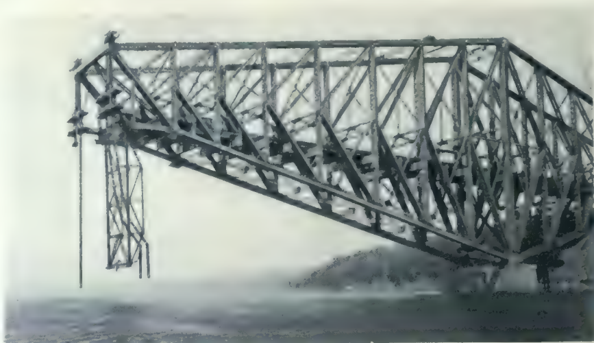
NORTH SHORE CANTILEVER WITH CENTRE SPAN LIFTING APPARATUS AT OUTER END.
