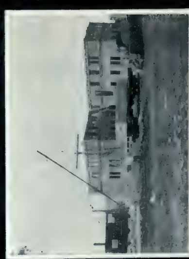
Lifting Beams directly by Travelling Crane to Upper Floors
