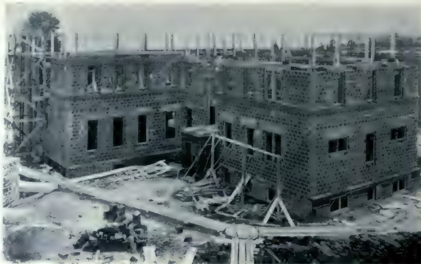
A COTTAGE UNDER CONSTRUCTION. NOTE USE OF LIGHT RAILWAY AND HOIST FOR DISTRIBUTING MATERIALS AND GILBRETH SCAFFOLD FOR UPPER STOREY.
