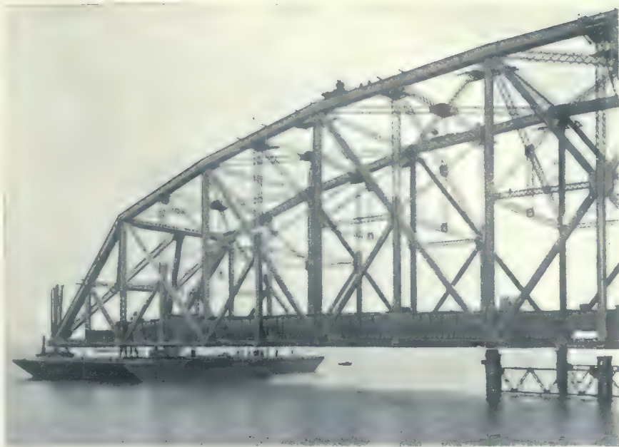
OUTER END OF CENTRE SPAN, SHOWING PONTOONS BEING PLACED IN POSITION.
