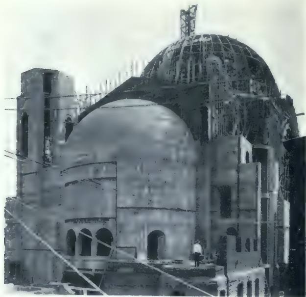
CONCRETE DOME, SHOWING FORMS IN PLACE.
