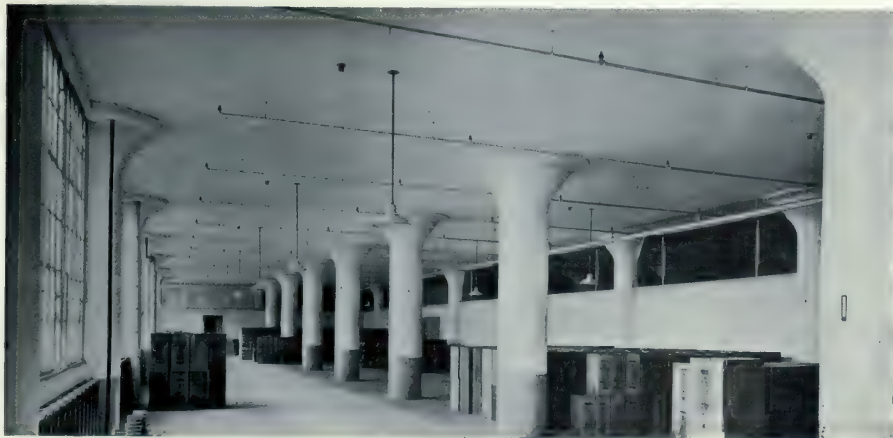
WM. WRIGLEY, JR., FACTORY, INTERIOR VIEW, SHOWING COLUMNS AND FLAT SLAB CONSTRUCTION, ALSO SPRINKLER SYSTEM.
