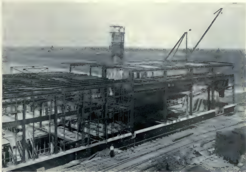
POWER HOUSE UNDER CONSTRUCTION, SHOWING HALF OF OVERHEAD BUNKERS IN BOILER ROOM.
