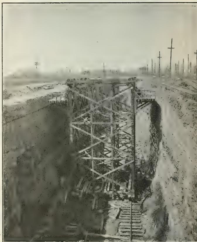
Travelling Derrick in Canal at Sta. 451 + 5, May 6th, 1920
