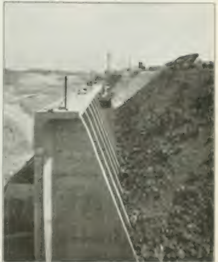
Welland Ship Canal. Lower West Entrance Wall Lock No. 1, in process of backfilling, looking south.
