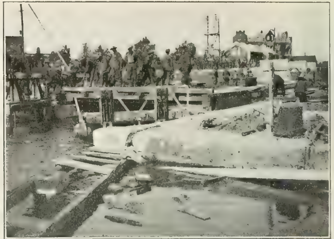
Canadians making emergency repairs to lock-gates in an effort to regain control of water level.
