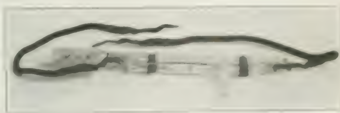
Marconi Coherer. Early Form of Oscillation Detector. 7/8 size.
