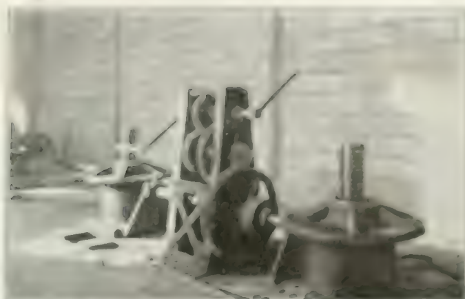
Gate Operating Mechanism
