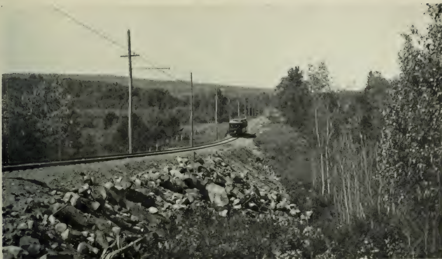
CLIMBING A STEEP GRADE AT FULL SPEED ON A STONE-BALLASTED PRIVATE RIGHT OF WAY
