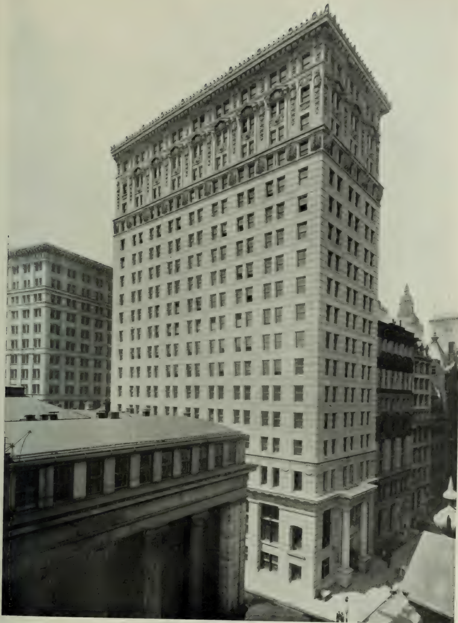
THE OFFICE BUILDING COMPLETED
