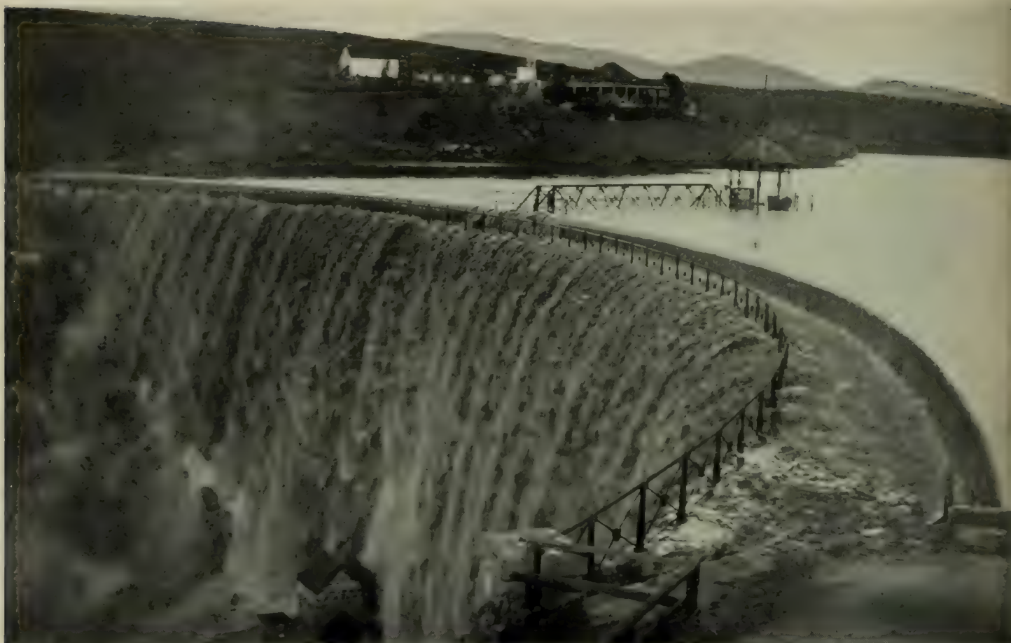
A RESERVOIR OVERFLOWING DURING A HEAVY RAIN, WASTING MILLIONS OF GALLONS OF WATER This reservoir will supply its tributary ranches several years without refilling
