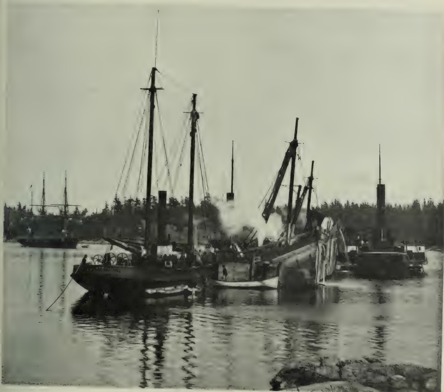
WRECKERS RAISING THE UMATILLA Showing the cofferdam at work
