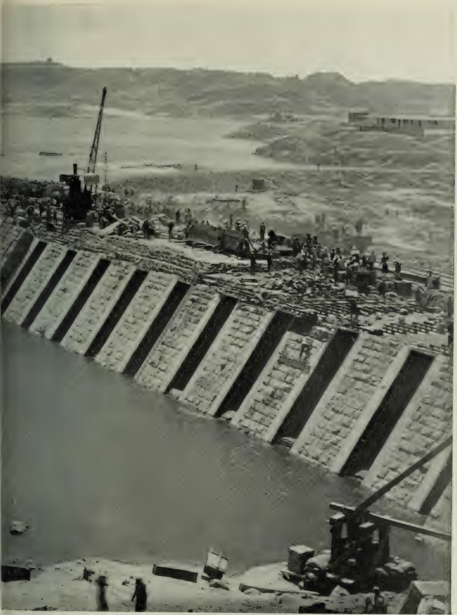
LF COMPLETED gates in the apertures
