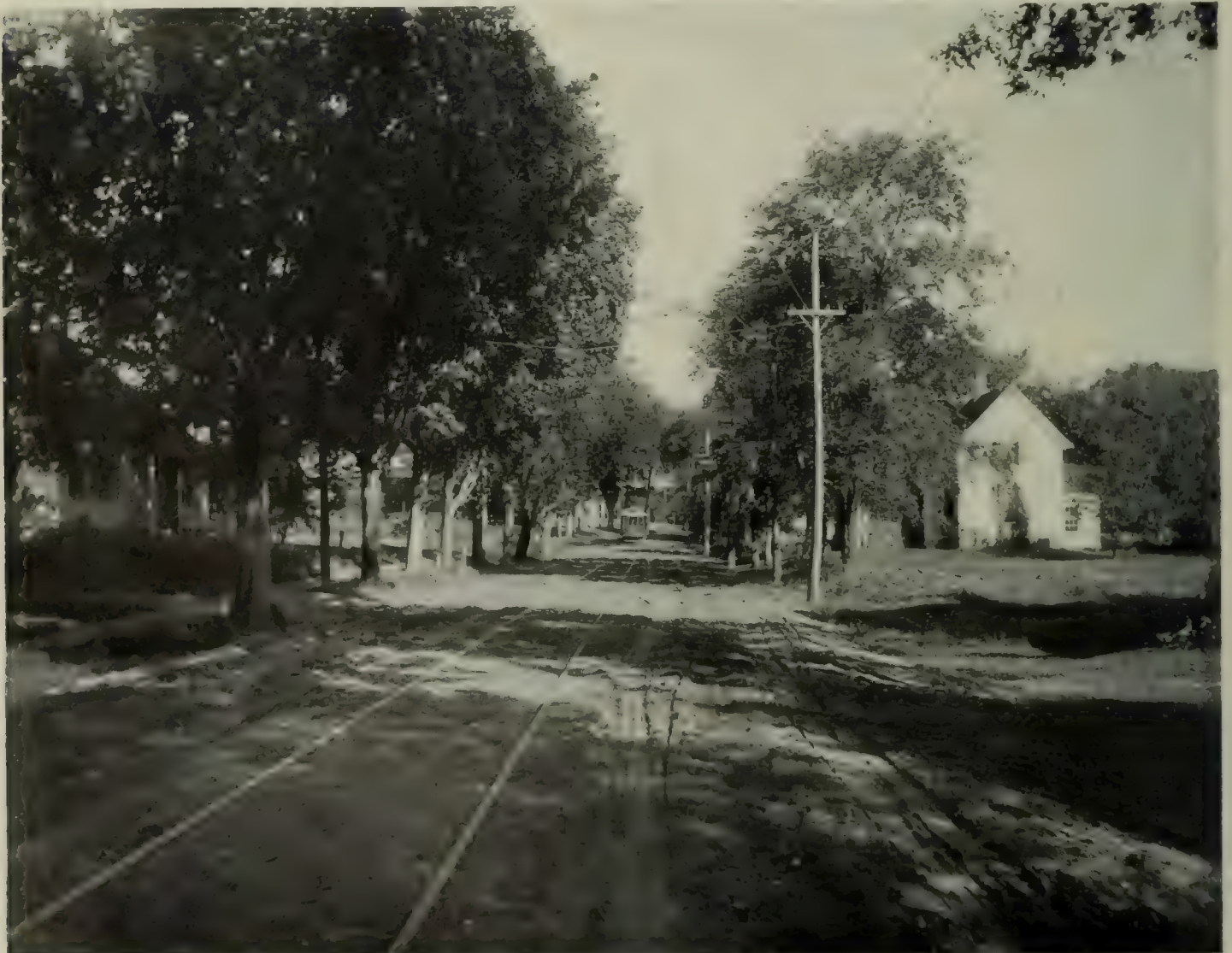
THE TRACK IN GOOD CONDITION IN THE SUBURBS OF CONCORD, NEW HAMPSHIRE
