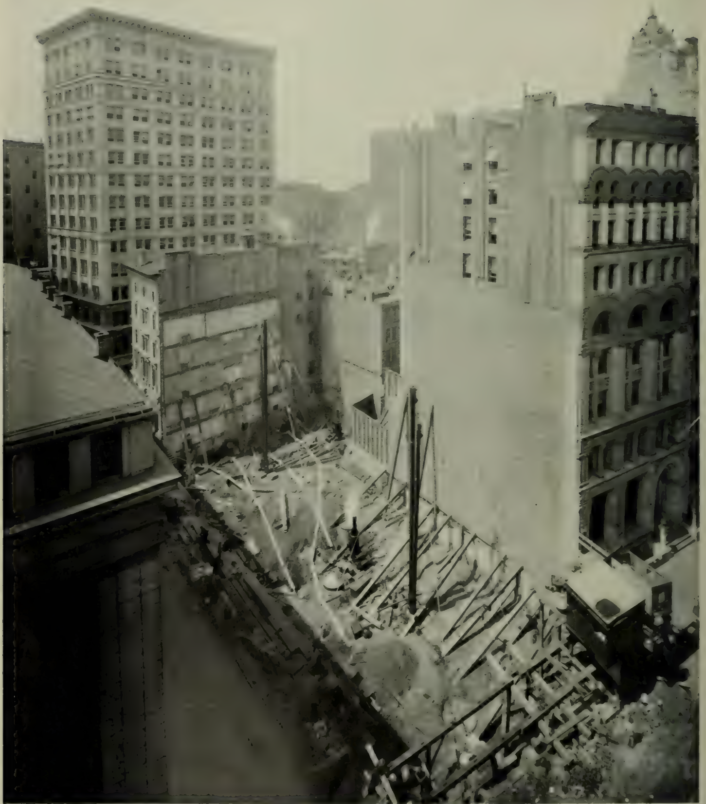
AFTER THE OLD BUILDING HAS BEEN CLEARED AWAY
