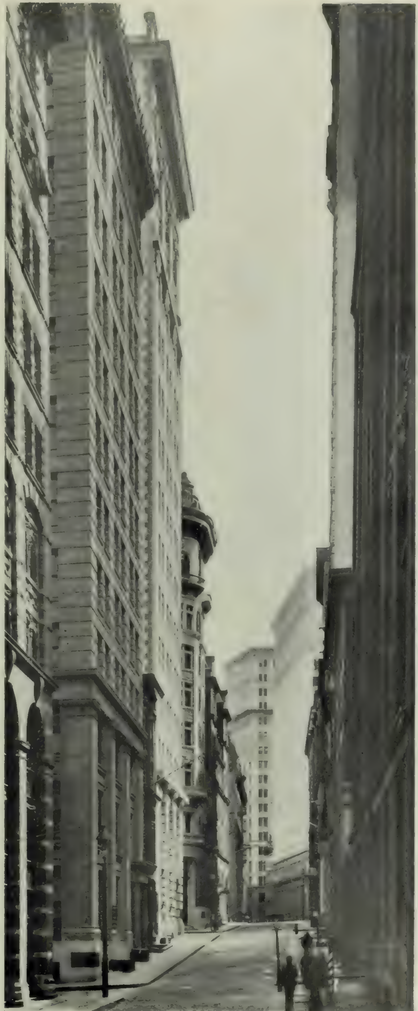
LOOKING DOWN AN OFFICE-BUILDING CANYON TO THE COMPLETED STRUCTURE
