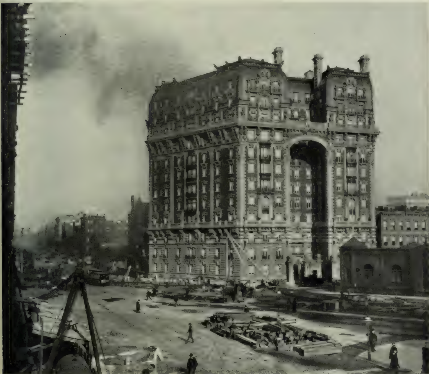
ONE OF THE MOST MODERN OF APARTMENT HOUSES
