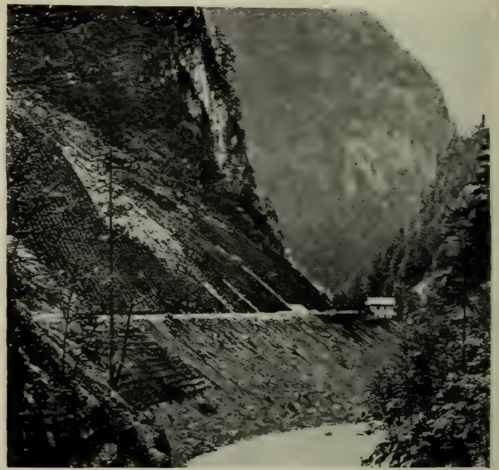
A RAILROAD IN EUROPE, SHOWING WATTLEWORK ON THE EMBANKMENT
