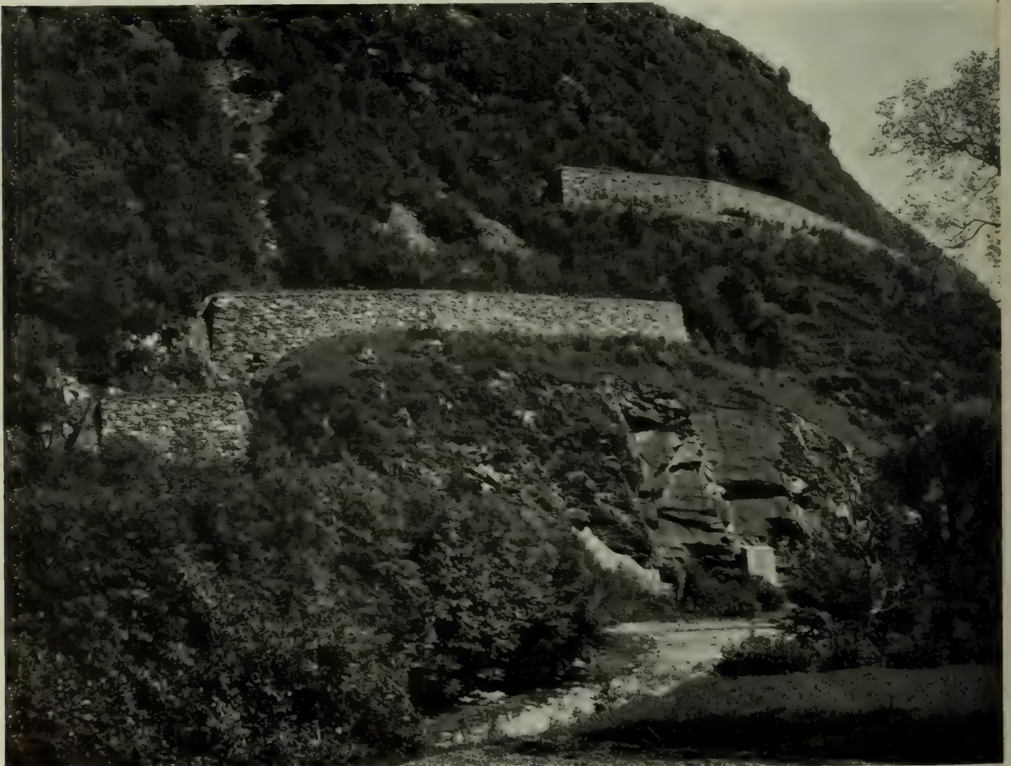
A EUROPEAN HILLSIDE WHERE LANDSLIDES ARE PREVENTED BY BOTH MASONRY AND PINE GROWTH
