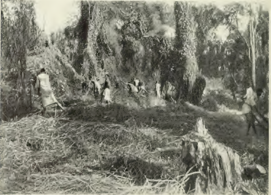
CLEARING THE RAILWAY ROUTE AHEAD OF THE STEEL-WORKERS
