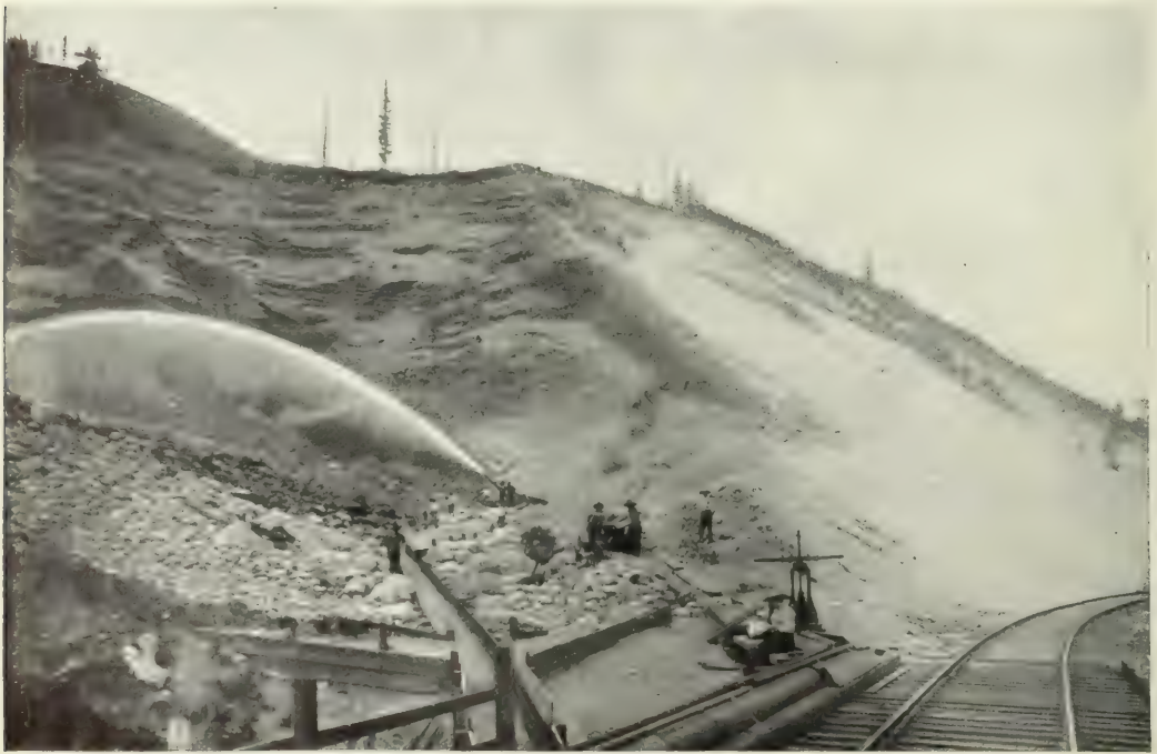
THE MONITOR AT MOUNTAIN CREEK WASHING DOWN GRAVEL FOR THE FILL
