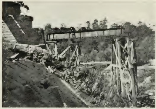
CONSTRUCTION WITH WOODEN FALSE WORK
