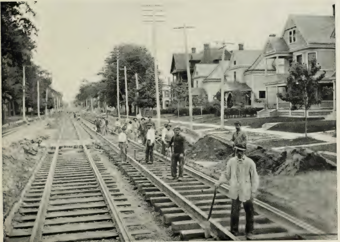
TROLLEY-LINE CONSTRUCTION Showing equipment as heavy as that on steam railroads
