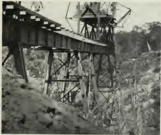
BUILDING STEEL TOWERS 112-FEET HIGH
