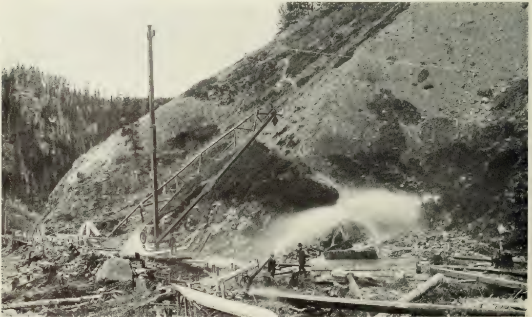
THE NEW METHOD—MINING WITH HYDRAULIC POWER
