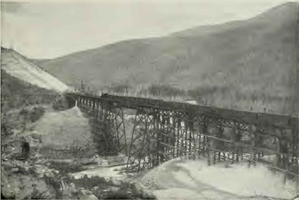
THE COMPLETED WORK AT MOUNTAIN CREEK
