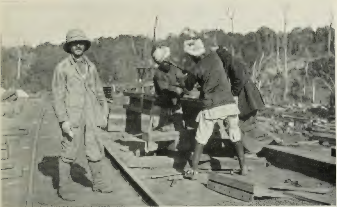
A COOLIE RIVETING GANG AND AN AMERICAN "BOSS"
