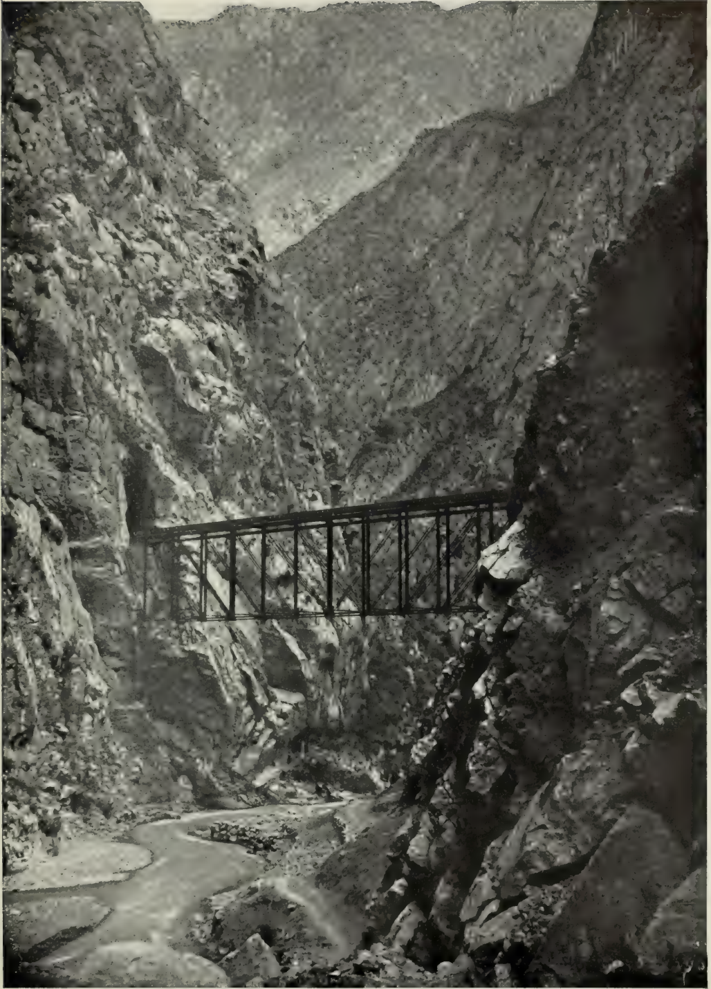
THE 575-FOOT BRIDGE CONNECTING TUNNELS 31 AND 32 ON THE OROYA RAILROAD
