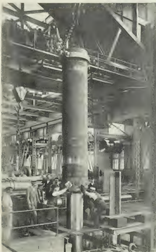
SHRINKING ON A 13-INCH JACKET
