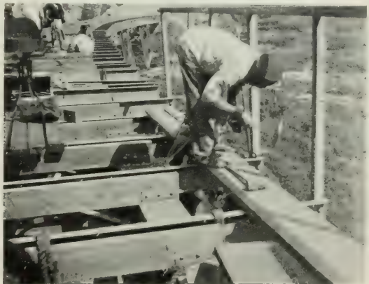
LAYING THE SOUTHERN PINE FLOORING
