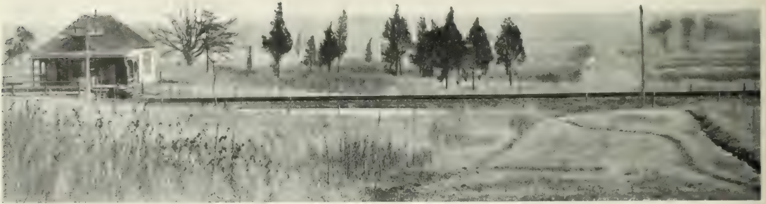
THE SITE OF A BUILT-TO-ORDER TOWN IN NOVEMBER
