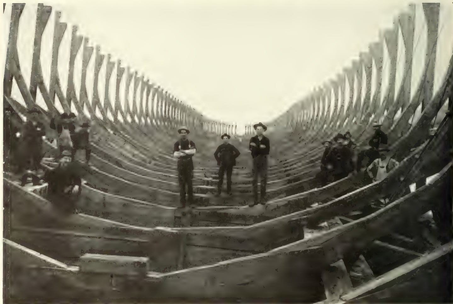
THE EMPTY "CRADLE" FOR BUILDING A GREAT RAFT—ON THE COLUMBIA RIVER, NEAR ASTORIA
