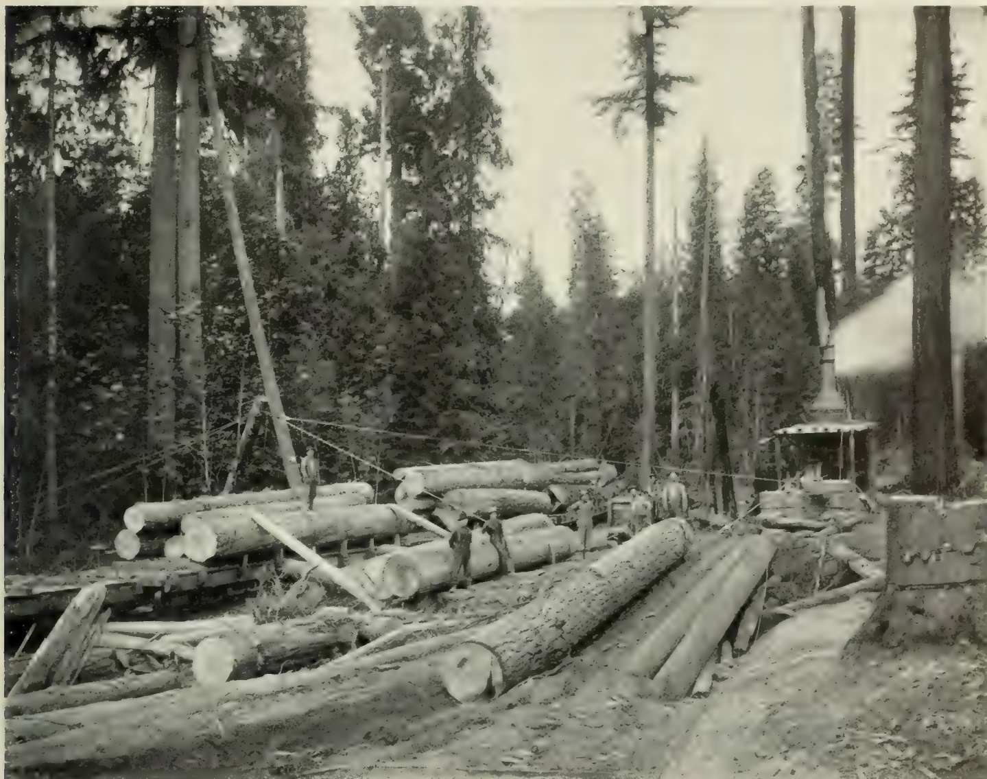
A DONKEY-ENGINE LOADING FLAT CARS AT A LANDING
