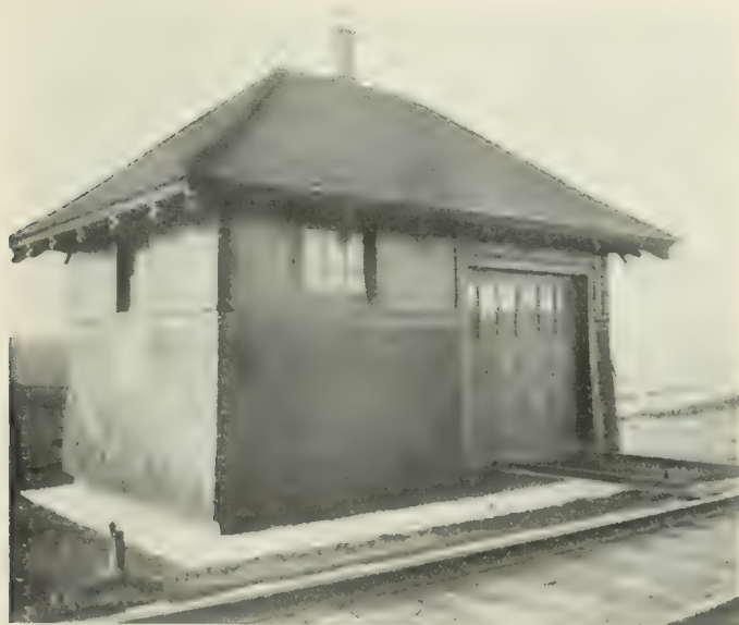
THE ORDINARY TYPE OF THE NEW SECTION-HOUSE
