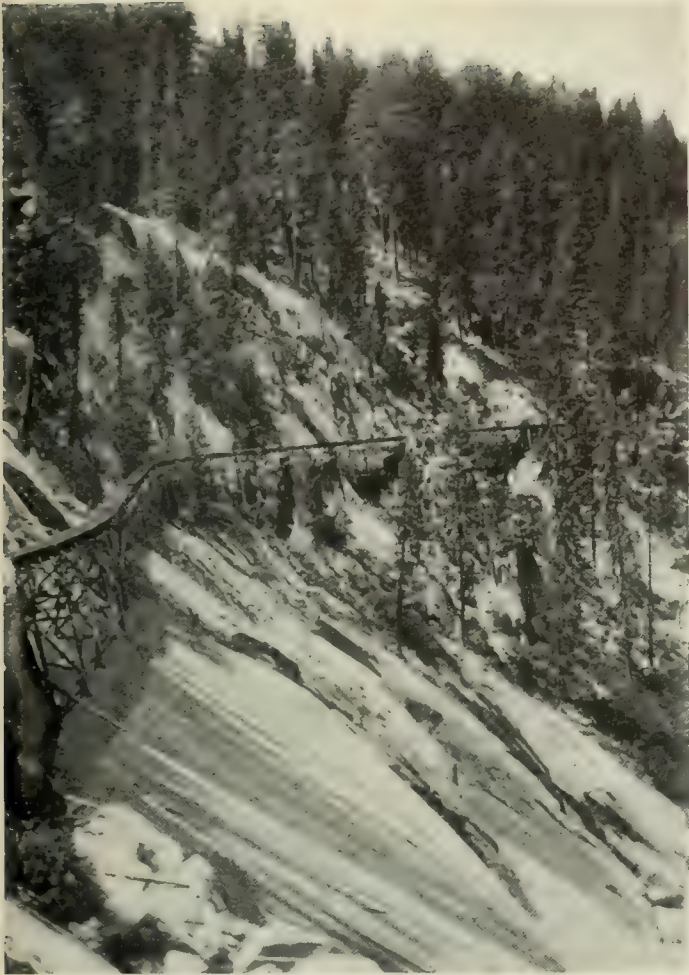
A SIXTY-MILE FLUME THAT CARRIES LOGS FROM THE MILL TO THE RIVER
