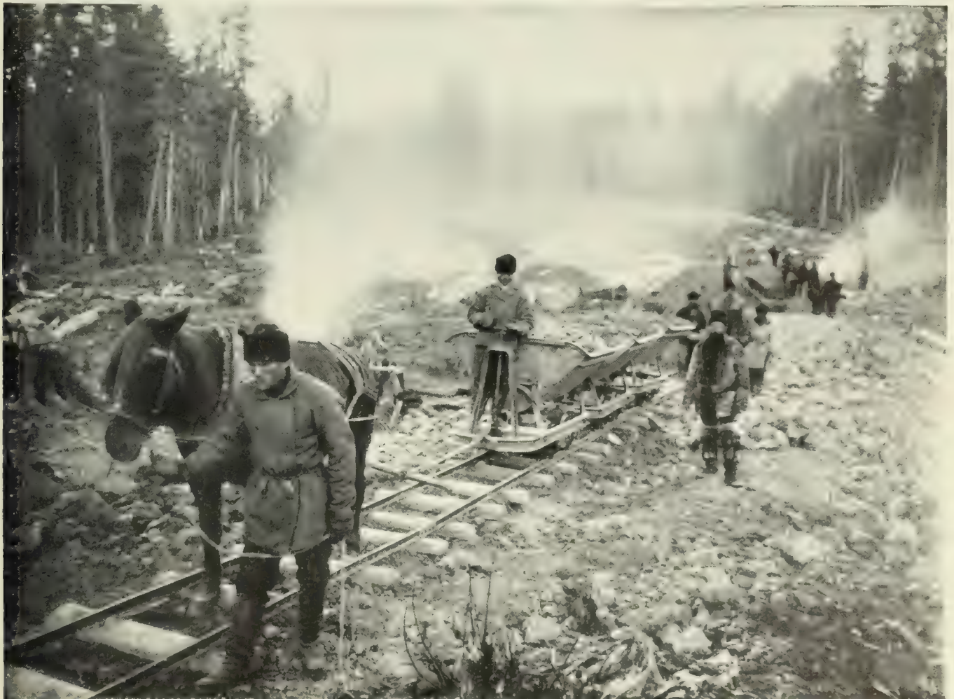
CONVICTS AT WORK ON THE CONSTRUCTION OF THE TRANS-SIBERIAN RAILWAY
