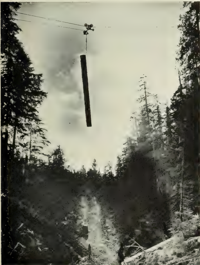
A CABLEWAY THAT CARRIES ENORMOUS LOGS ACROSS A WIDE VALLEY
