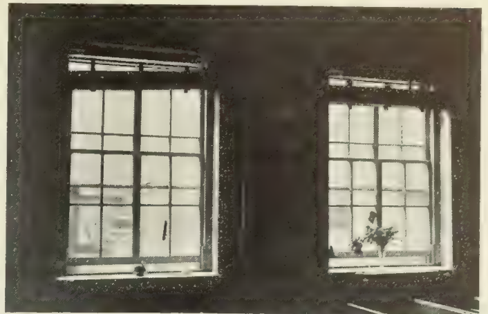
SCHOOL WINDOWS COVERED WITH WIRE NETTING TO PREVENT TENEMENT THIEVES CRAWLING IN
