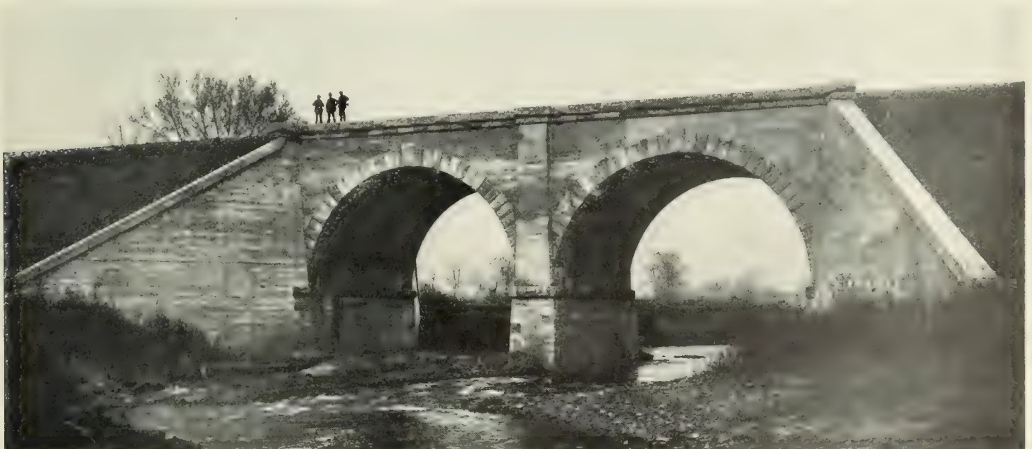
A MODERN CREEK-CROSSING BRIDGE OF THE SAME CLASS AS THE FOREGOING
