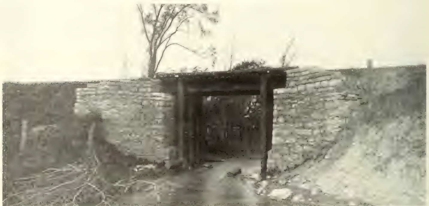
AN OLD CREEK-CROSSING BRIDGE
