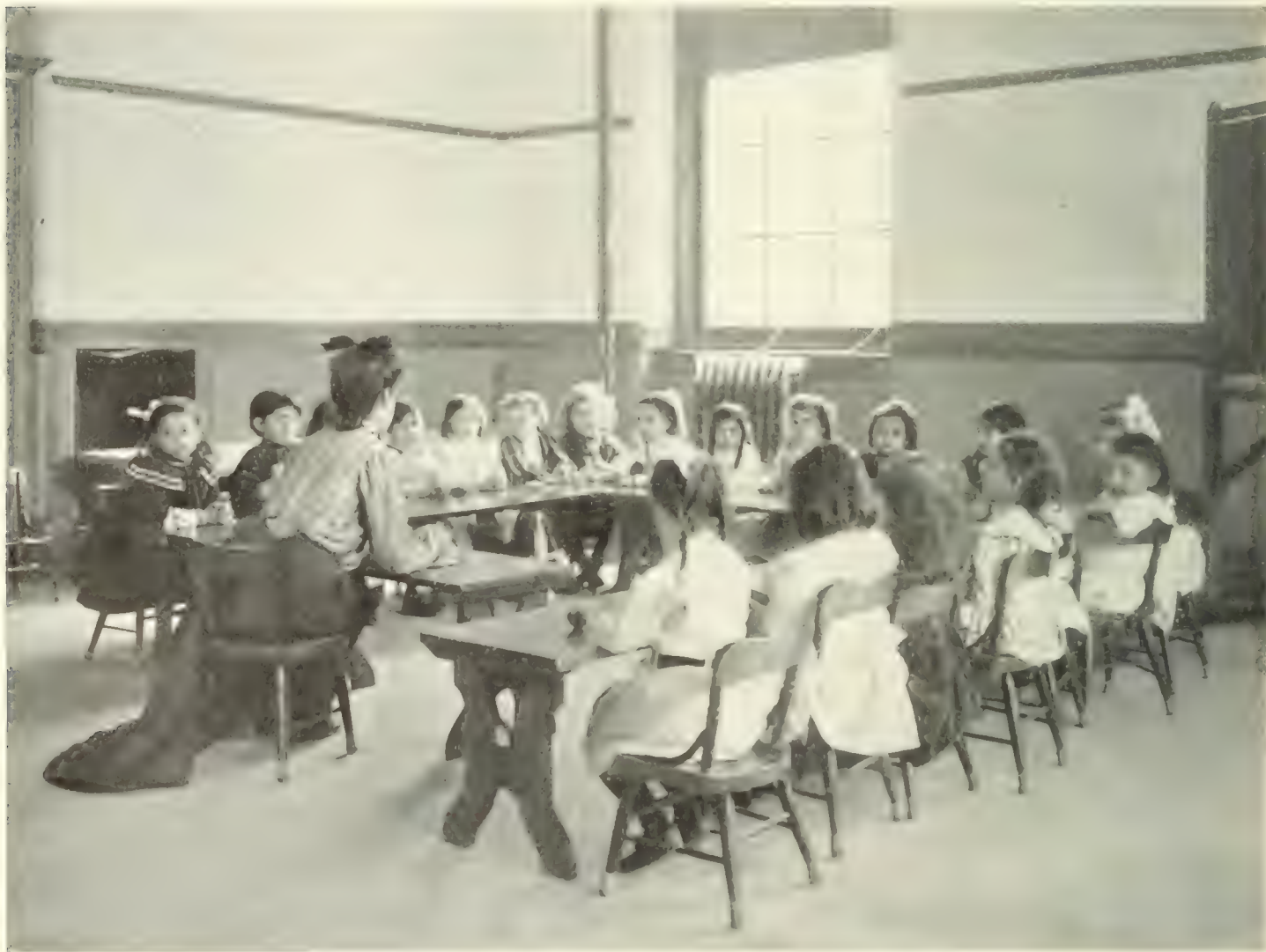
A KINDERGARTEN IN ONE OF THE NEW PARTLY FINISHED SCHOOLS
