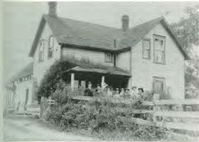
The Adachi Family Home at 10065 McGrath Road.
