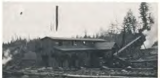
Below: The McNair Shingle Mill.
