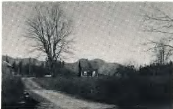
The house that withstood the flood of 1894.
