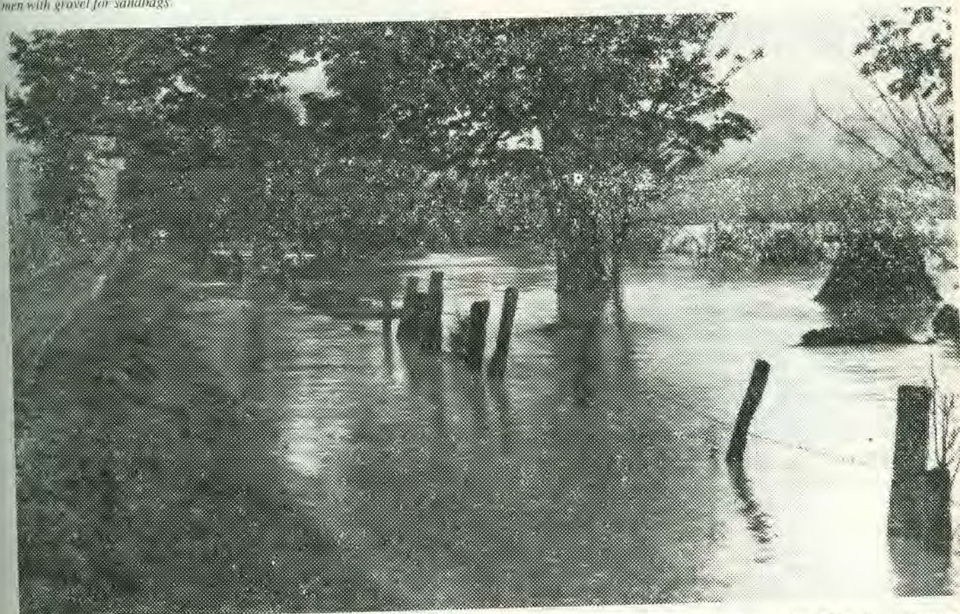
Water alongside the Rosedale dyke. All farm lands outside dyke have been flooded but dykes like these, reinforced by sandbags, kept all but the seepage water out of the fields.
