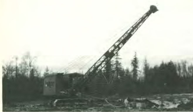
Dragline at Popkum Lake. (Cheam Marl Products).
