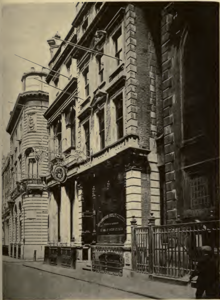
OFFICE OF THE BANK OF BRITISH COLUMBIA, LOMBARD STREET, LONDON
