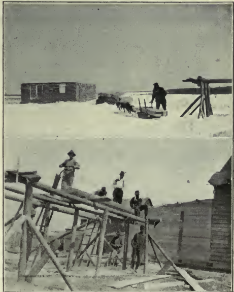
At Fort Hope, Ontario. Upper view: Hauling lumber by dogsleigh for addition to old H.B.C. store. Lower view: Whip sawyers and sawpit working on construction.
